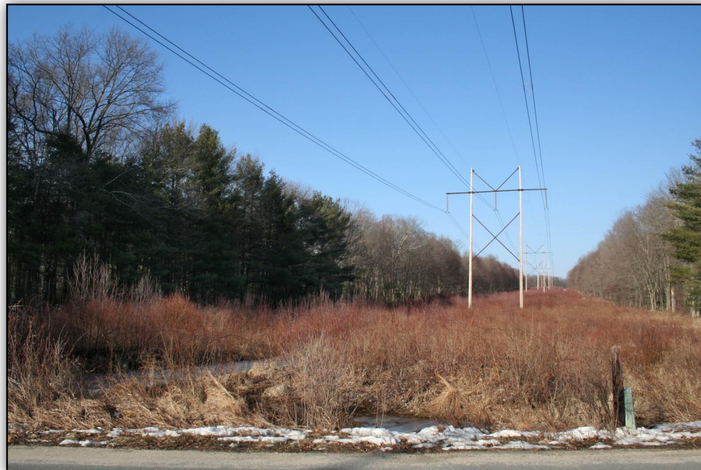
(Existing View – Leaf-off Condition)
