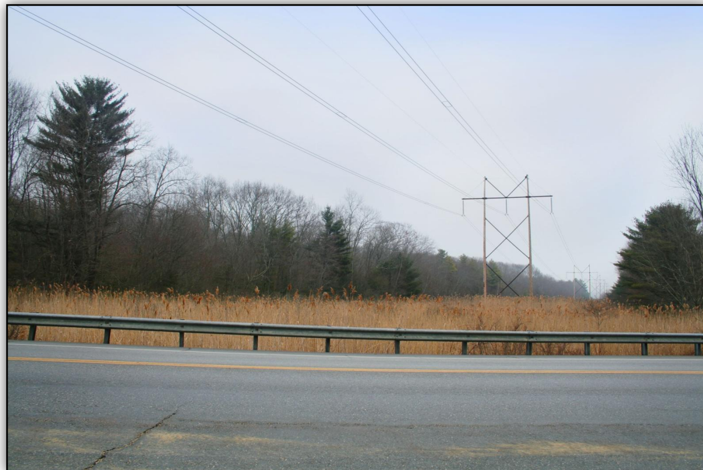
(Existing View – Leaf-off Condition)
