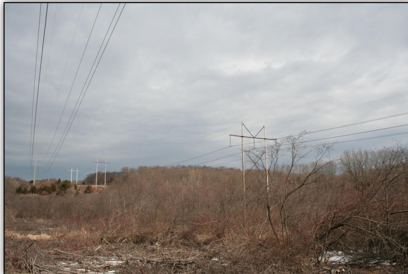
(Existing View – Leaf-off Condition)
