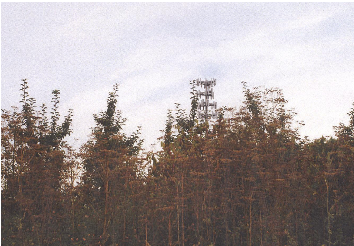
Figure 12: Photo simulation of 160-foot ATC replacement tower (top) and 150-foot Cellco tower (bottom) from 80 West Quasset Road. (Cellco 1, Tab 9; Cellco 10)
