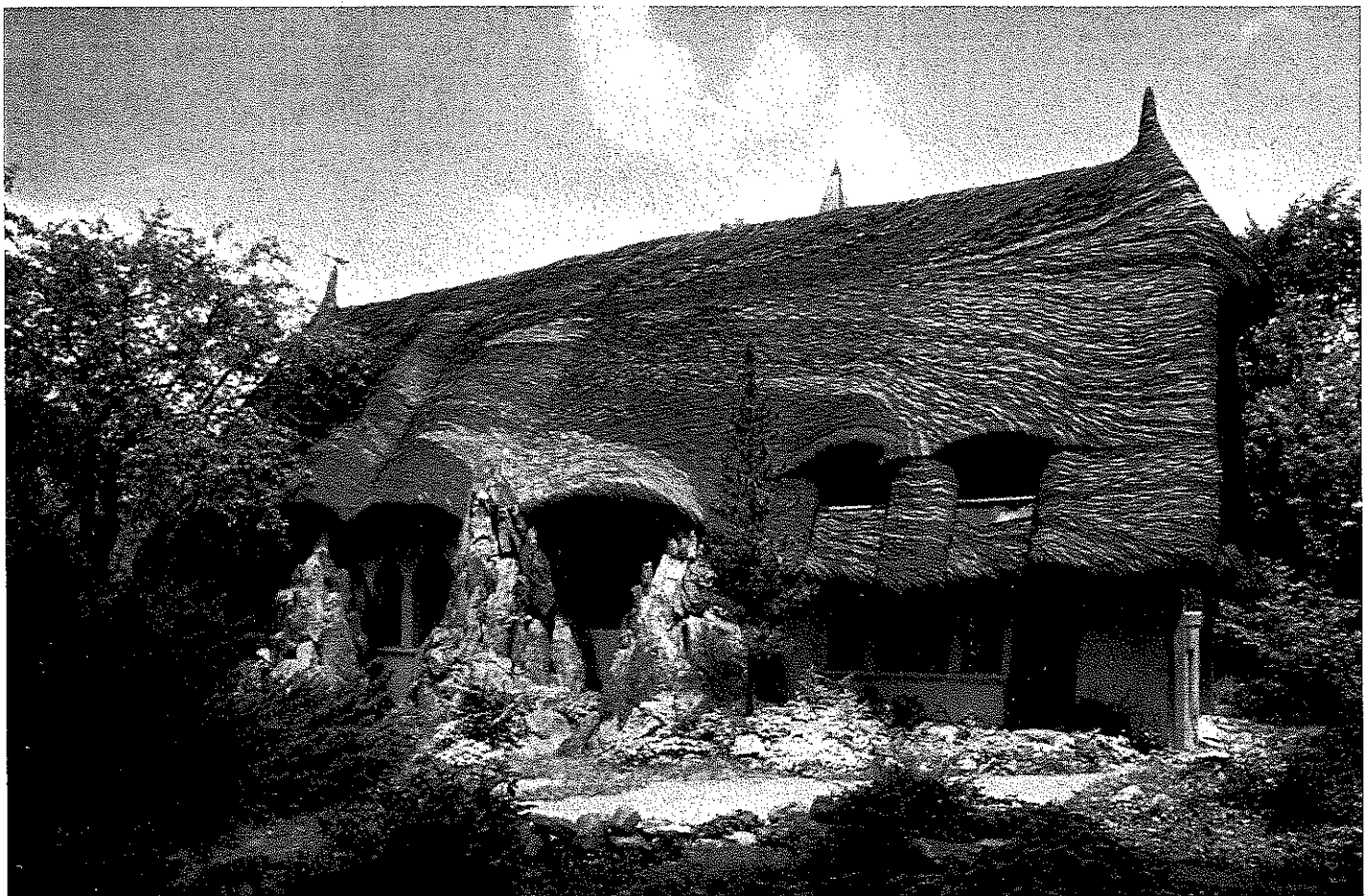
Sculptor Henry Hudson Kitson used Santarella, in Tyringham, MA, as his studio in the 1930s & 40s. The wooden shingle roof is designed to resemble a thatched cottage.
