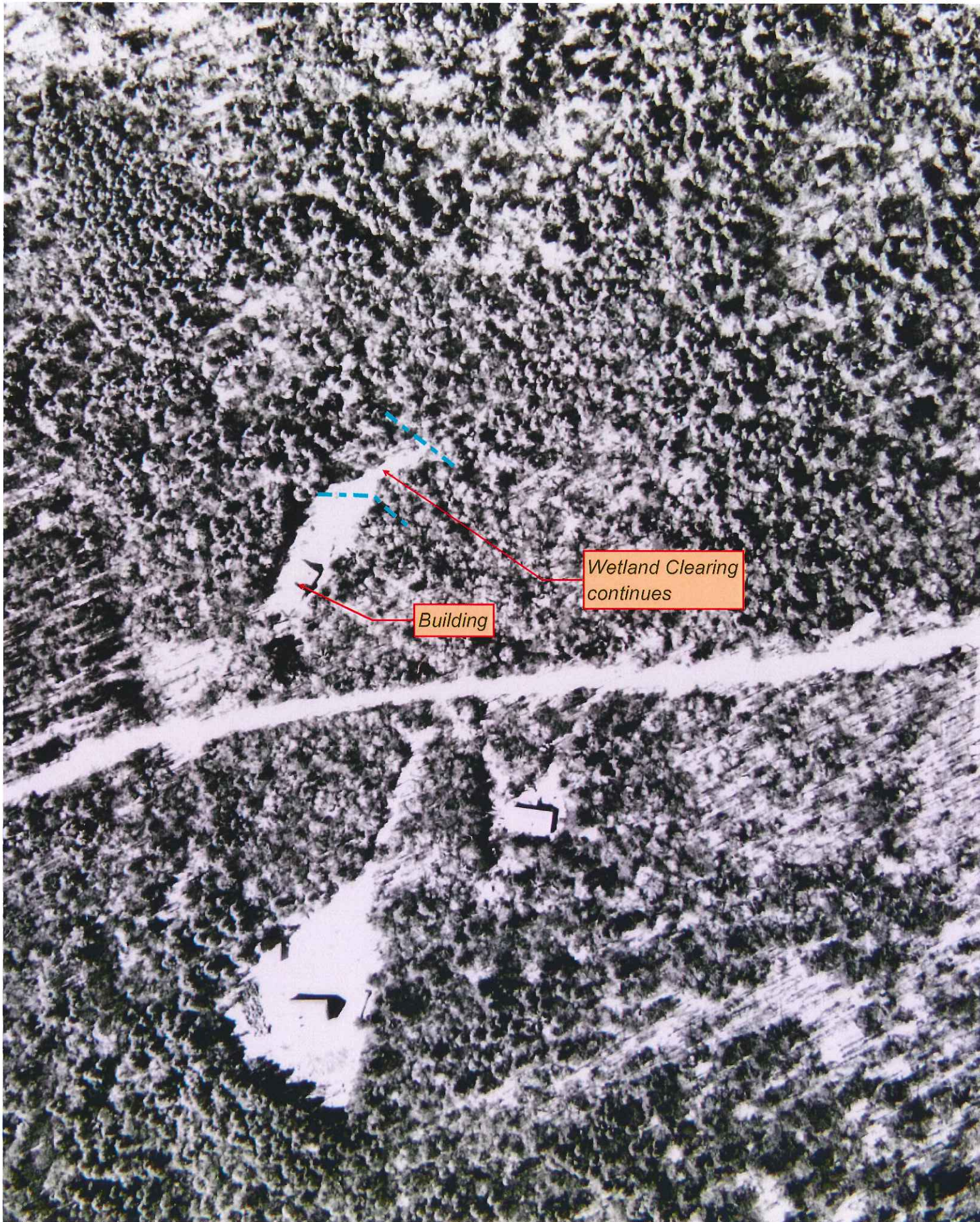
Figure 5: 1990 CT DEP Aerial Photograph of 95 Balance Rock Road, East Hartland, CT
