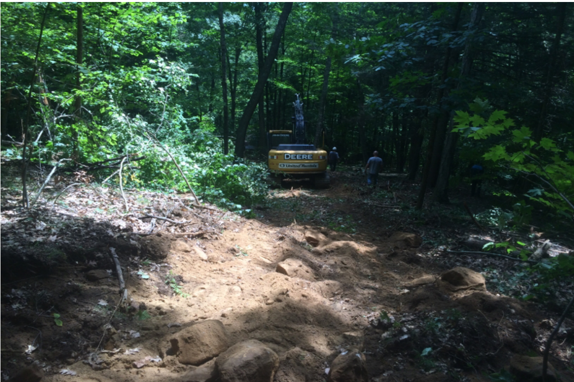
Photo 4: View of proposed access road under construction looking Southeast.
