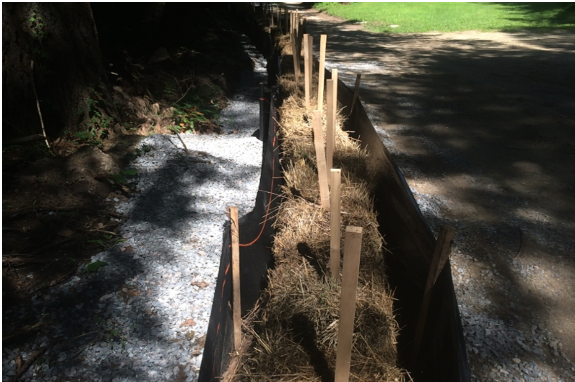
Photo 2: Close up view of partially installed E&S controls.
