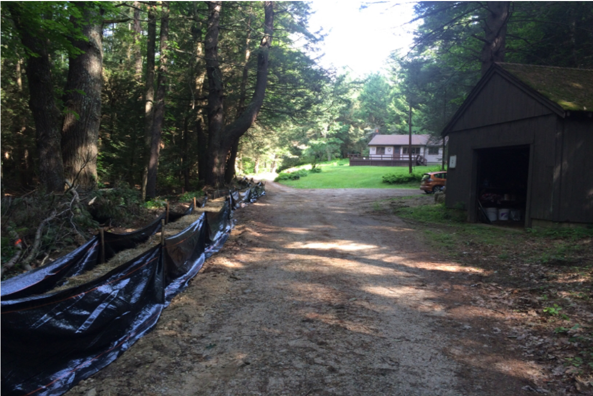
Photo 3: Overview of access road looking northwest.
