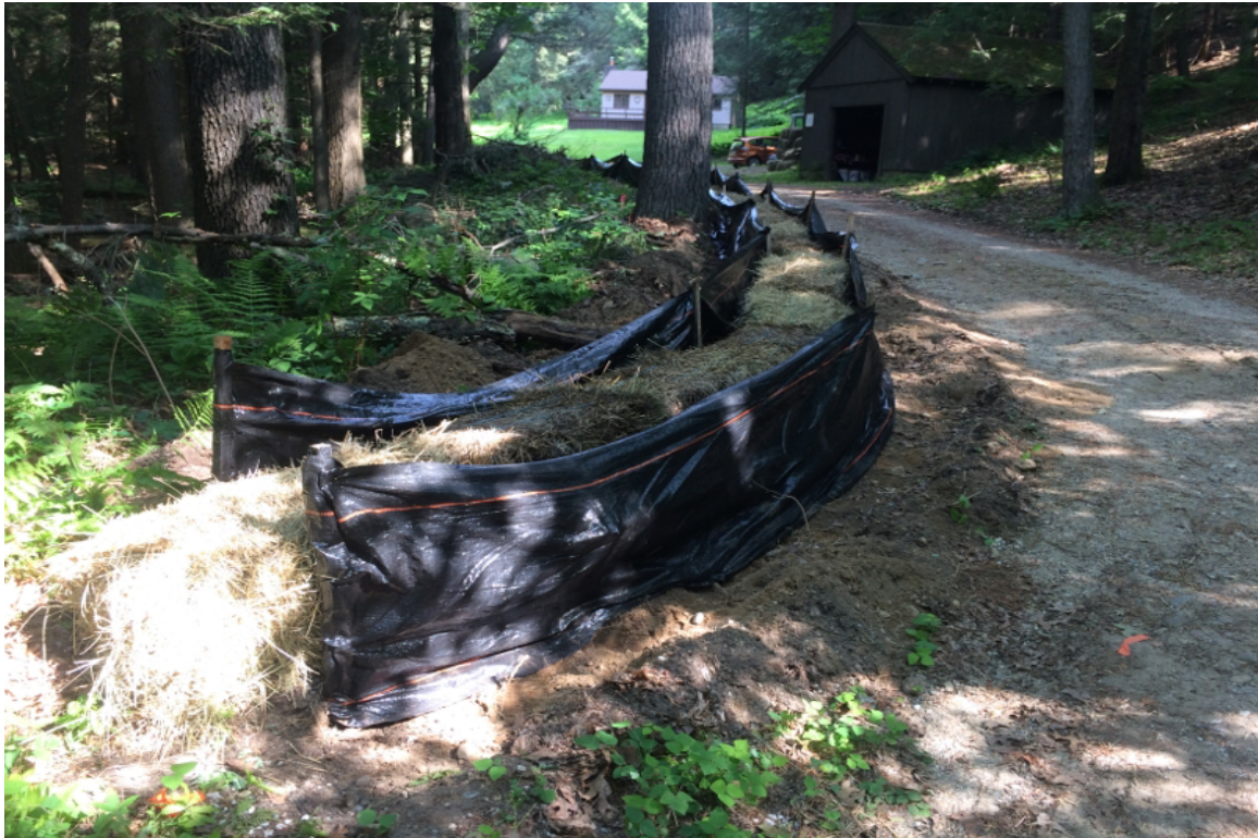
Photo 1: View of start of E&S controls looking northwest.
