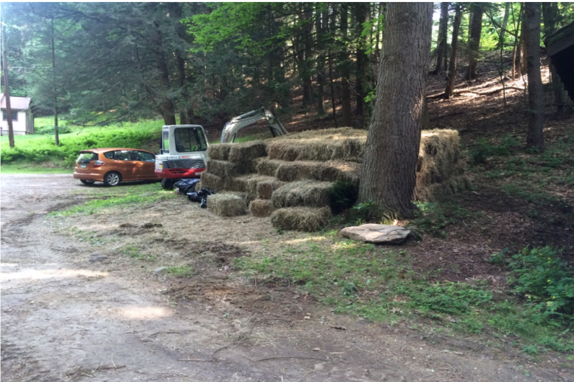
Photo 4: View of stockpiled E&S controls looking north.
