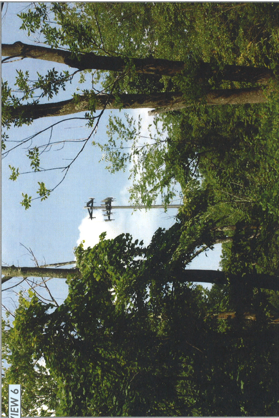
PHOTO TAKEN FROM DAYTON ROAD ADJACENT TO HOUSE# 271, LOOKING WEST DISTANCE FROM THE PHOTOGRAPH LOCATION TO SITE IS 0.06 MILE +/-
