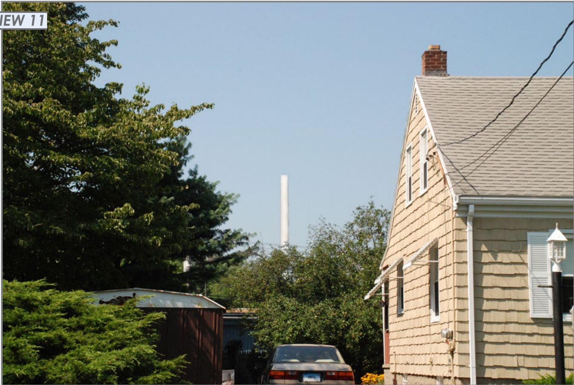
PHOTO TAKEN FROM VIELE STREET SOUTH OF MARCROFT STREET, LOOKING SOUTHWEST DISTANCE FROM THE PHOTOGRAPH LOCATION TO SITE IS 0.11 MILE +/-
