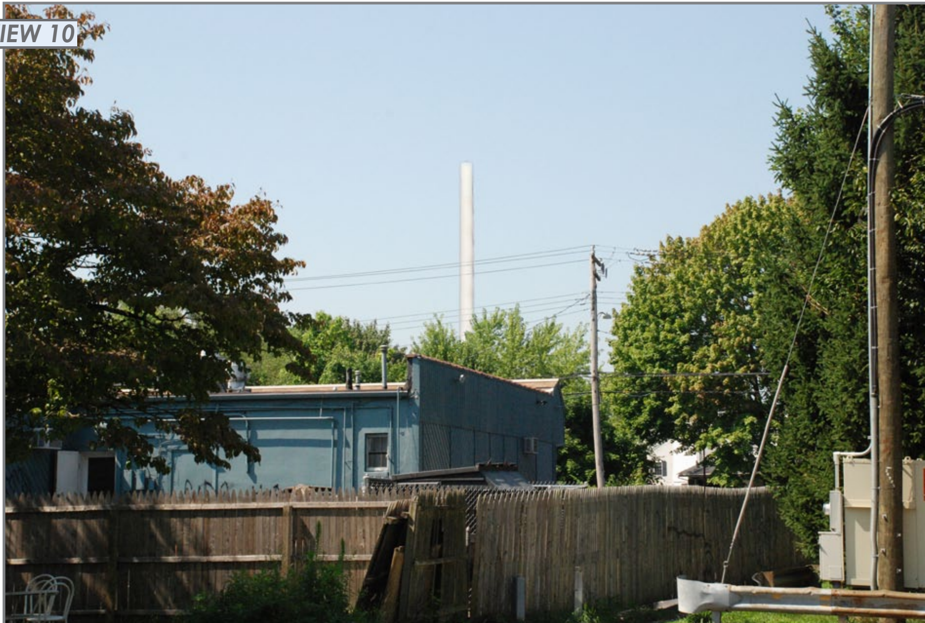
PHOTO TAKEN FROM END OF MARCROFT STREET, LOOKING SOUTHWEST DISTANCE FROM THE PHOTOGRAPH LOCATION TO SITE IS 0.11 MILE +/-
