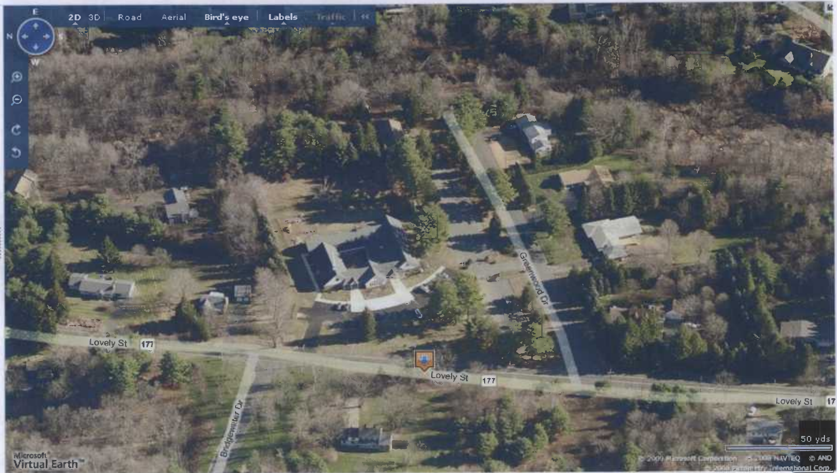
Aerial Photo of St. Matthew Church - eastern orientation
