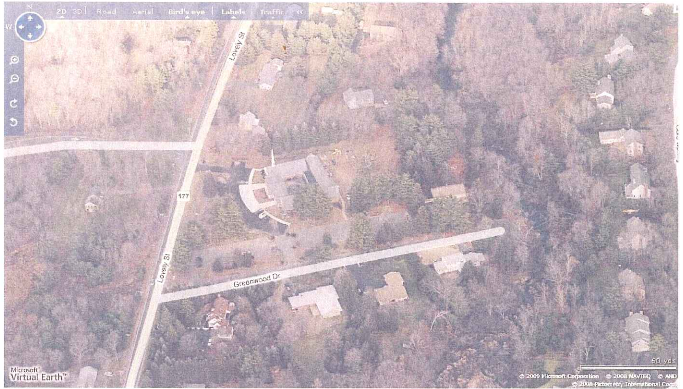
Figure 2: Aerial view of 224 Lovely Street, Avon. (AT&T 3, Tab A)
