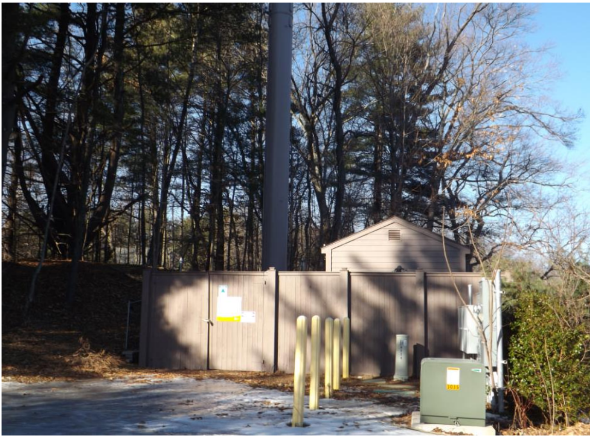
Tower compound area, January 2015.
