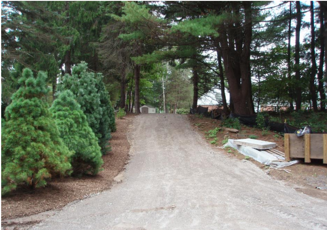
Access road near end of construction. Note evergreen landscaping. September 2011.
