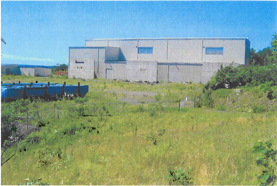
Existing Power House and GSU Platforms
