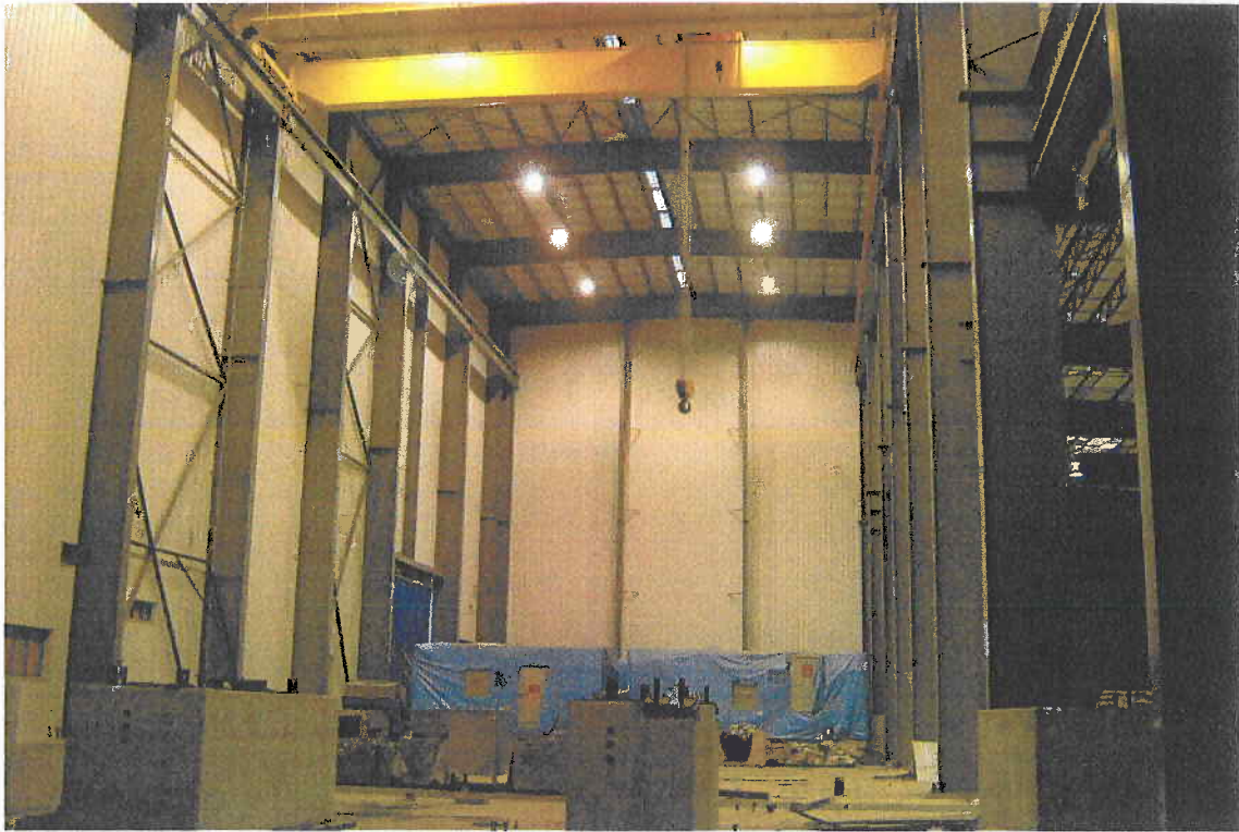
Power House Interior
