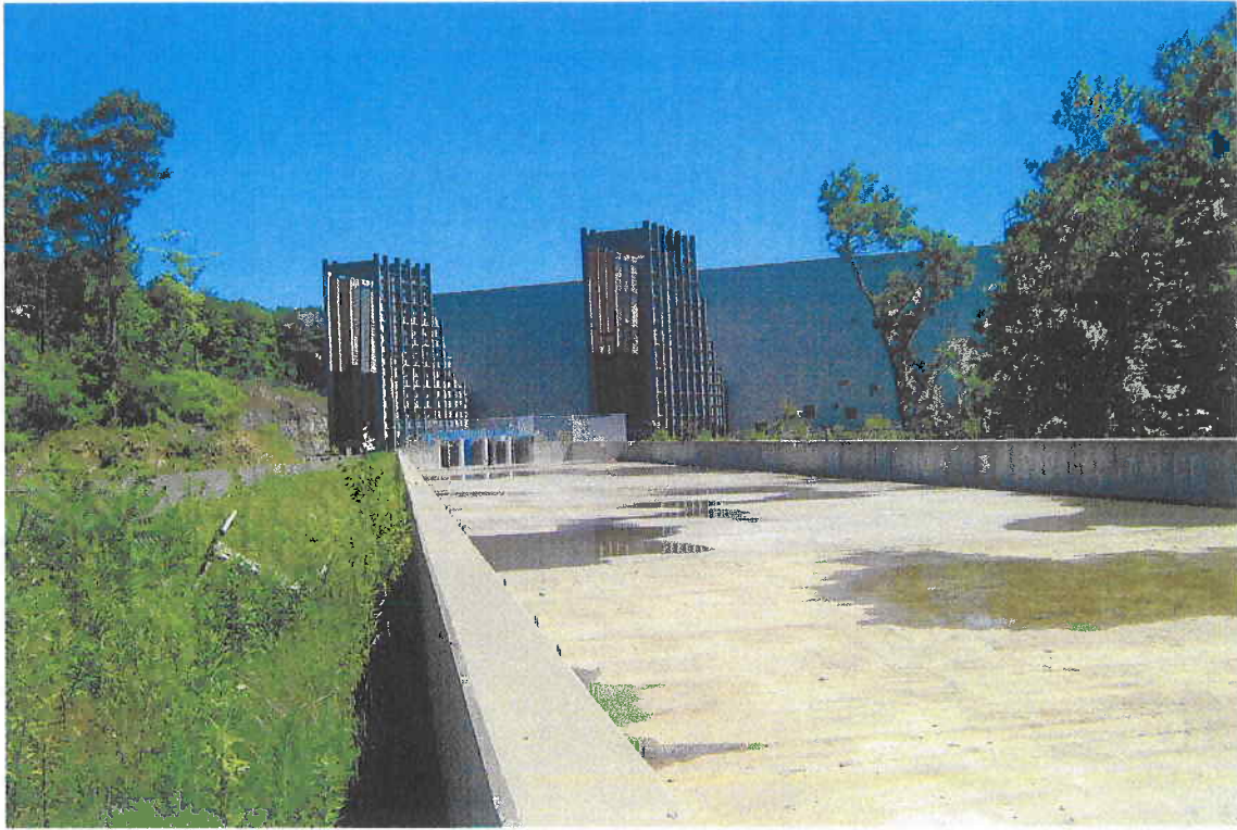
Existing Cooling Tower Basis Looking Towards HRSGs
