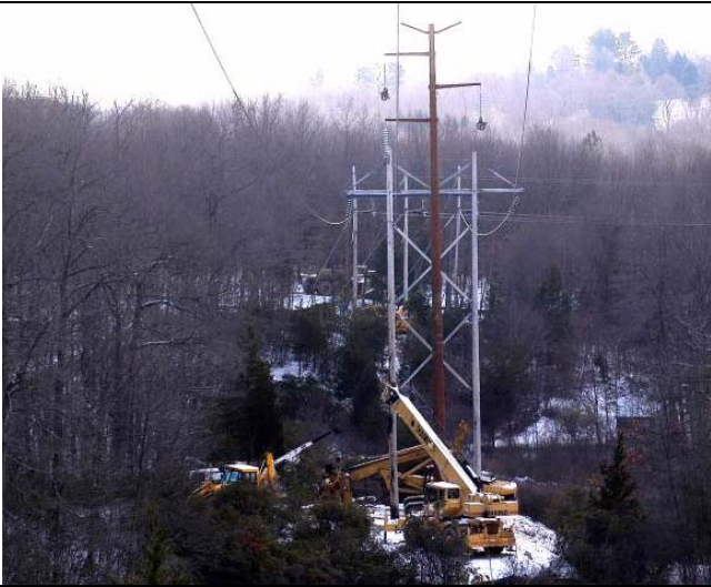
Installation of overhead pole structures
