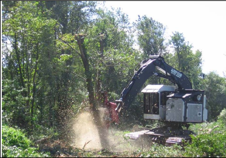
Vegetation clearing within existing right-of-way.
