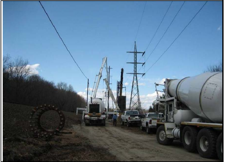
Installation of pole structures
