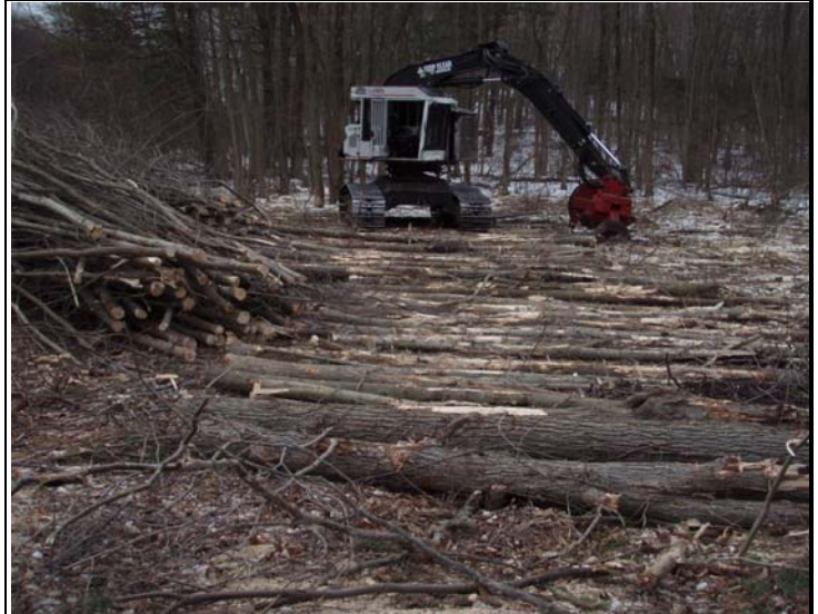
Cleared vegetation being used for wetland matting.
