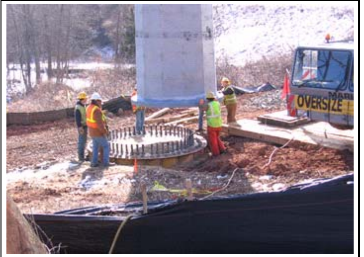
Installing pole structure on foundation.
