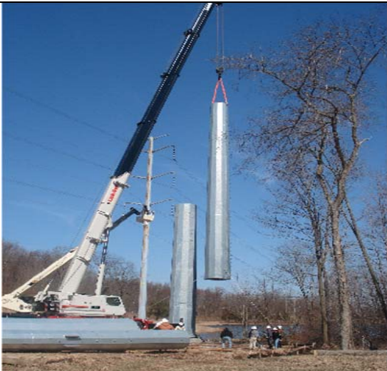
Assembly of pole structure.
