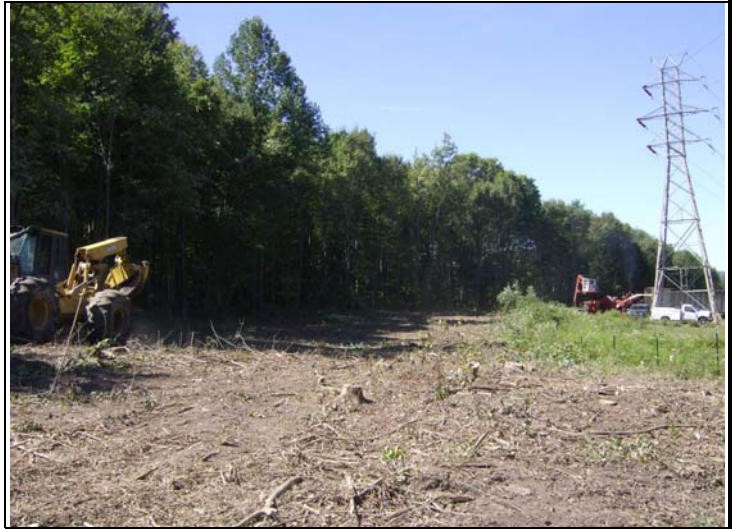
Vegetation clearing within existing right-of-way.
