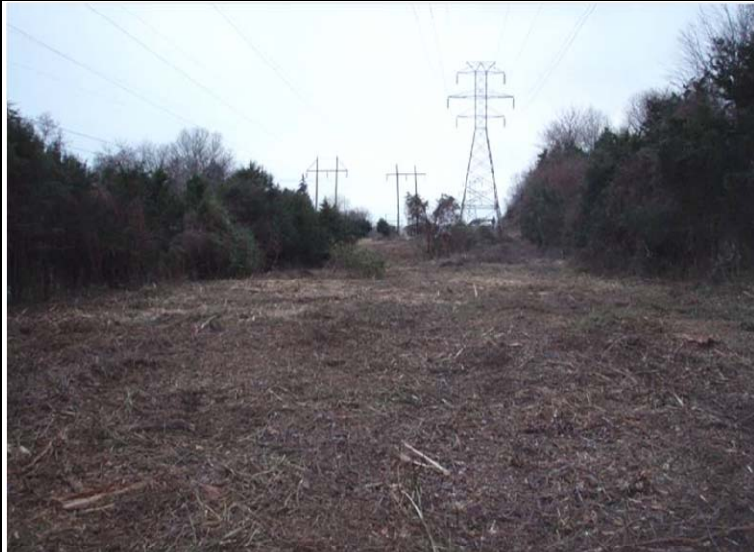
Vegetation clearing within existing right-of-way.
