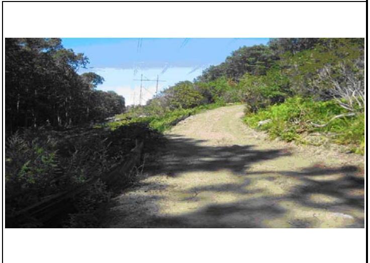
Construction equipment access road.
