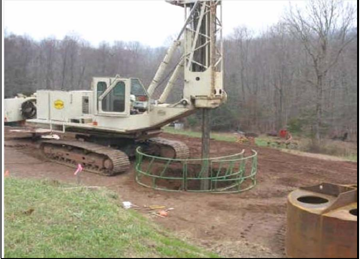
Boring foundation for pole structure.
