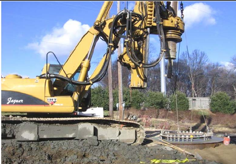
Installation of bolts for pole structure.
