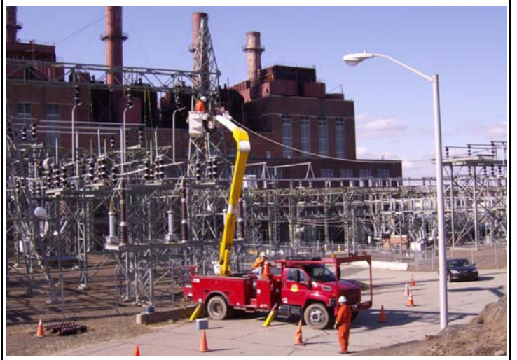
Construction activity at substation.
