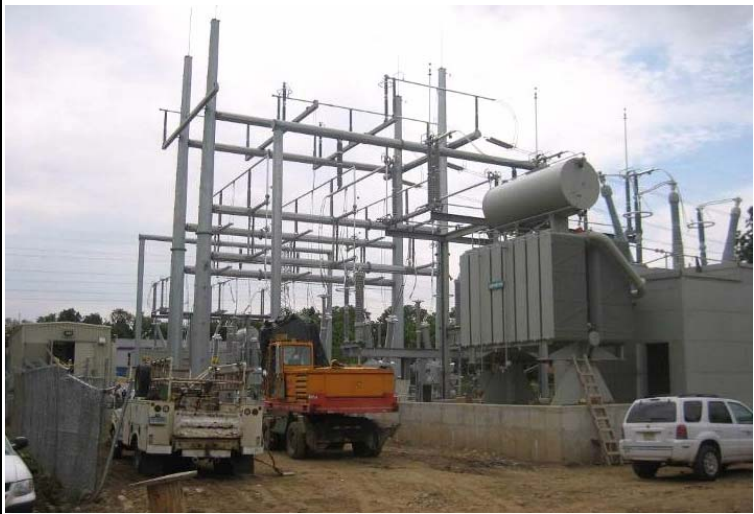
Construction activity at substation.
