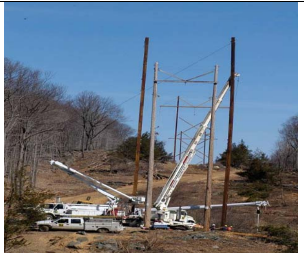
New H-framed being installed.
