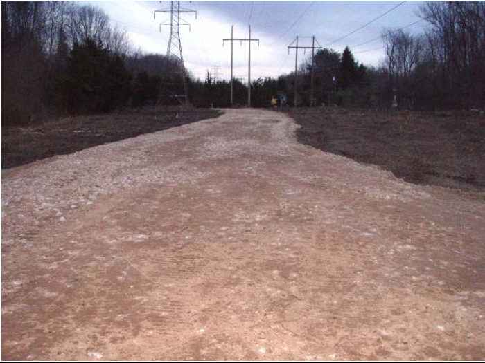
Construction equipment access road.
