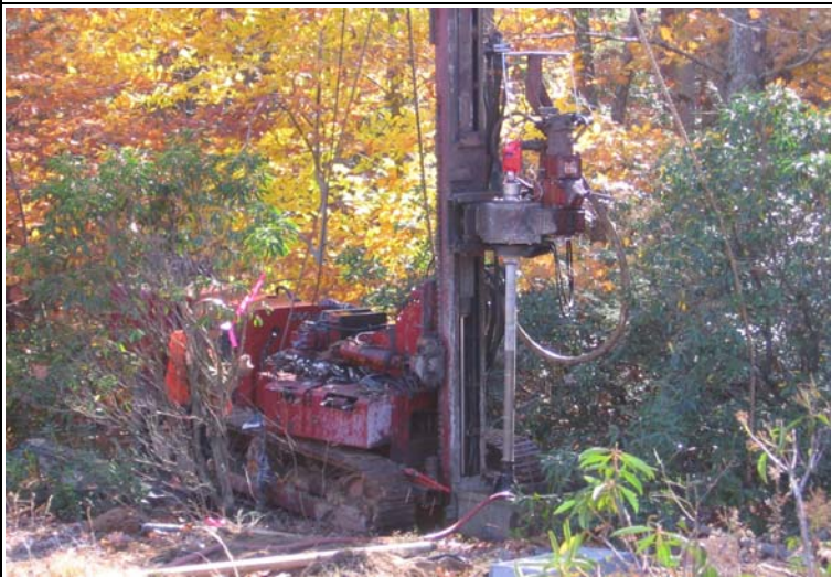
Test bore for soil conditions.
