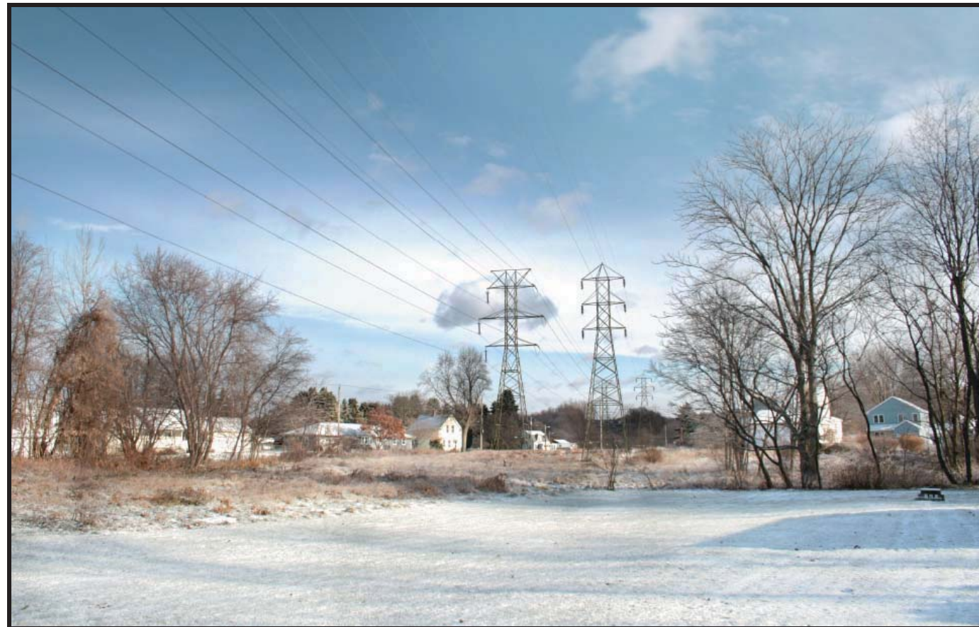
Existing electric transmission line structures looking east from Wayfield Avenue, northeast of Piper Substation
