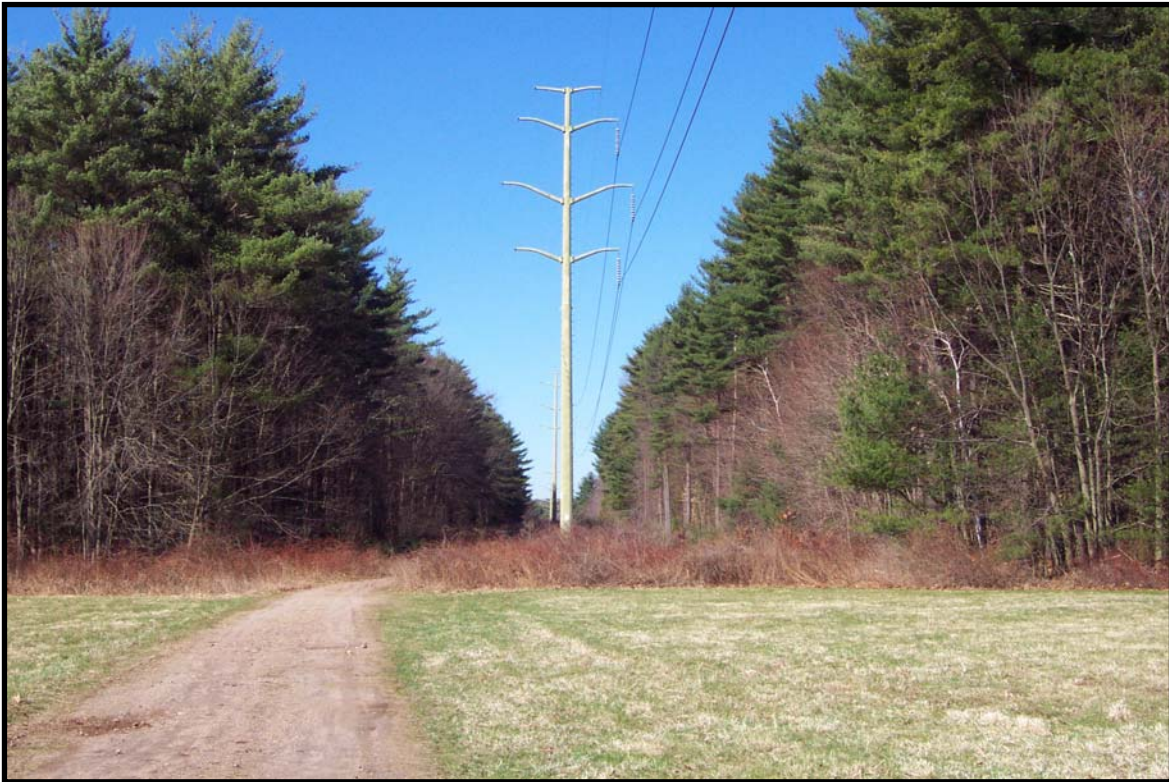
Photo 345-kV Line Route OH-21: View west from Prospect Street in the Town of East Longmeadow, MA.
