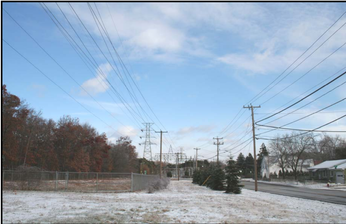
Photo 345-kV Line Route OH-12: View northeast from Ponds Street toward Chicopee Substation in the City of Chicopee, MA.
