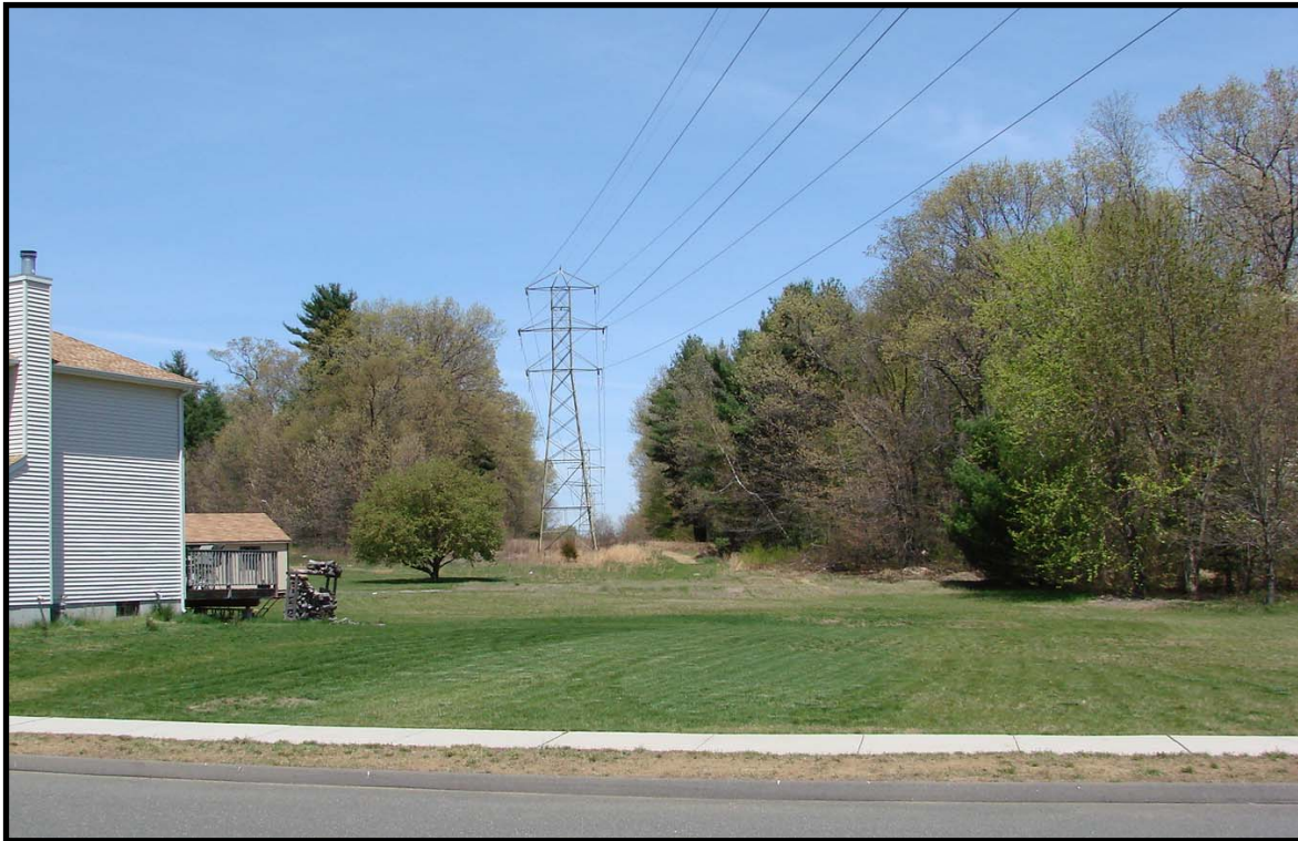
Photo 345-kV Line Route OH-05: View north from Lancaster Drive in the Town of Agawam, MA.
