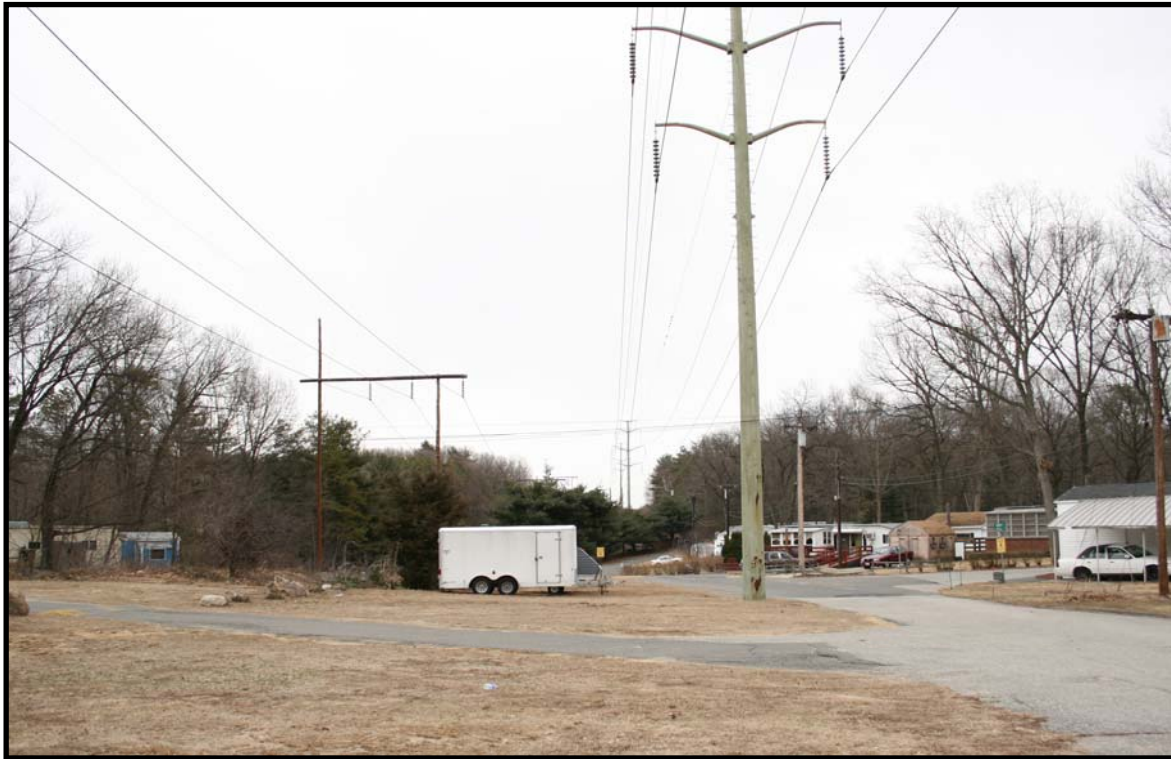
Photo 345-kV Line Route OH-15: View east from Dove Drive and Wren Drive in the City of Chicopee, MA.
