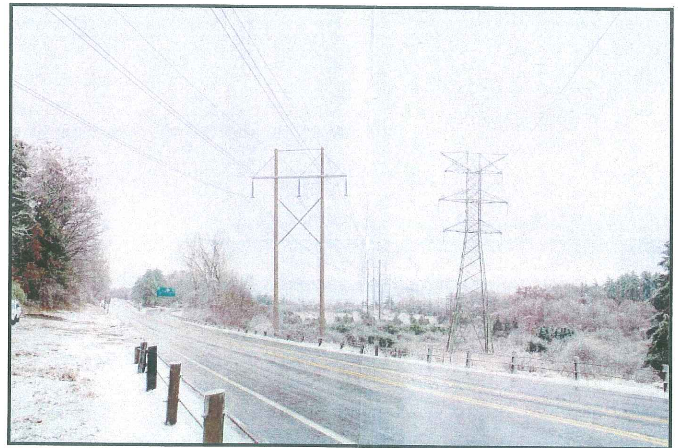
Proposed electric transmission line structures looking southwest from State Highway 189, north of North Bloomfield Substation.
