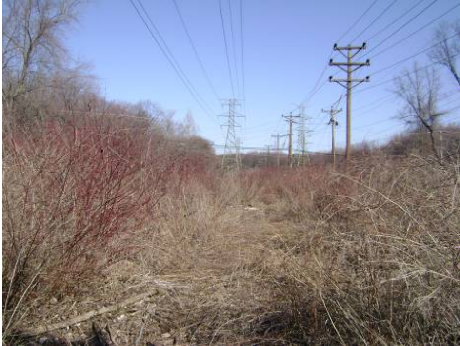
W01HF001, photograph looking north
