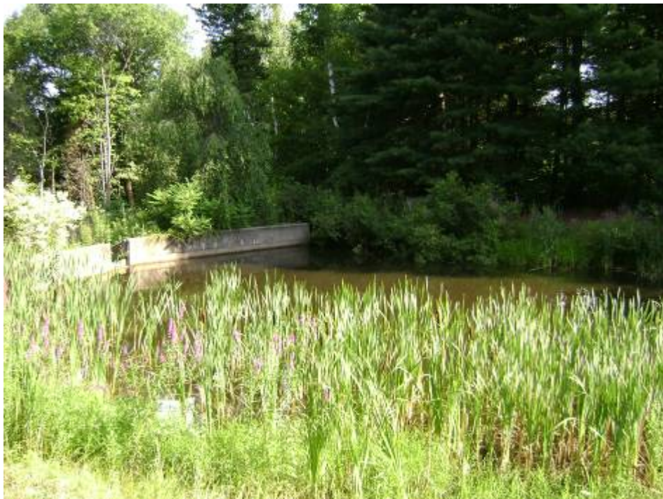
Wetland W01HF013, photograph looking northwest
