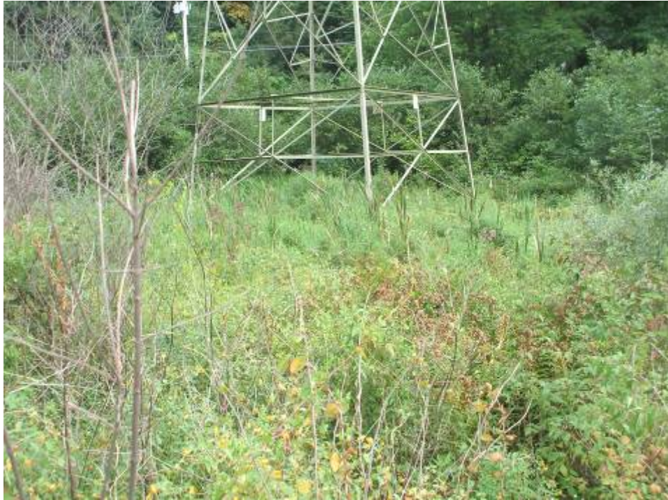
W04HF005, photograph looking northeast
