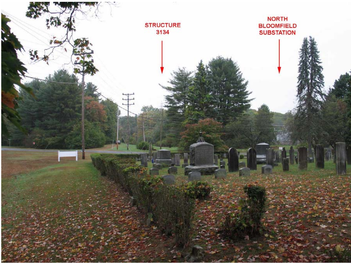
EXISTING VIEW SOUTHEAST TO STRUCTURE 3134
