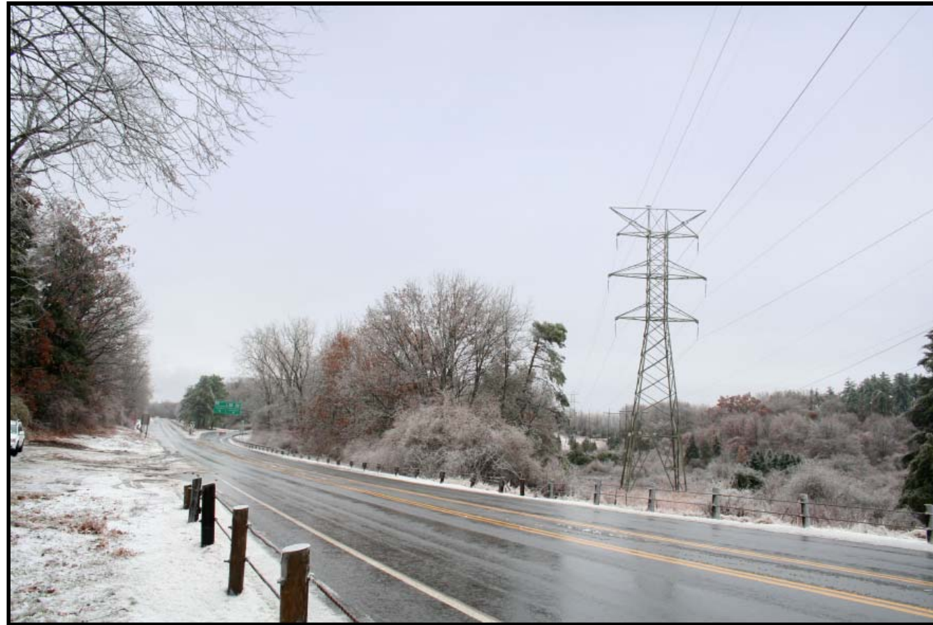
Existing electric transmission line structures looking southwest from State Highway 189, north of North Bloomfield Substation.
