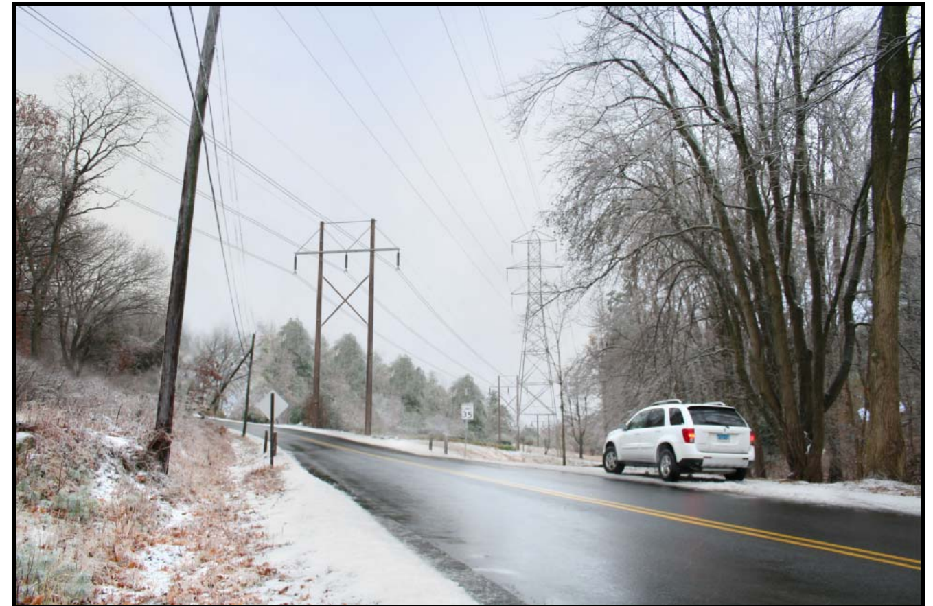
Proposed electric transmission line structures looking south from Newgate Road, northeast of Granby Junction.
