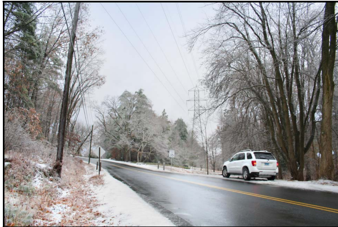
Existing electric transmission line structures looking south from Newgate Road, northeast of Granby Junction.
