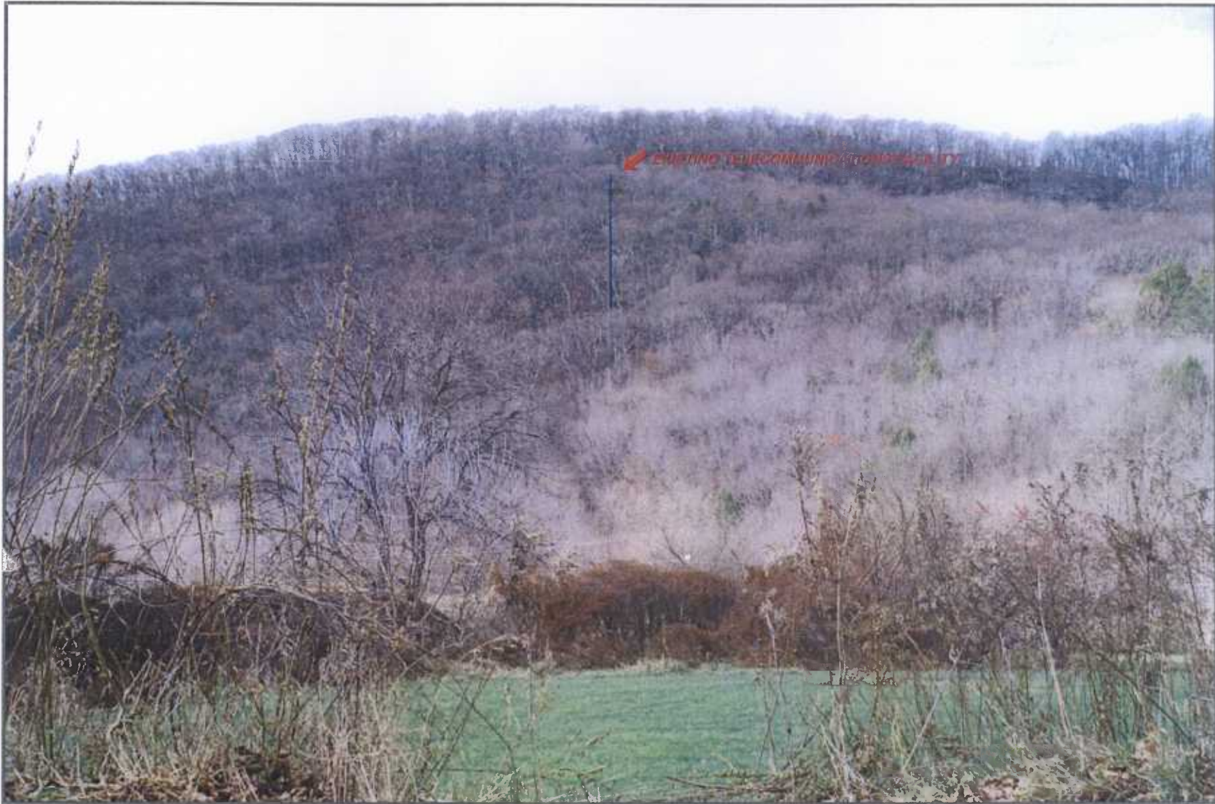
EXISTING 150 - FOOT TALL MONOPOLE WITH FLUSH-MOUNTED ANTENNAS (PHOTOGRAPHED NOVEMBER 2008), WASHINGTON, CT
