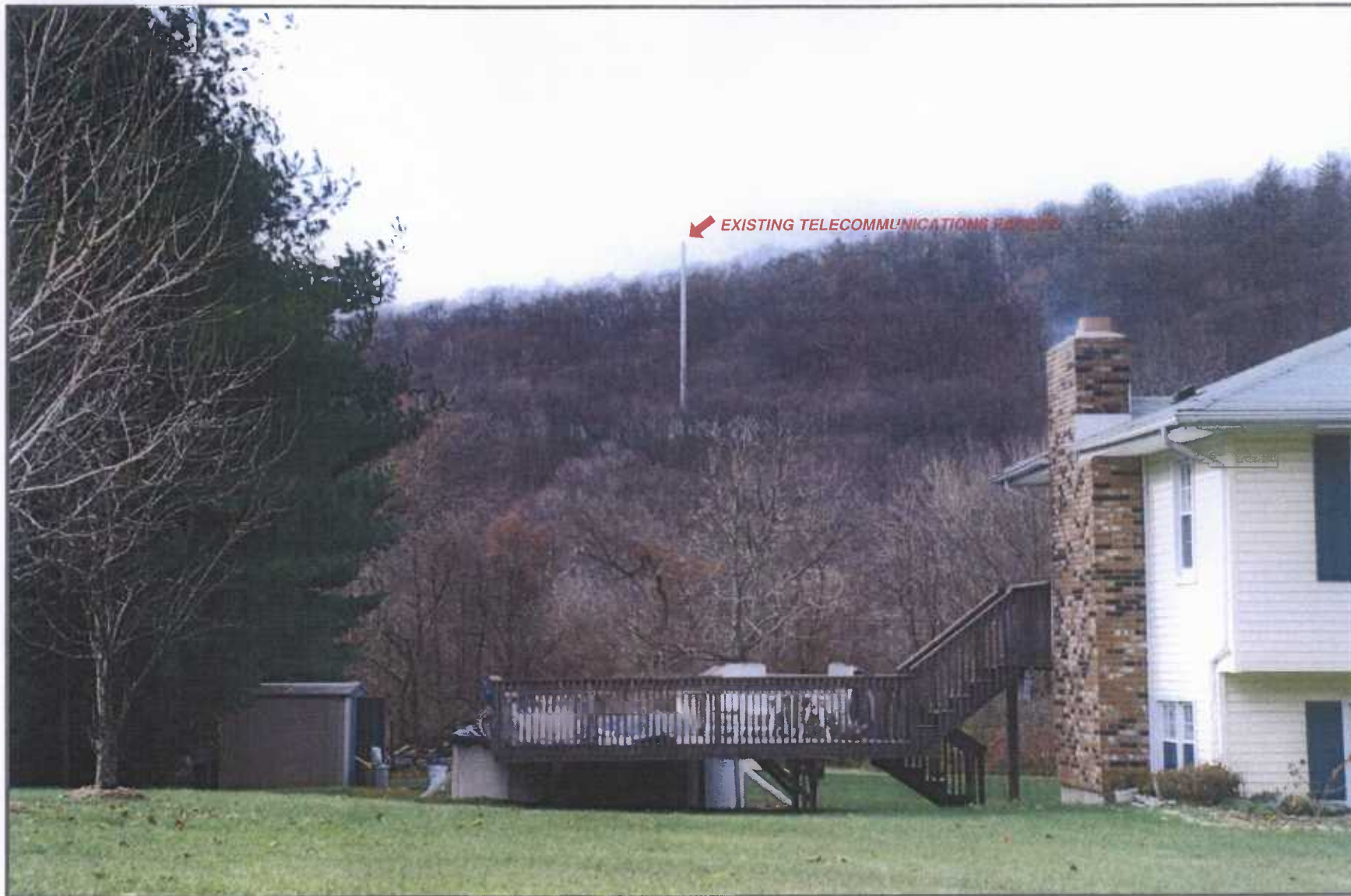
EXISTING 140 - FOOT TALL MONOPOLE (PHOTOGRAPHED NOVEMBER 2008 - ANTENNAS NOT INSTALLED AT THIS TIME), NEW MILFORD, CT
