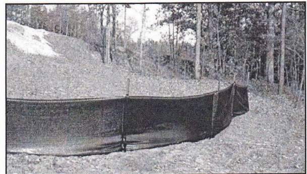
Mirafi® prefabricated Silt Fence.
