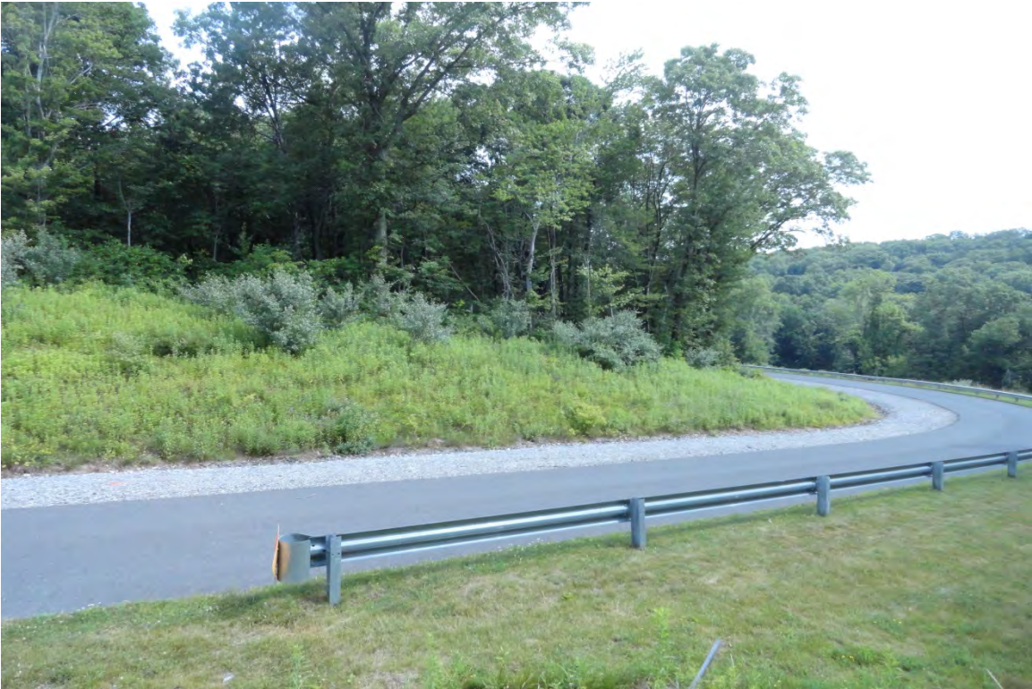
Photo 3: View of access road to compressor station looking northeast at the southeast corner of the Site. Photo date: July 3, 2014.
