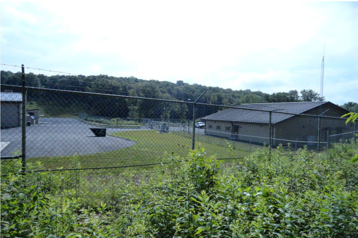
Photo 4: View of compressor station looking southeast from eastern property boundary of Site. Photo date: July 3, 2014.
