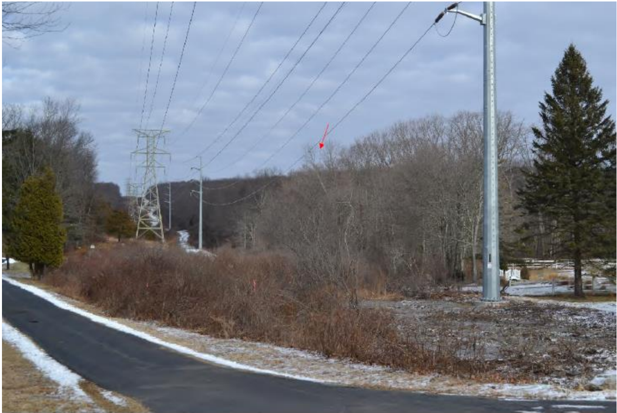
Photograph 4: Prokop Transmission ROW
