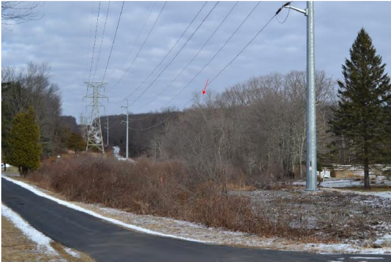
Photograph 4: Prokop Transmission ROW
