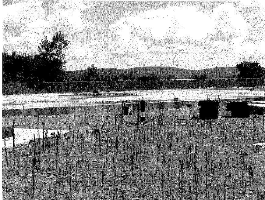
Foundation east of control- administration building
