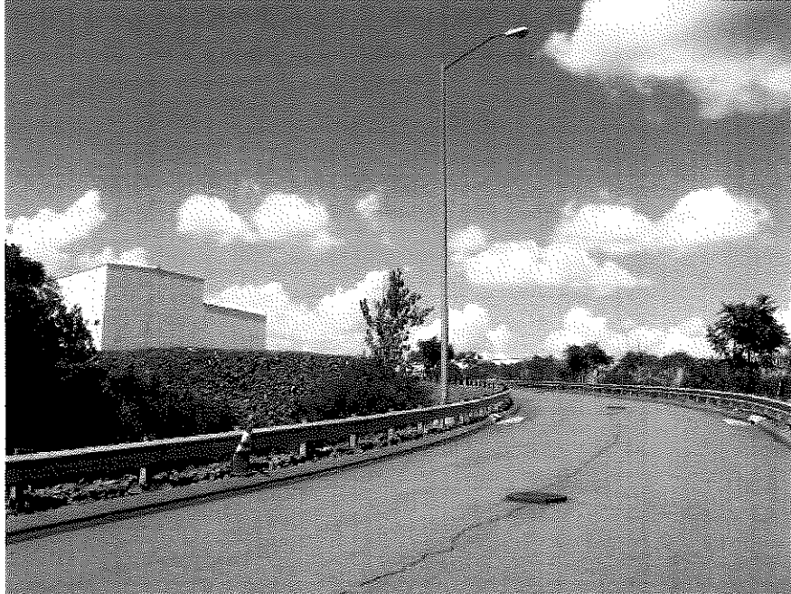
Access Road Looking to Power Plant
