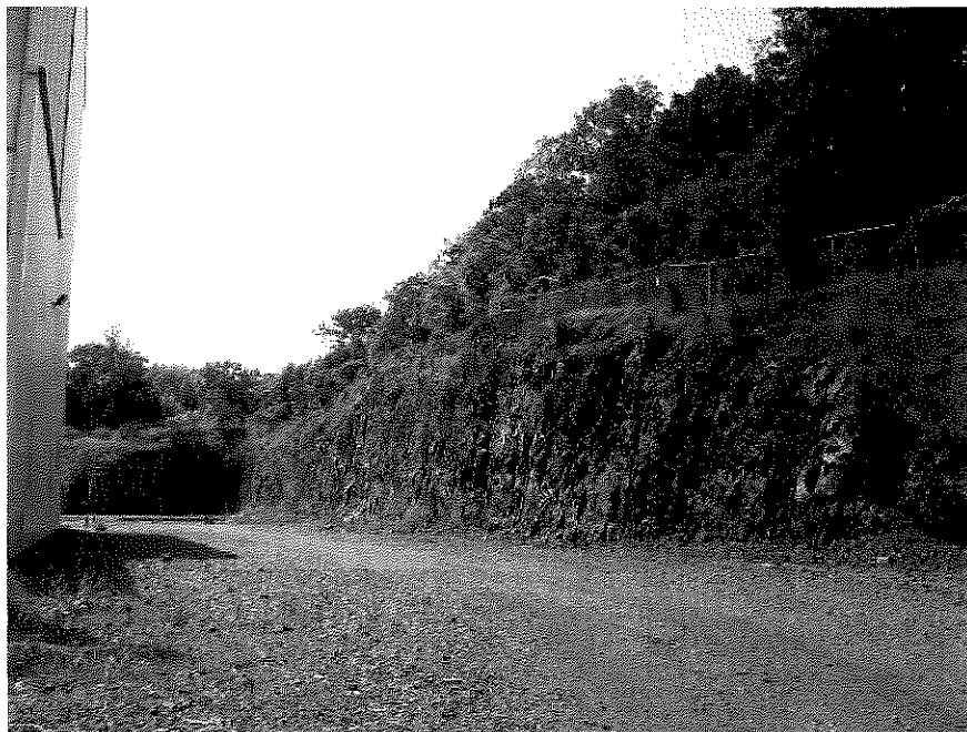
Site north of power plant looking west at rear of power plant building
