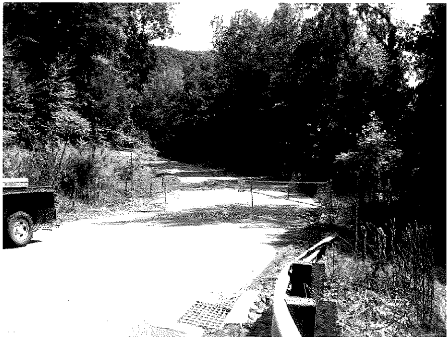
Entry to South Mountain Road from Route 71
