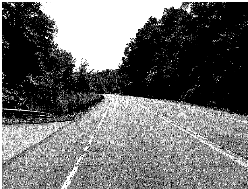
Route 71 Looking South
