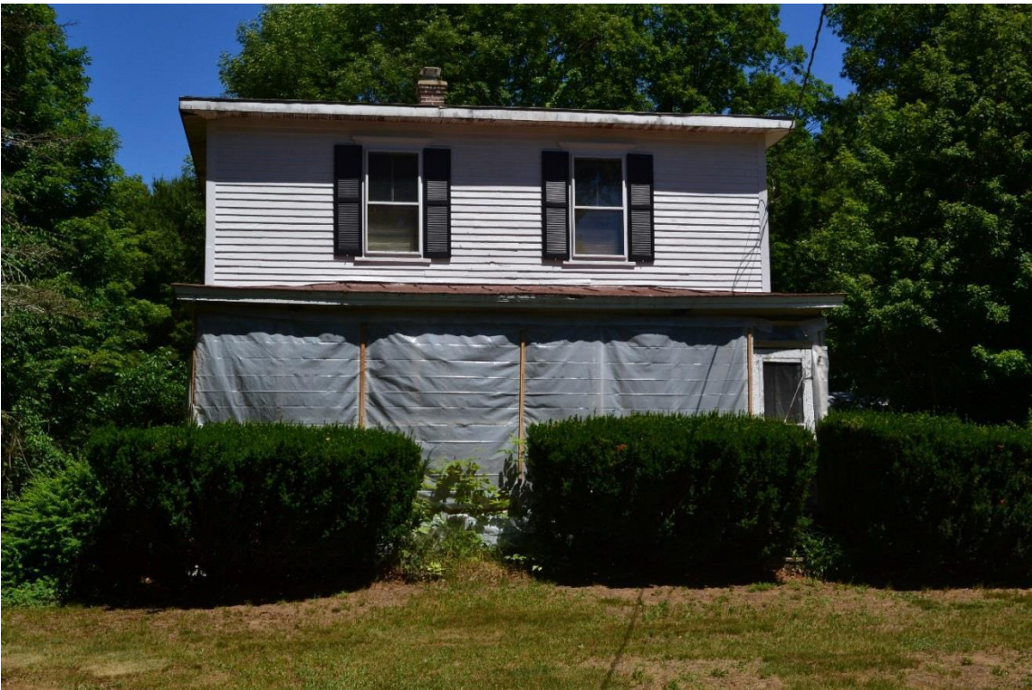
Photograph 2. Looking north at the Sorrow House (James Sexton, Tetra Tech, June 30, 2016).
