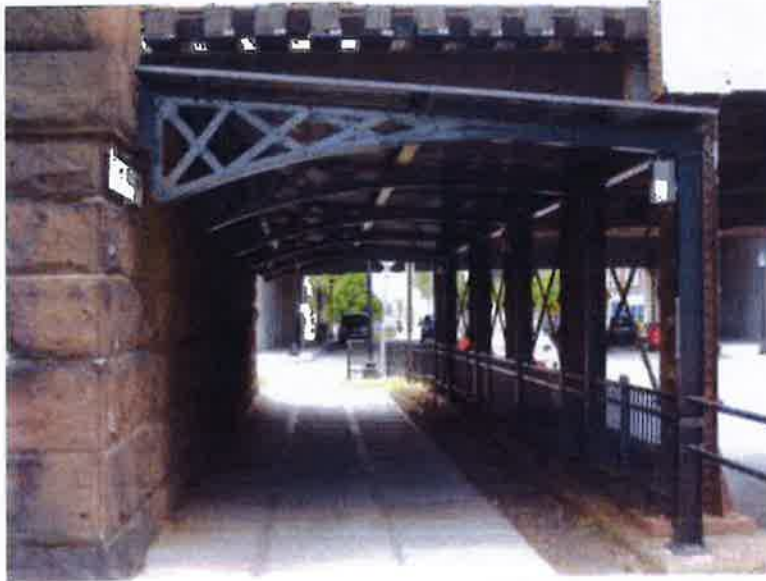
A Pedestrian Friendly Underpass Treatment in Stratford, CT
