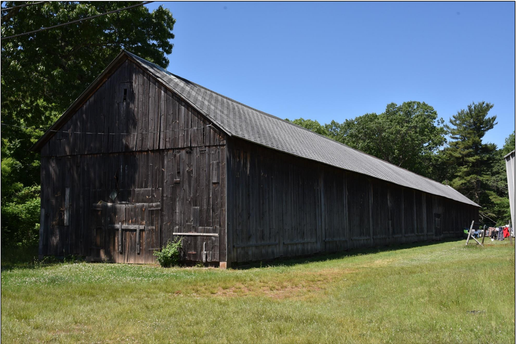
Photo 50: Shed 19, view southwest.
