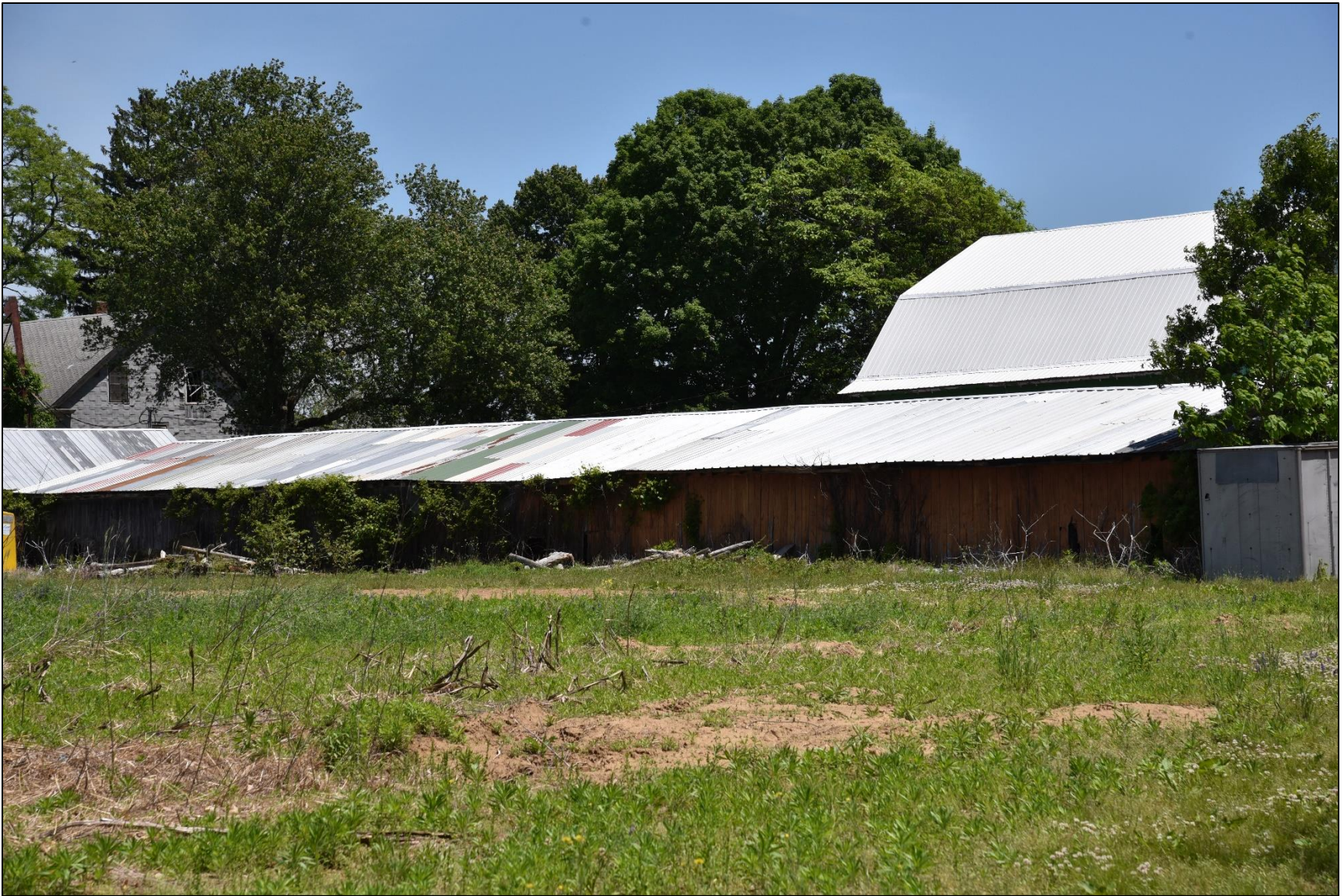
Photo 71: Barn 3—Pole barn open, view northeast.
