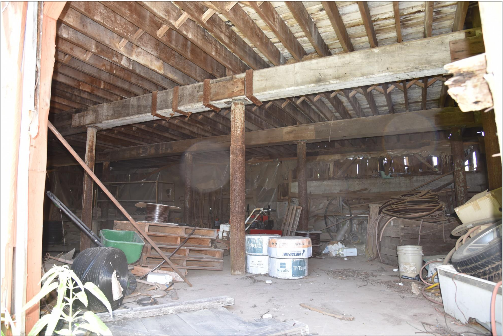
Photo 70: Barn 2—English bank barn, interior.
