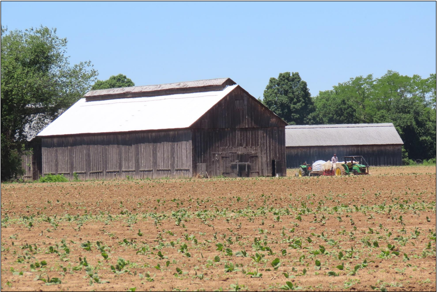
Photo 54: Shed 25 (foreground) and Shed 28 (background), view west.
