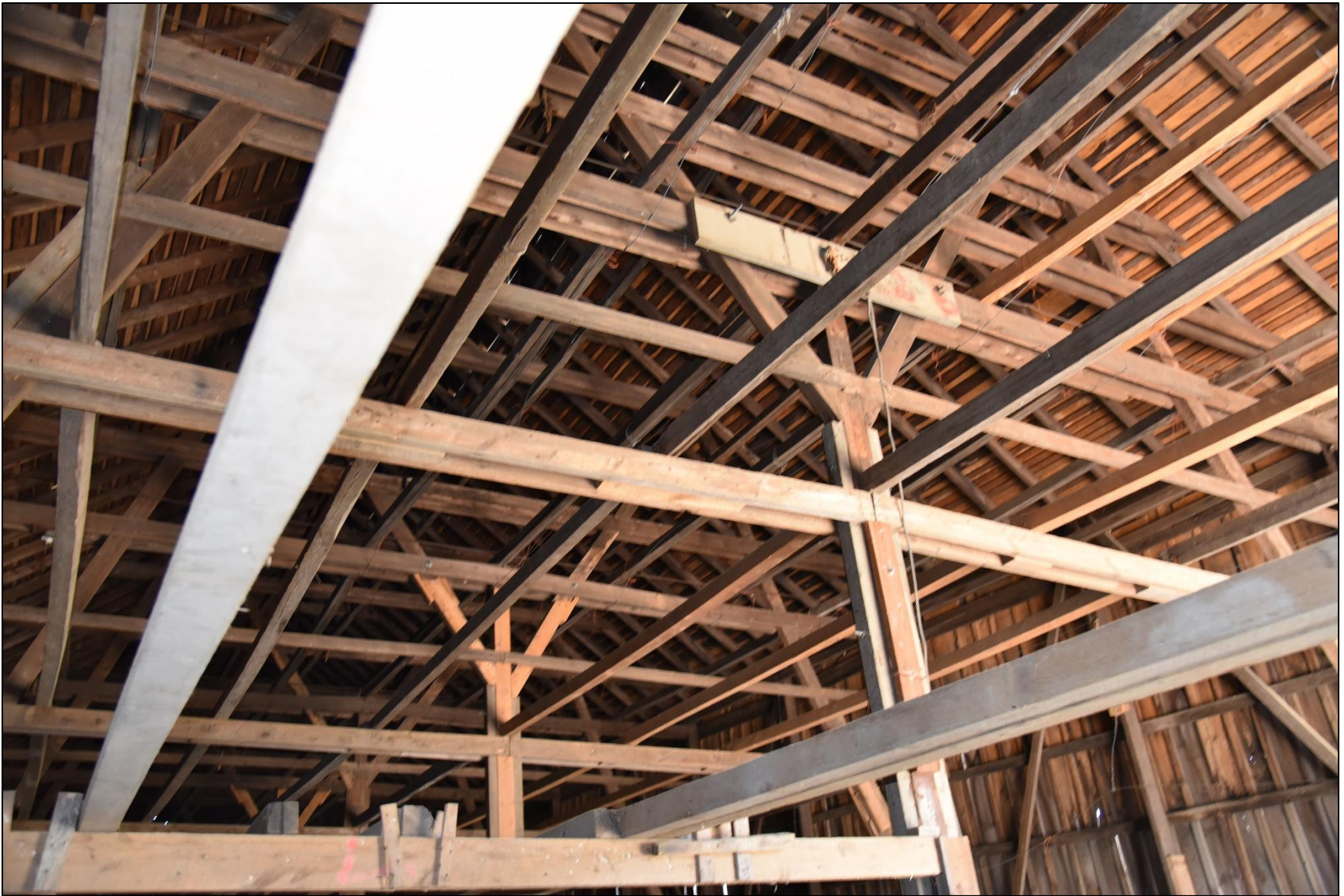
Photo 41: Shed 1, interior framing detail.
