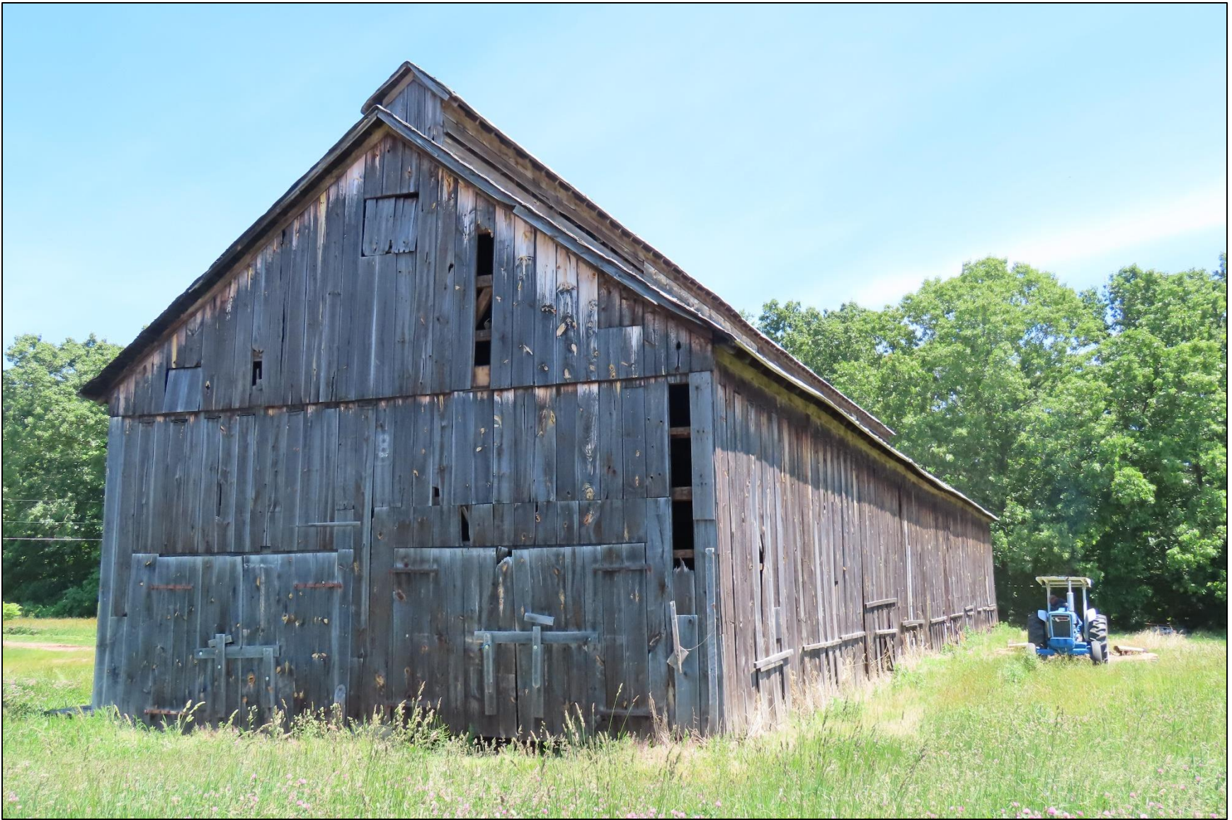
Photo 18; Shed 8, view northeast.
