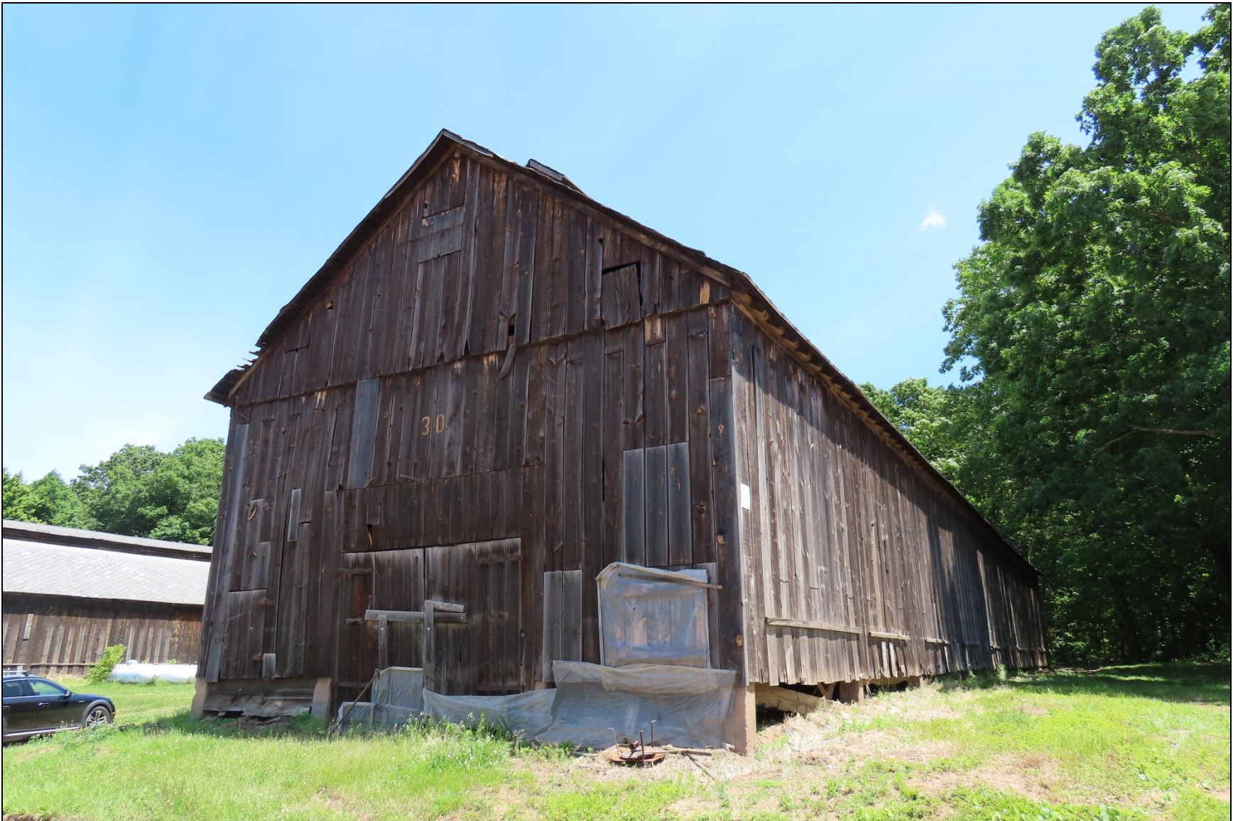
Photo 38: Shed 30, view northeast.
