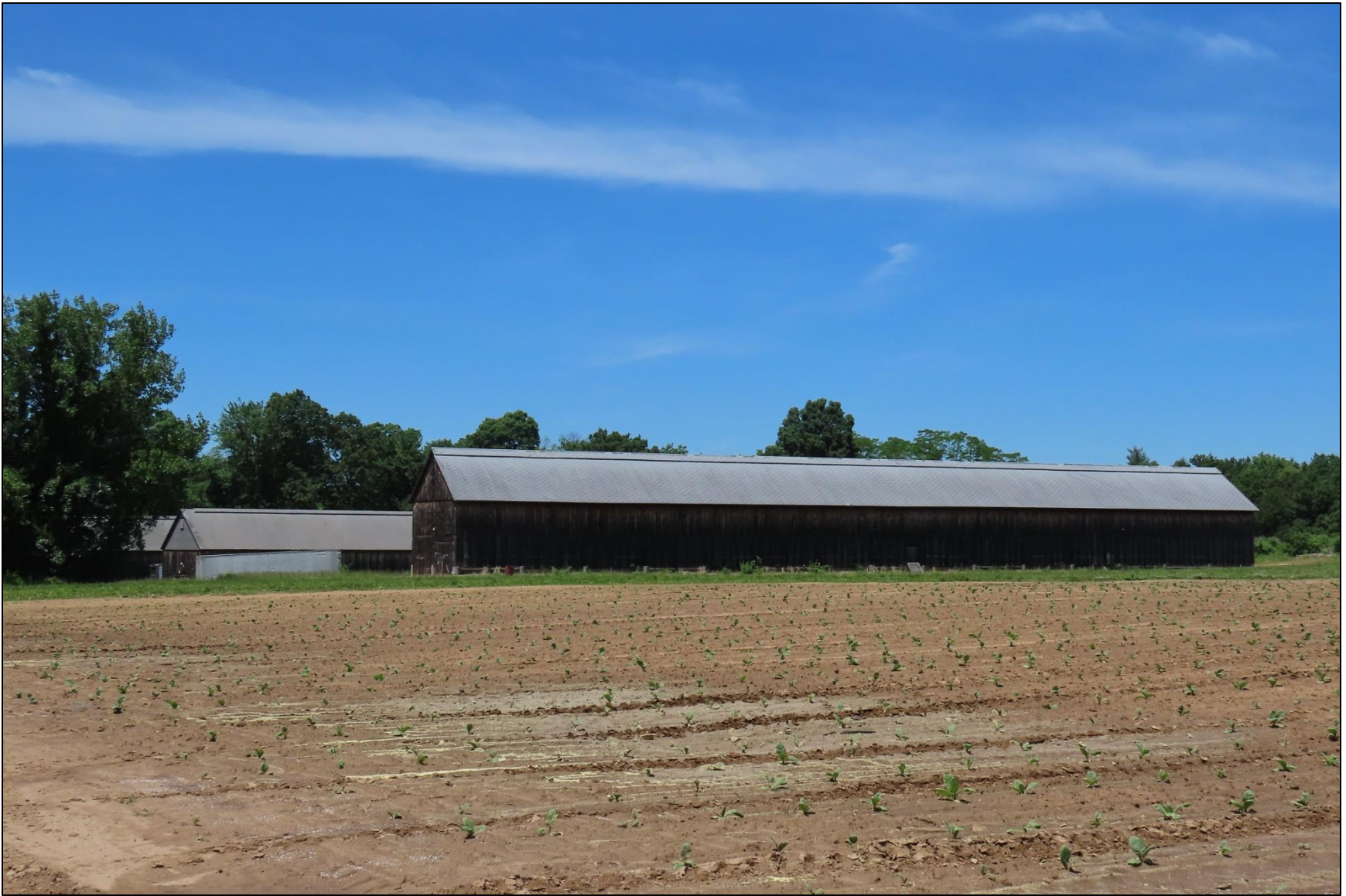
Photo 57: Shed 27 (foreground) and Sheds 32 and 33 (background), view west.
