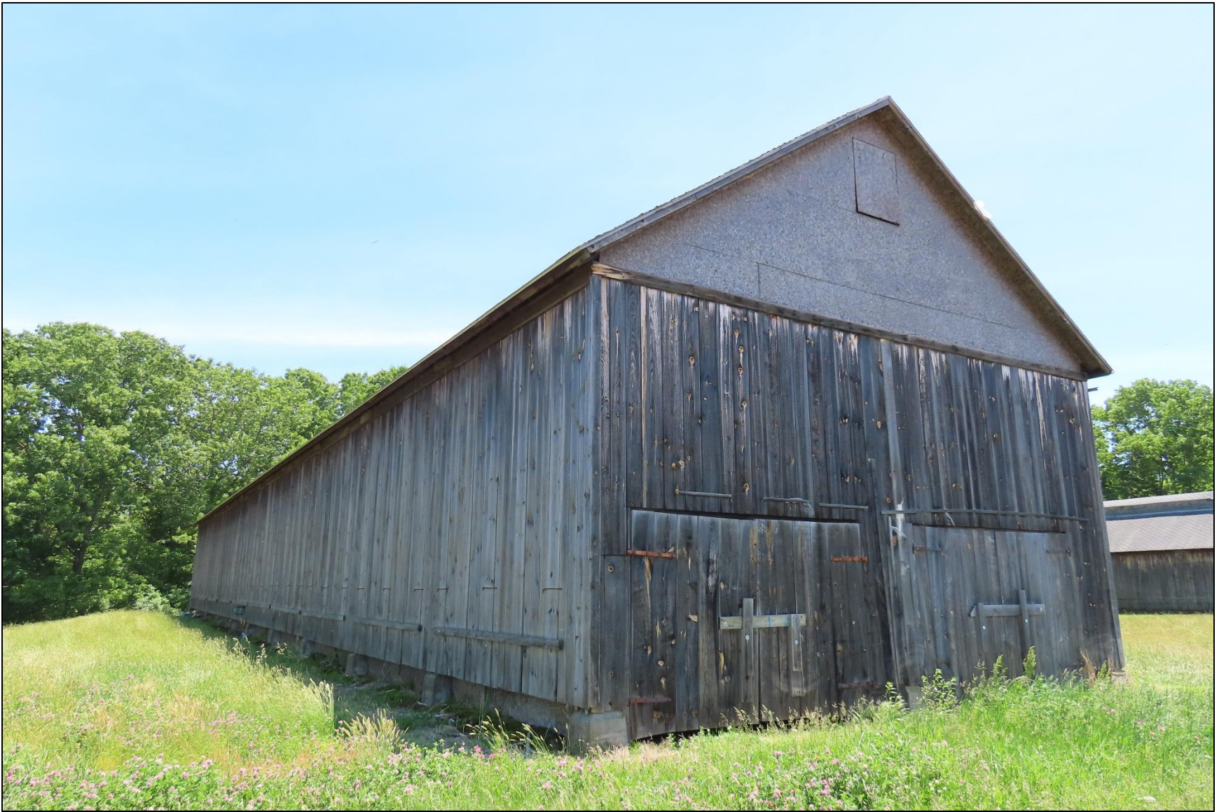
Photo 56: Shed 9, view northwest.
