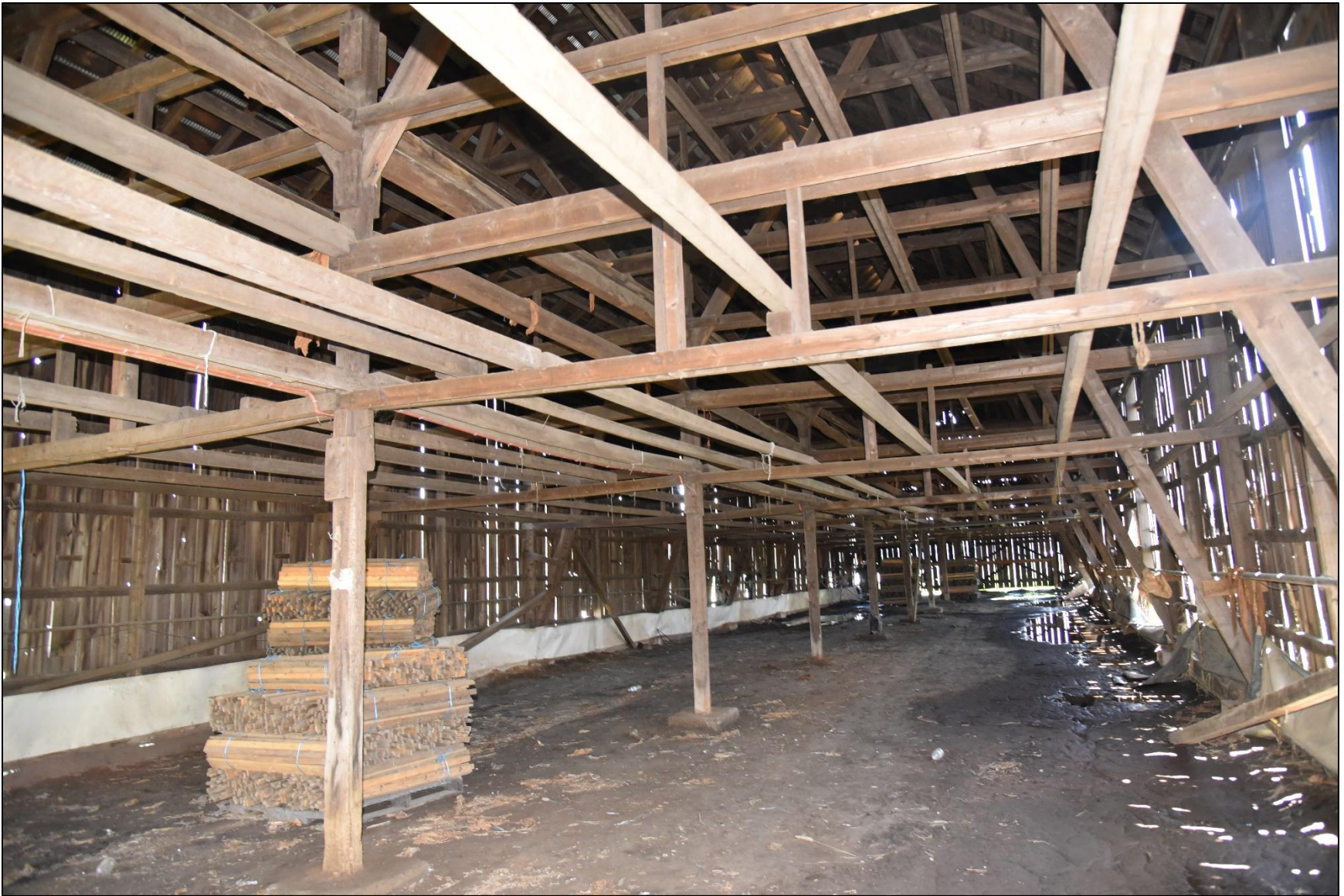
Photo 48: Shed 4, interior detail.
