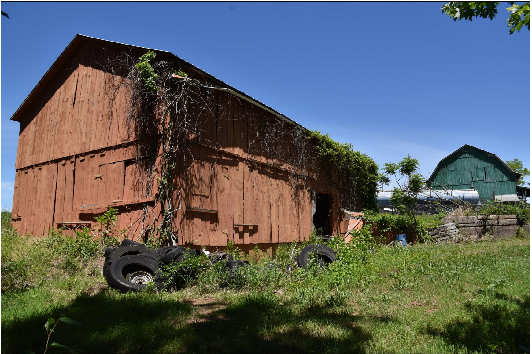
Photo 68: Barn 2—English bank barn, view north.
