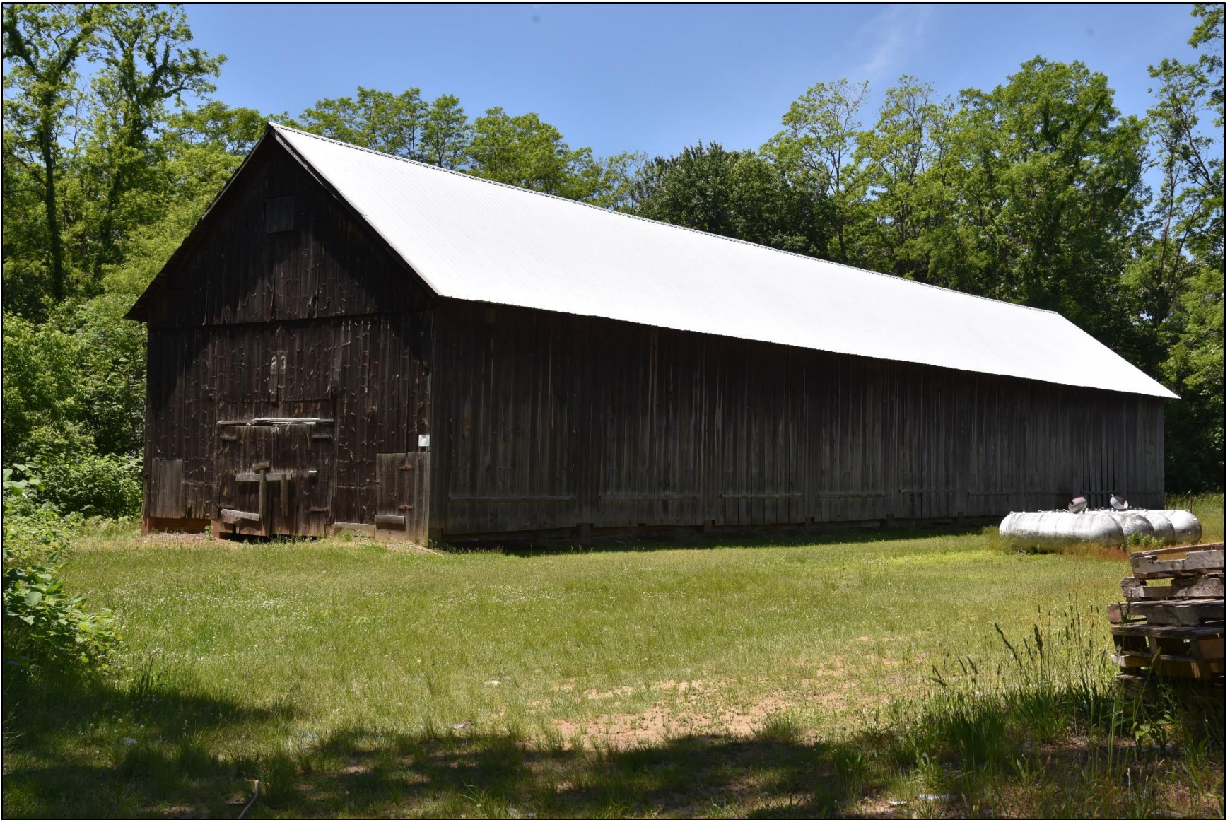
Photo 53: Shed 23, view west.
