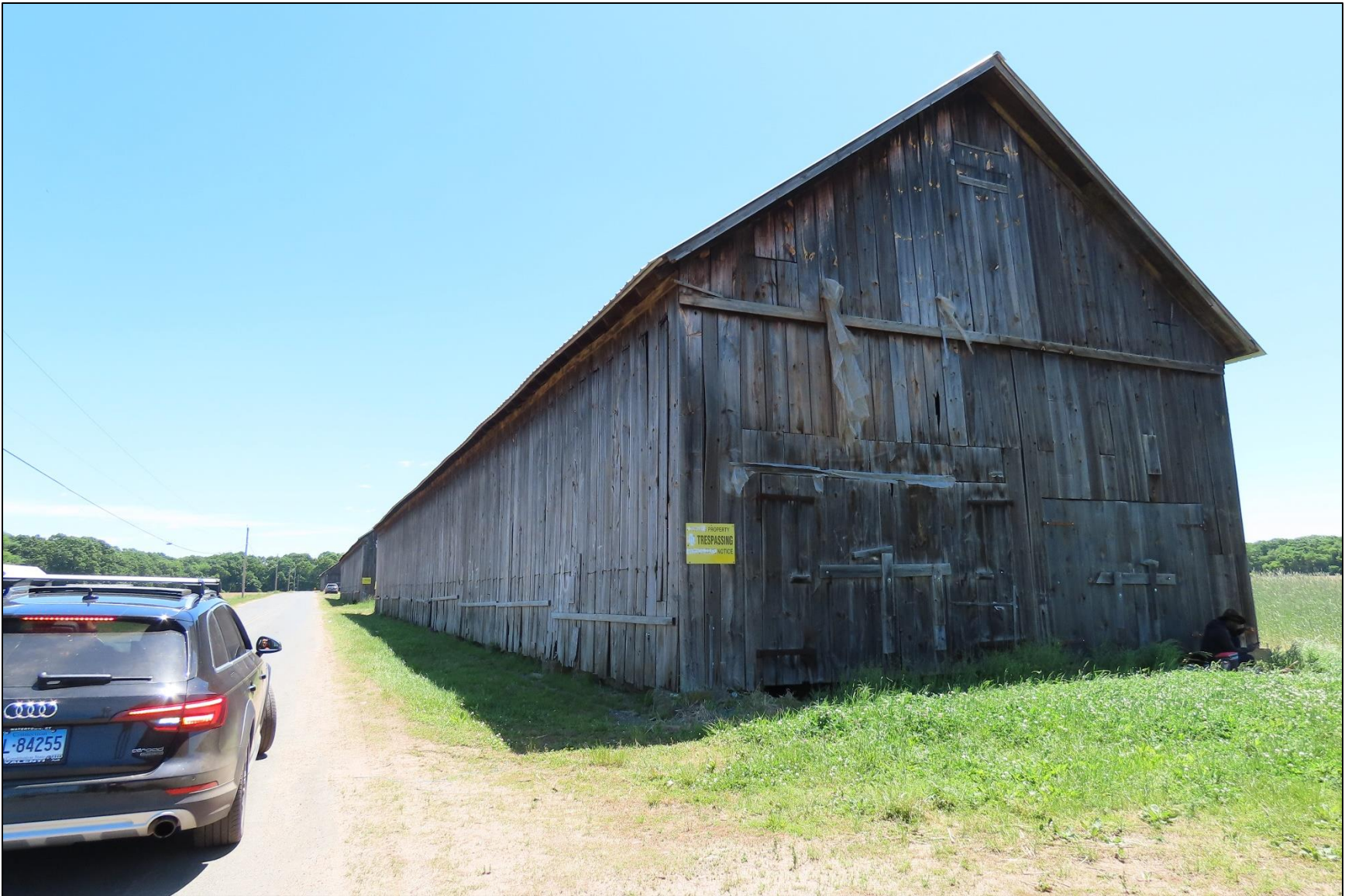
Photo 44: Shed 3, view east along Planation Road.
