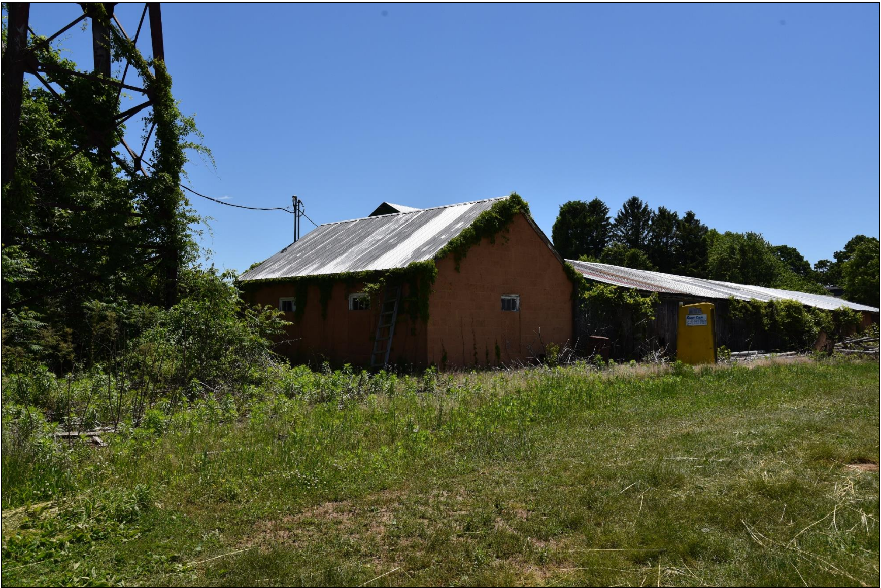
Photo 73: Barn 4—Concrete barn near pole barn.
