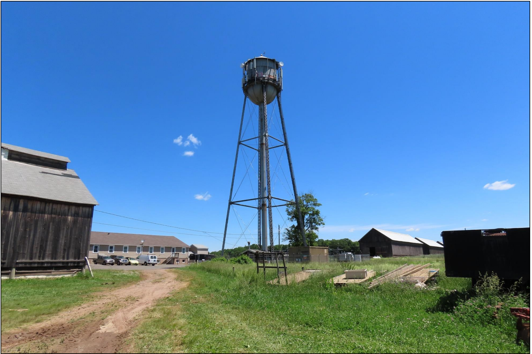
Photo 76: Water tower, view northeast.
