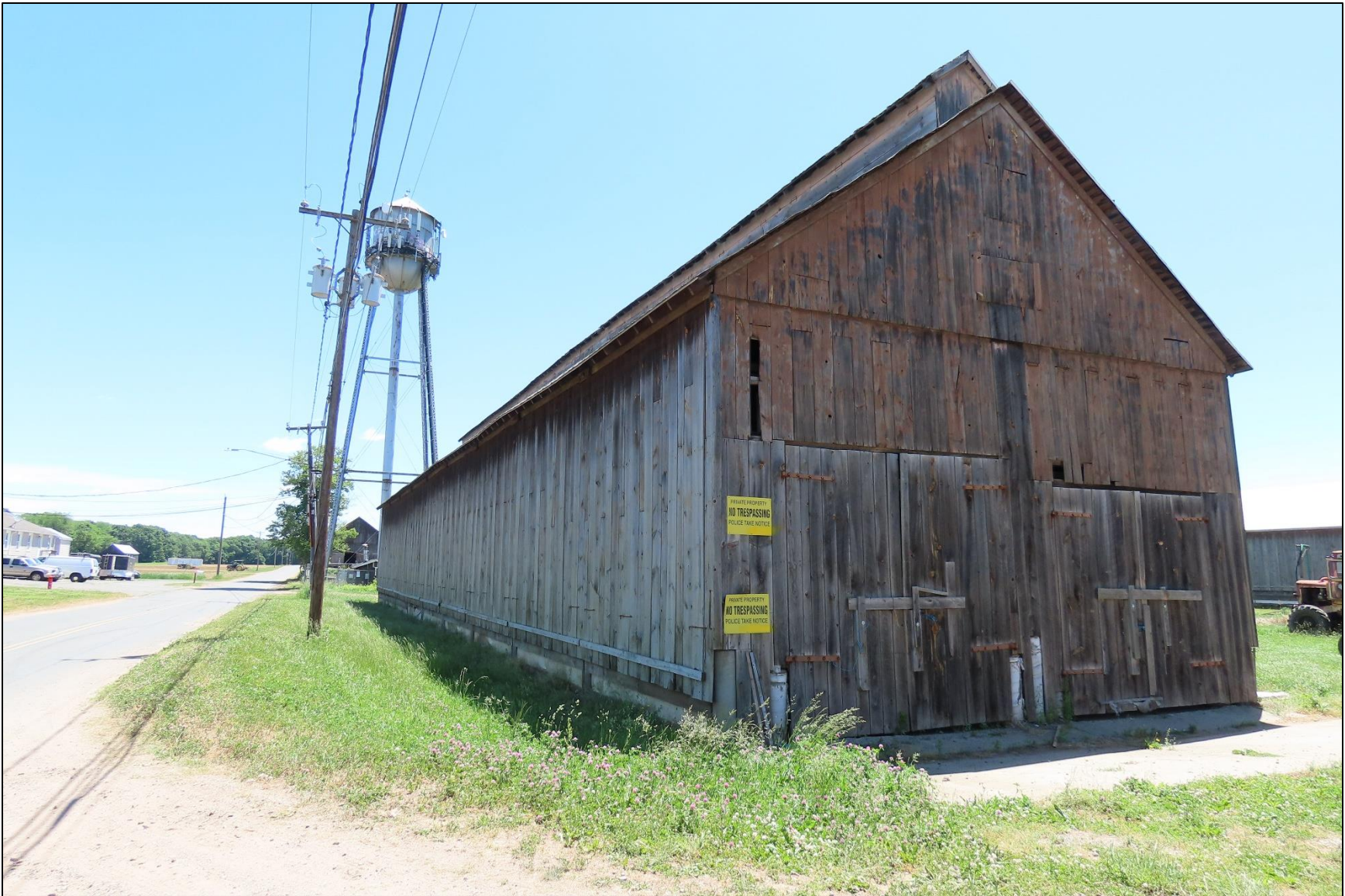
Photo 39: Shed 1, view east along planation road.
