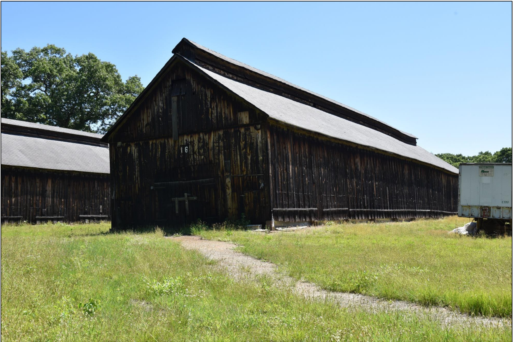
Photo 28: Shed 16, view east.
