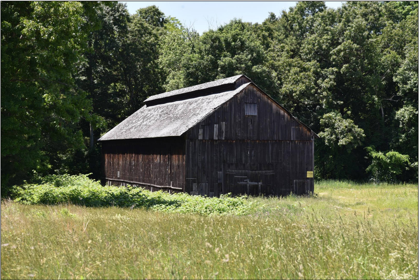
Photo 23: Shed 14, view northwest.
