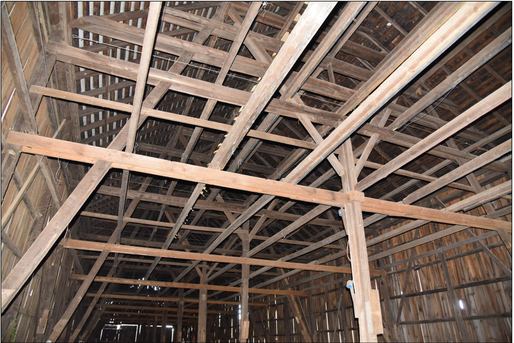
Photo 43: Shed 2, framing detail.
