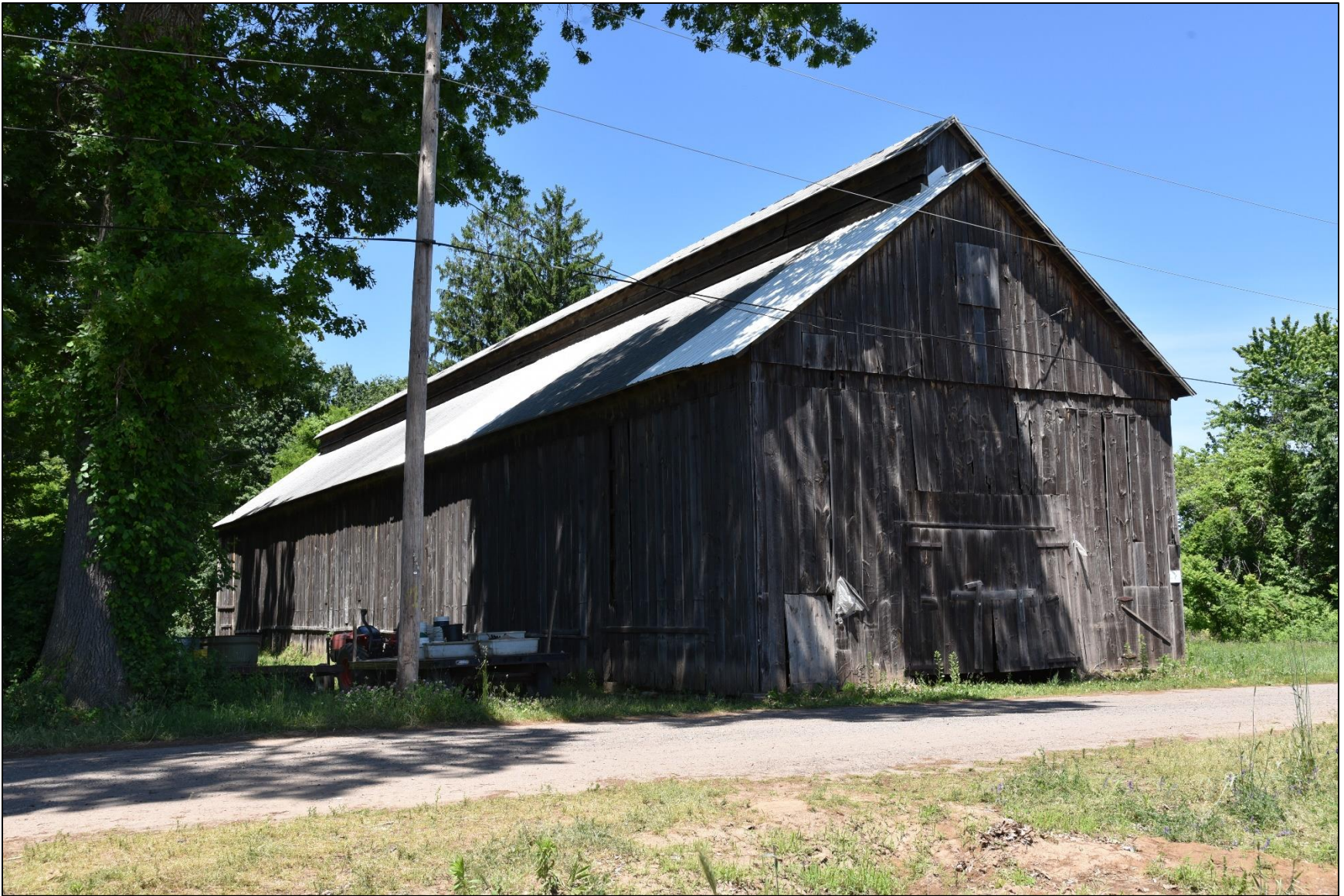
Photo 33: Shed 22, view north.
