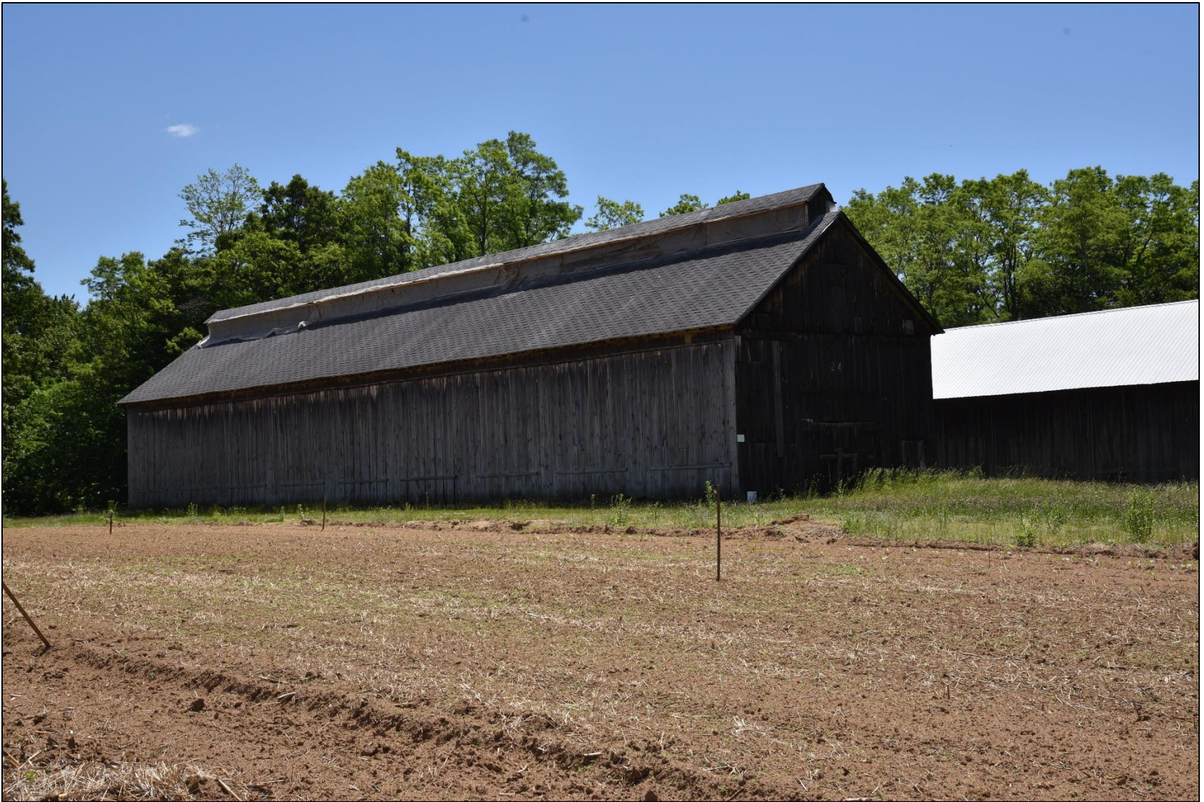
Photo 34: Shed 24, view southeast.
