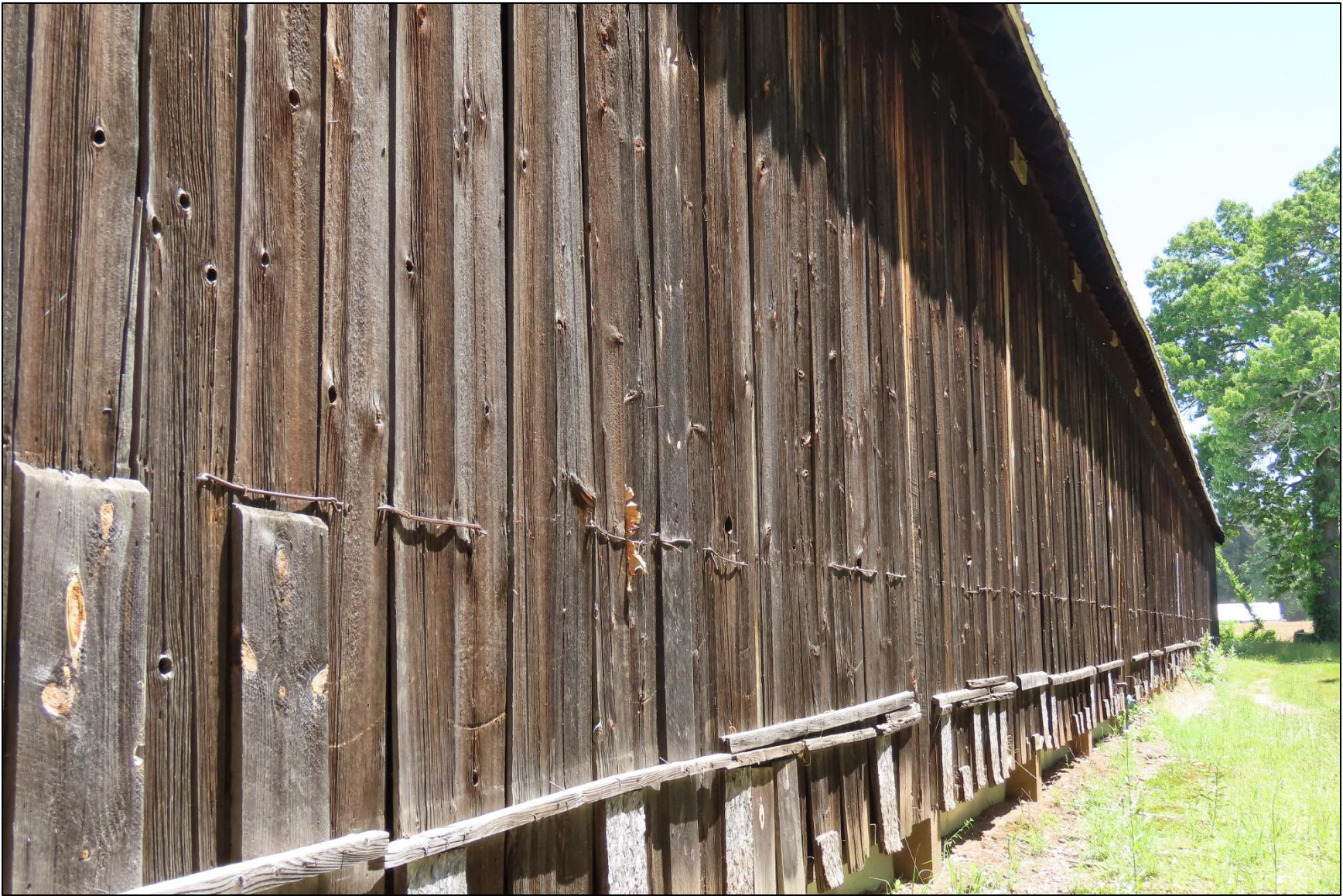
Photo 31: Shed 18, siding detail.
