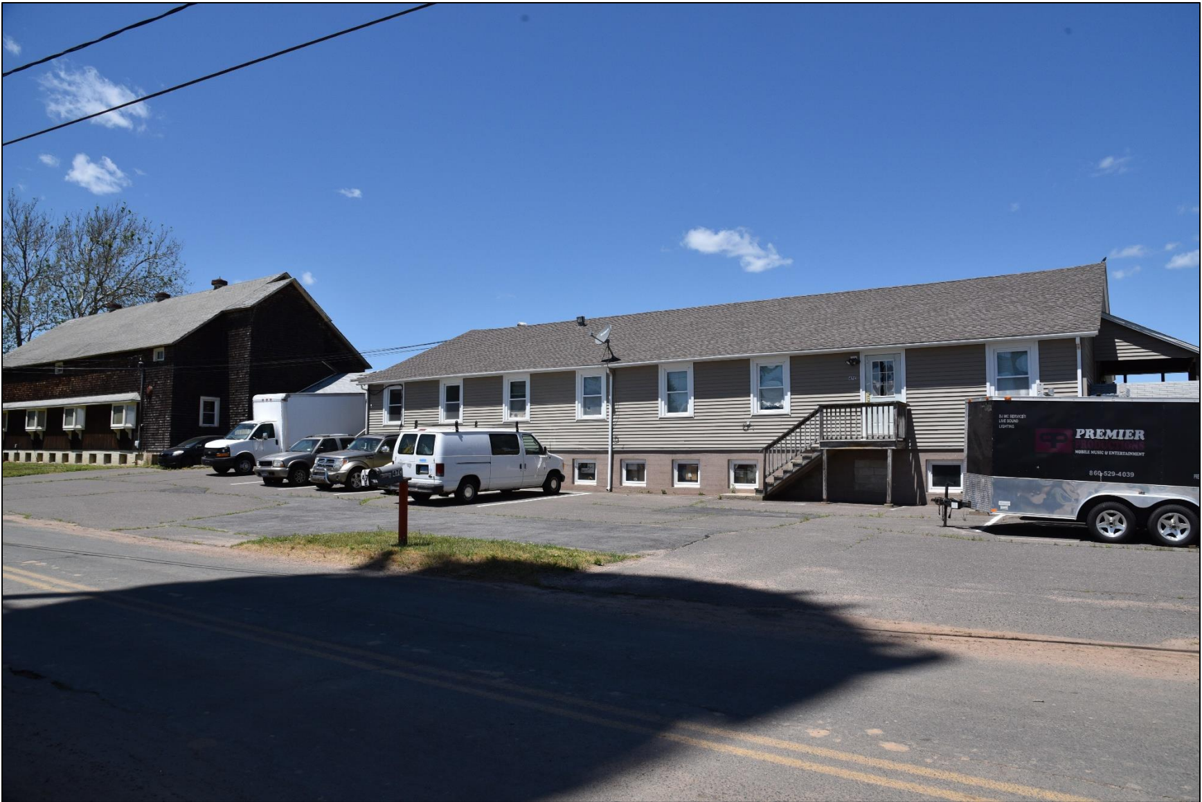
Photo 75: Barn 5-converted barn/dormitory, view west.
