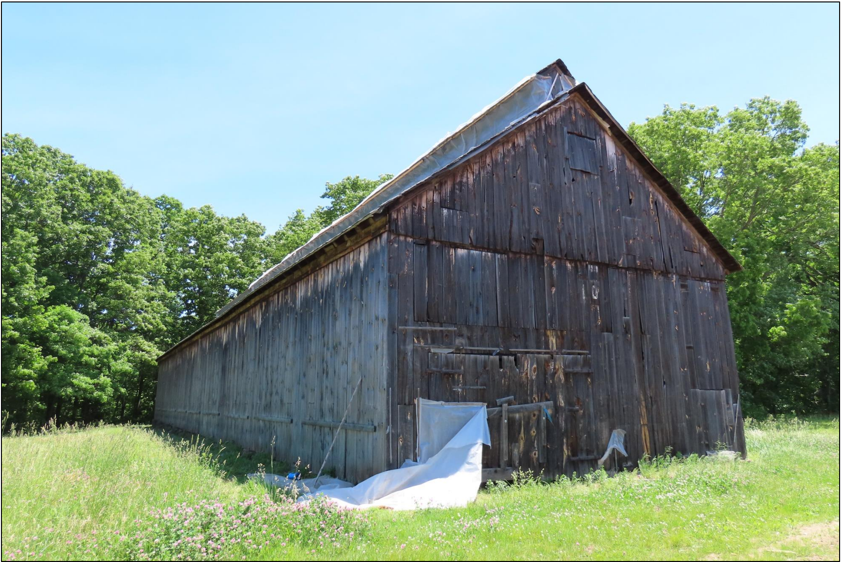
Photo 19: Shed 10, view southeast.
