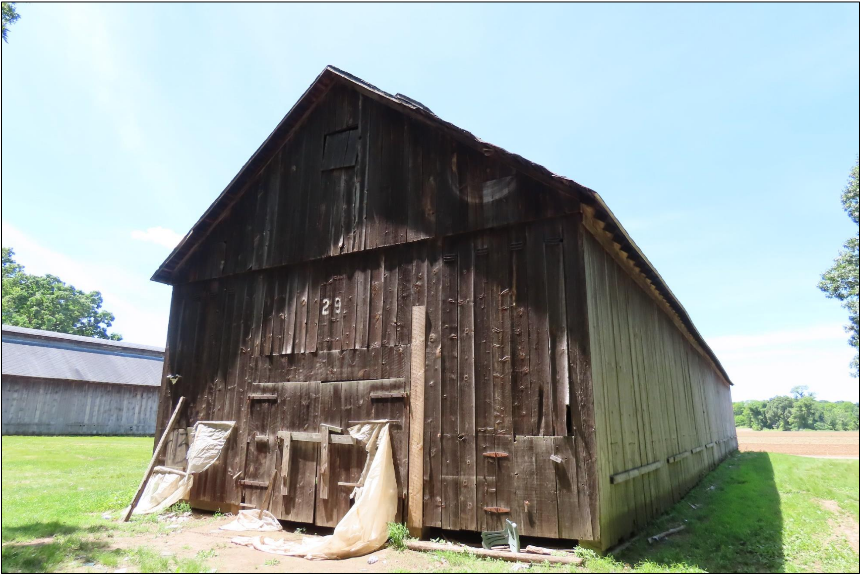
Photo 37: Shed 29, view southwest.
