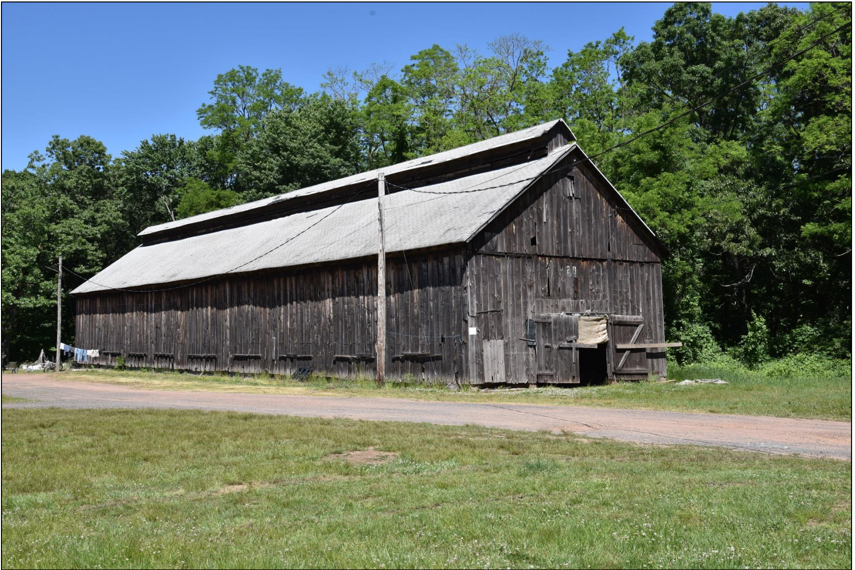
Photo 32: Shed 20, view northwest.
