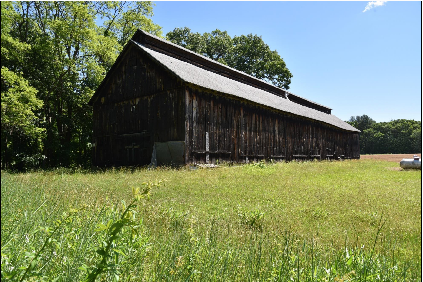
Photo 29: Shed 17, view north.
