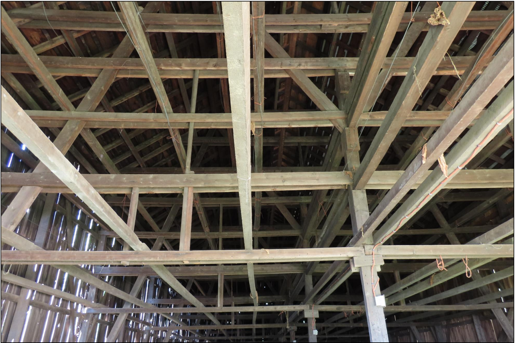
Photo 25: Shed 15 interior framework detail.
