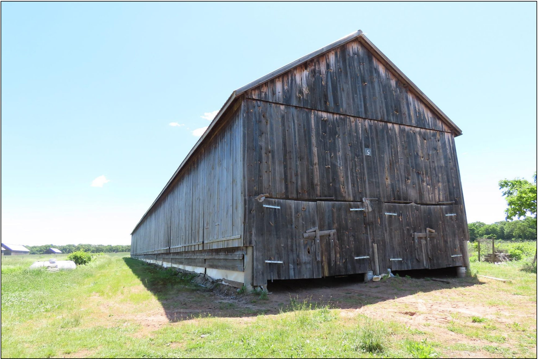
Photo 49: Shed 6, view southeast.
