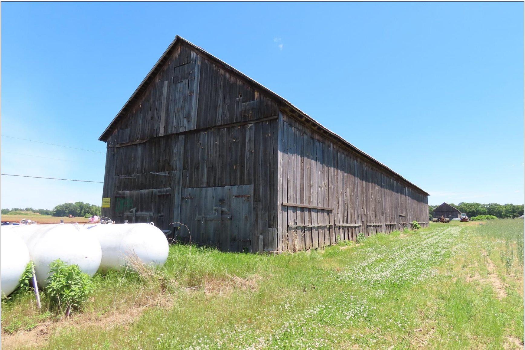
Photo 47: Shed 4, view east.
