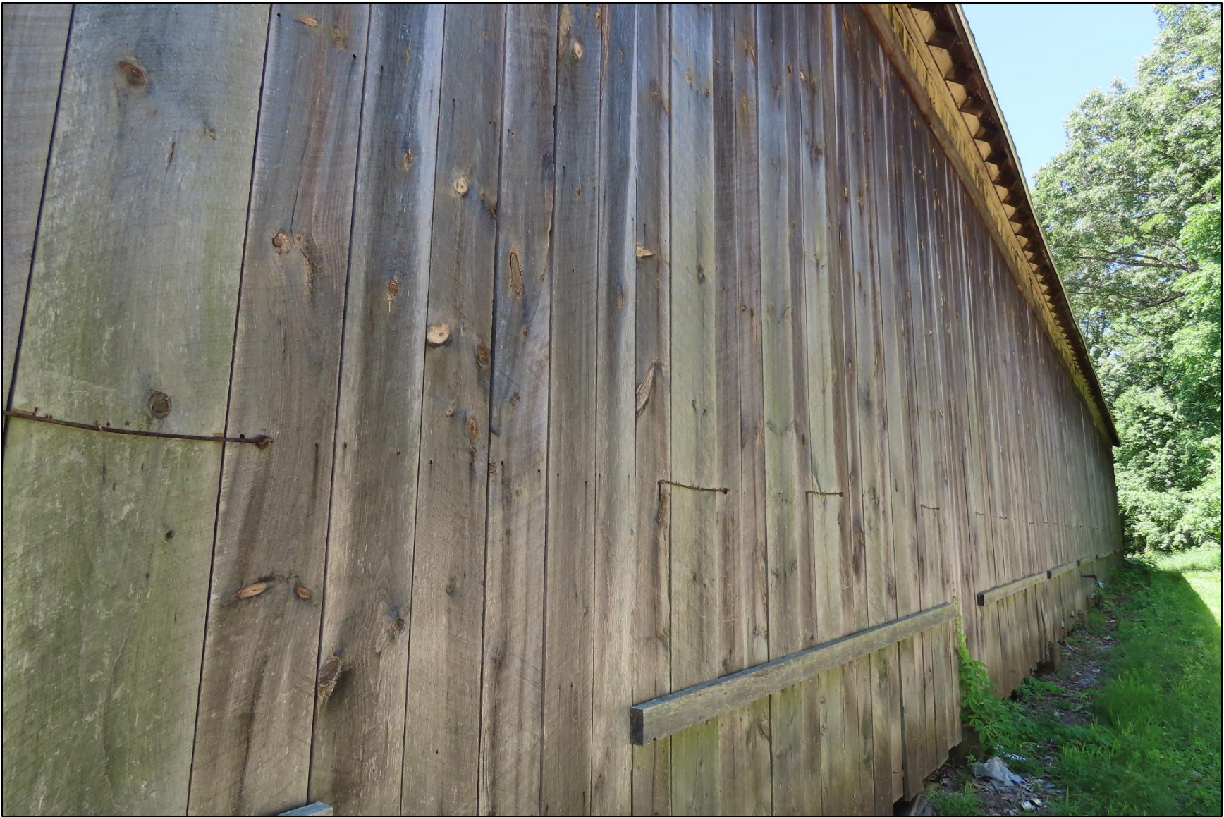
Photo 27: Shed 15 siding detail.
