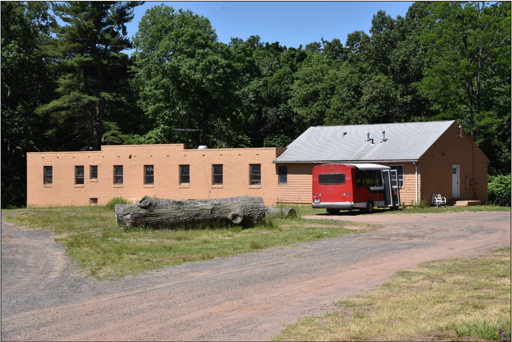
Photo 65: Dormitory between Sheds 19 and 20, view west.
