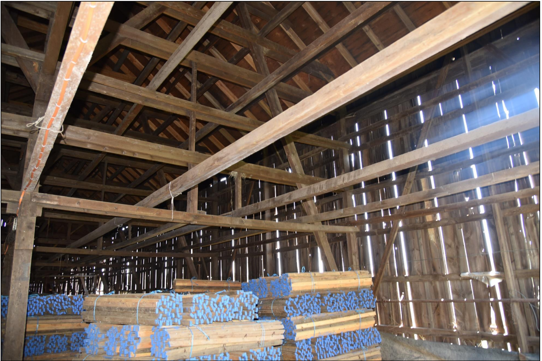
Photo 46: Shed 3, interior detail.
