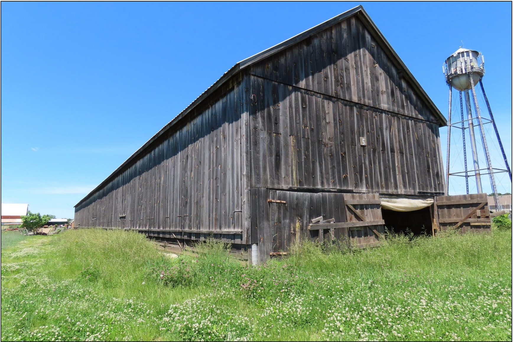
Photo 58: Shed 5, view northwest.
