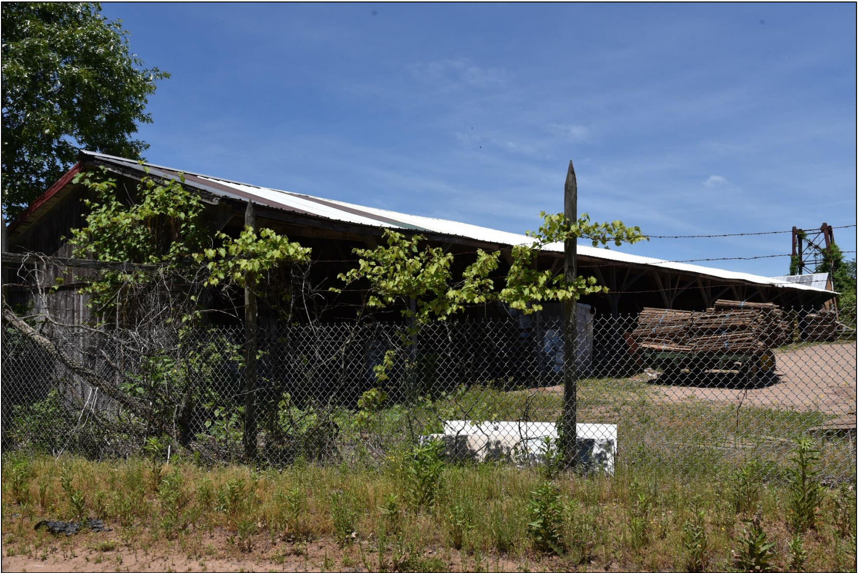
Photo 71: Barn 3—Pole barn open, view northwest.
