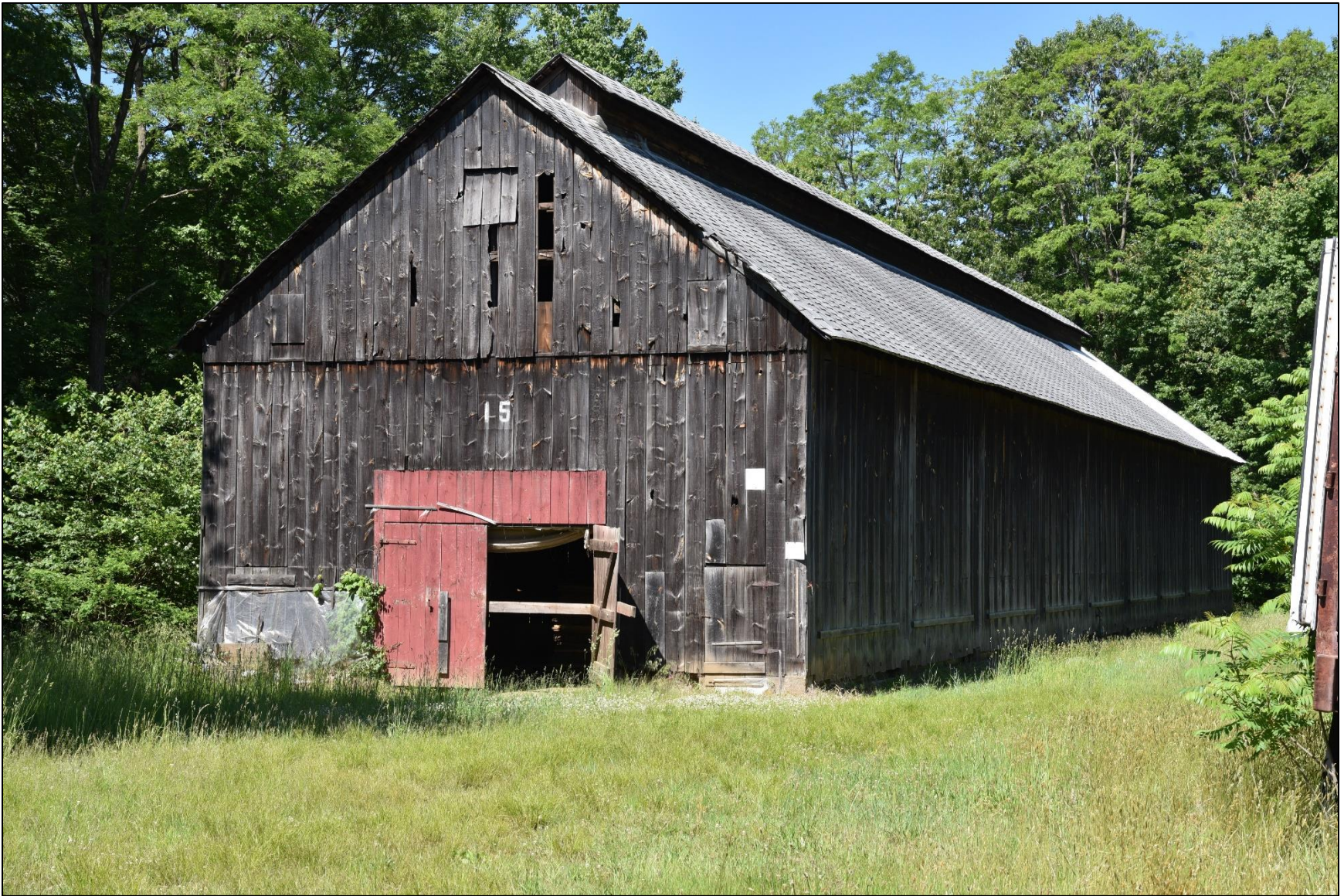
Photo 24: Shed 15, view southwest.
