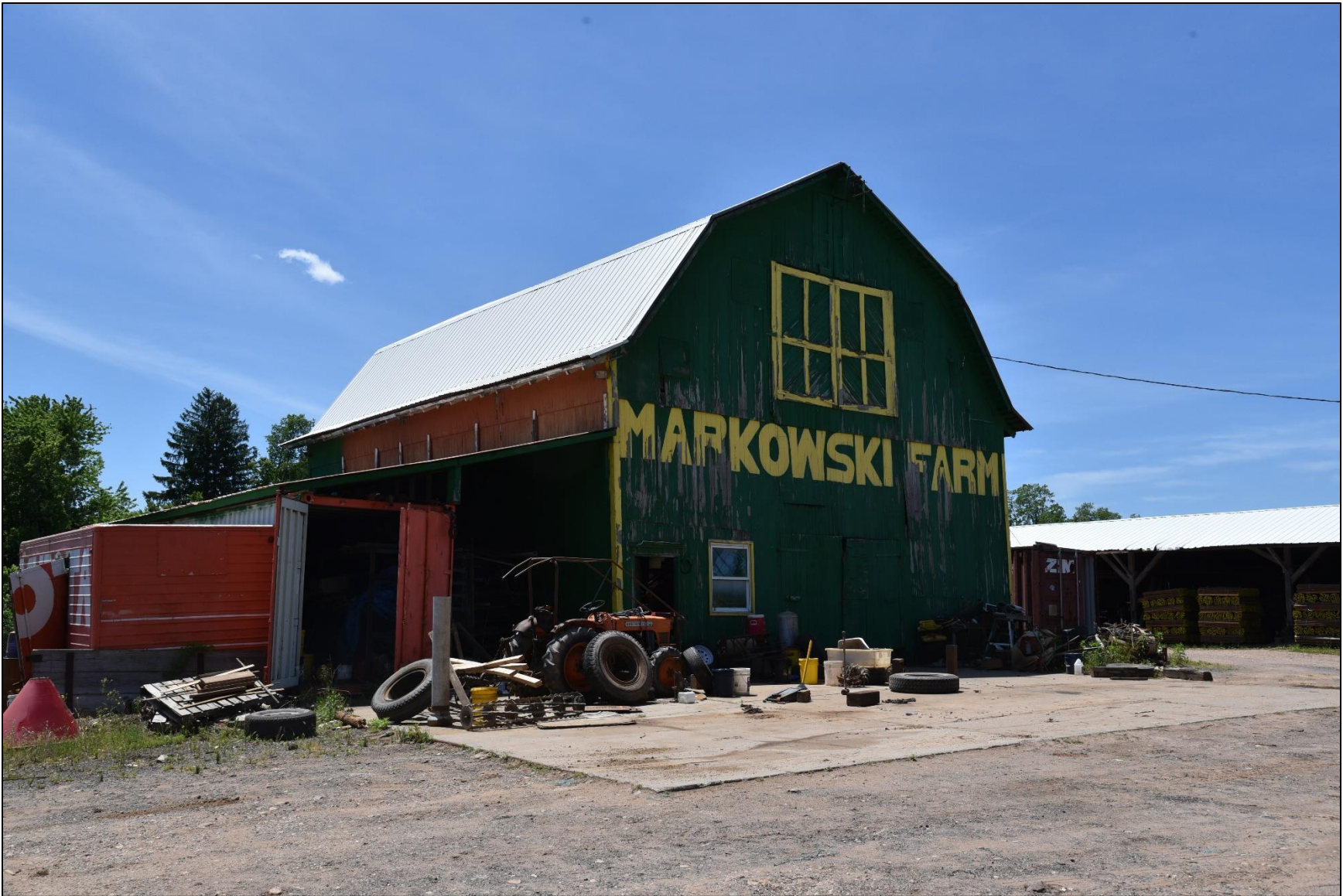
Photo 66: Barn 1-Markowski Barn, view southwest.
