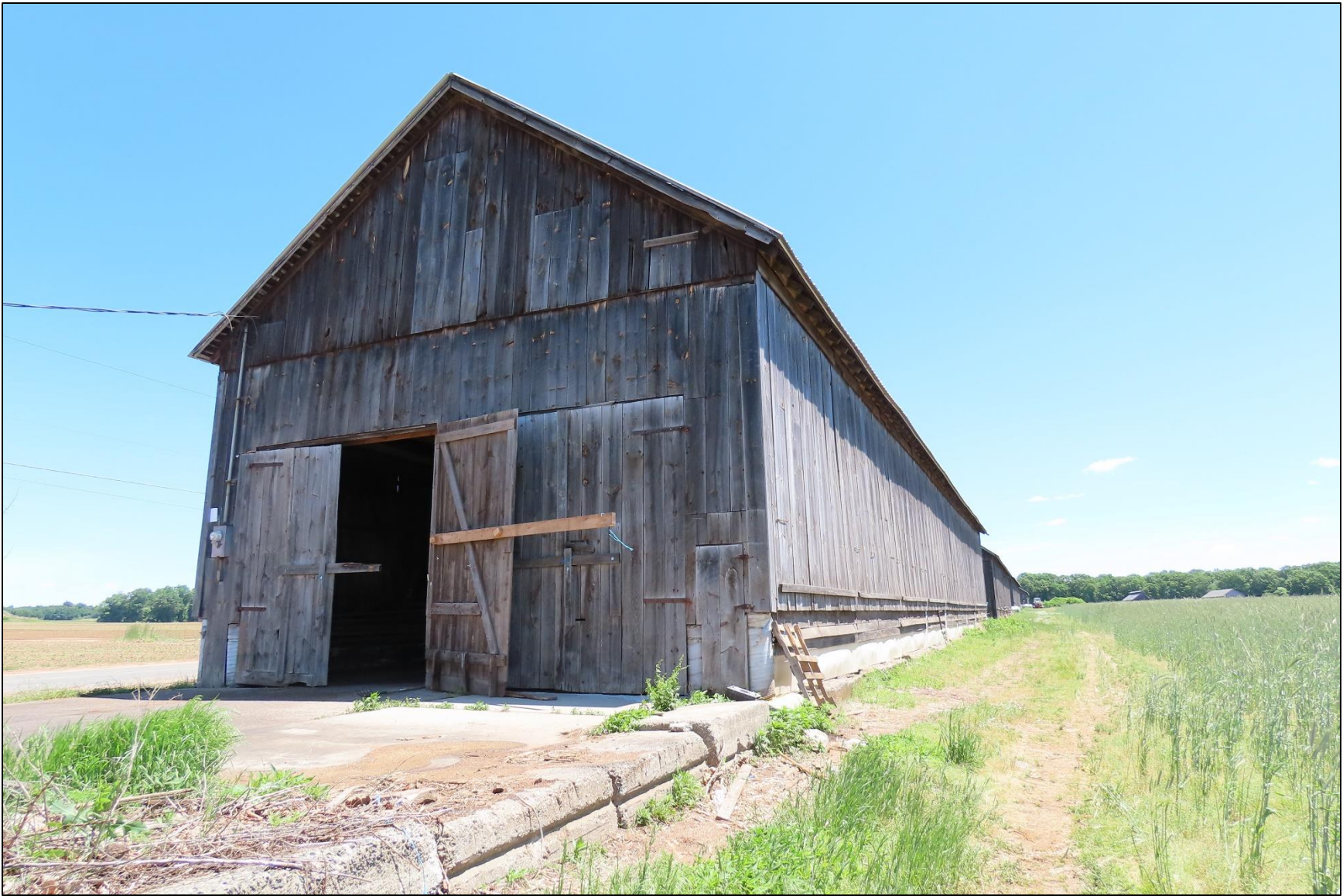
Photo 42: Shed 2, view east along Plantation Road.
