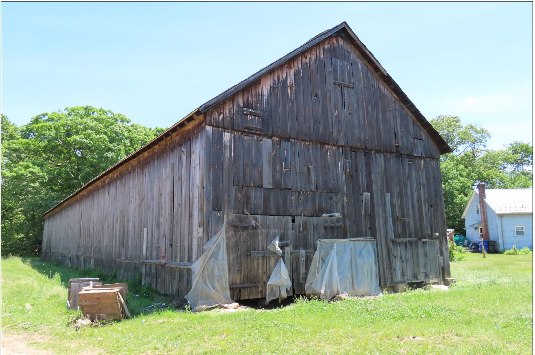
Photo 20. Shed 11, view Northwest.
