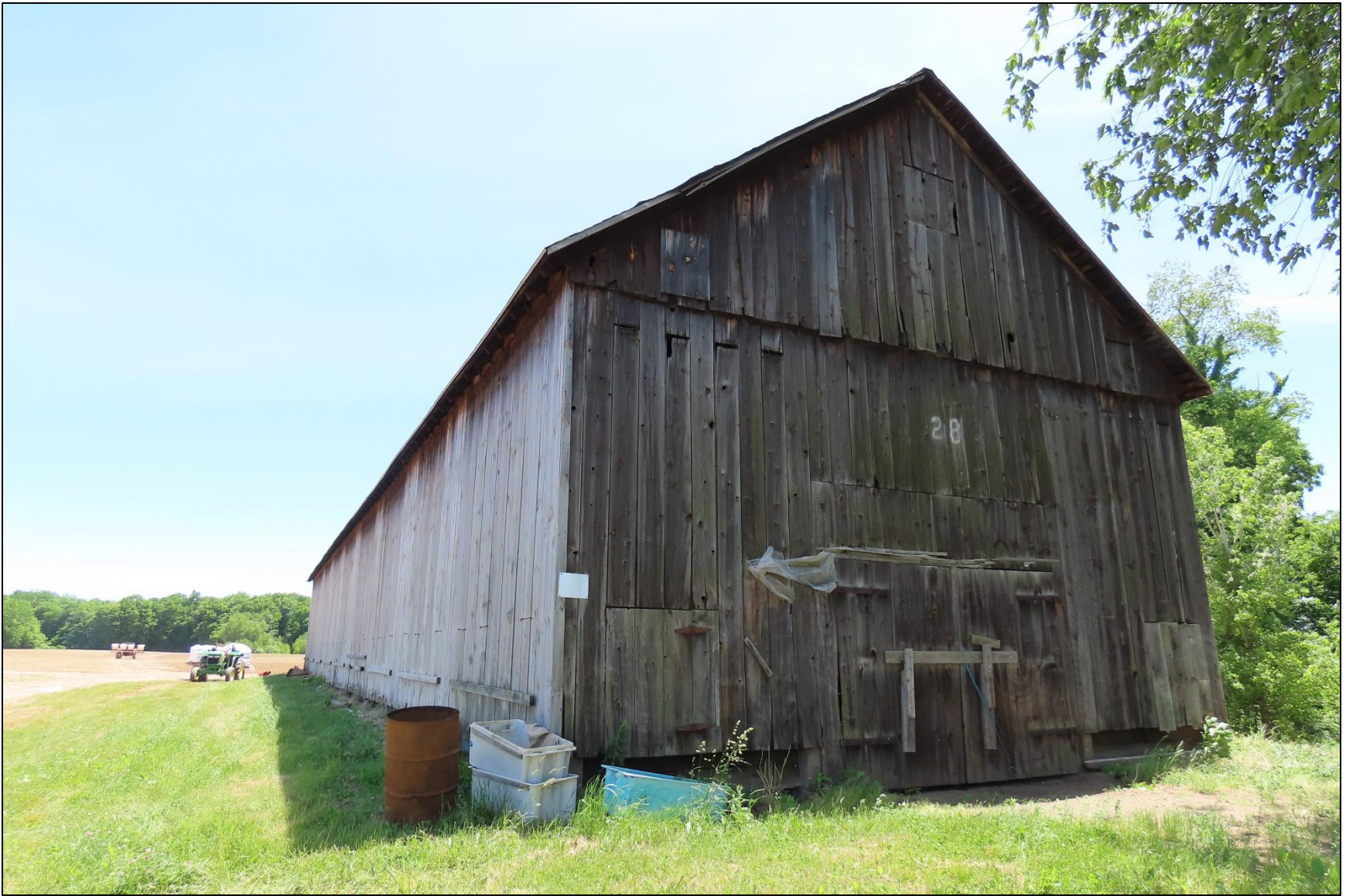
Photo 36: Shed 28, view northwest.
