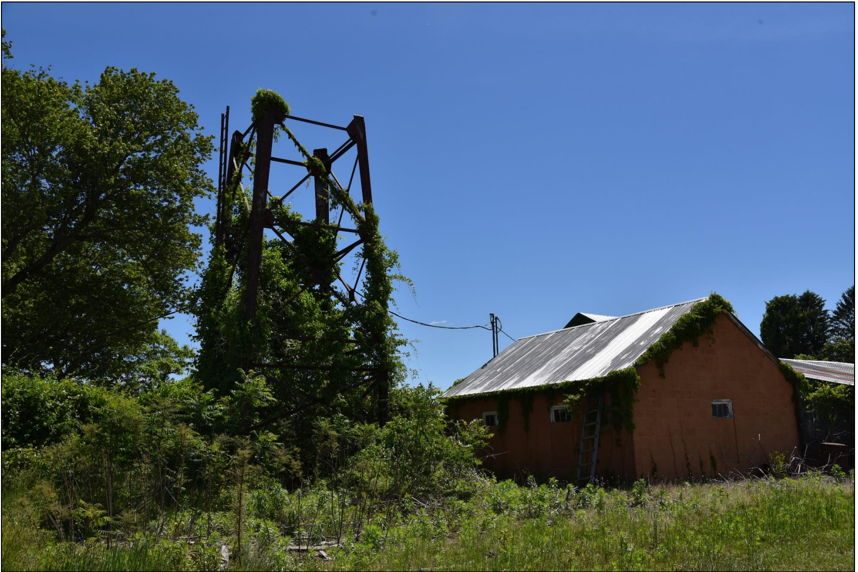
Photo 77: Original water tower, view southeast.
