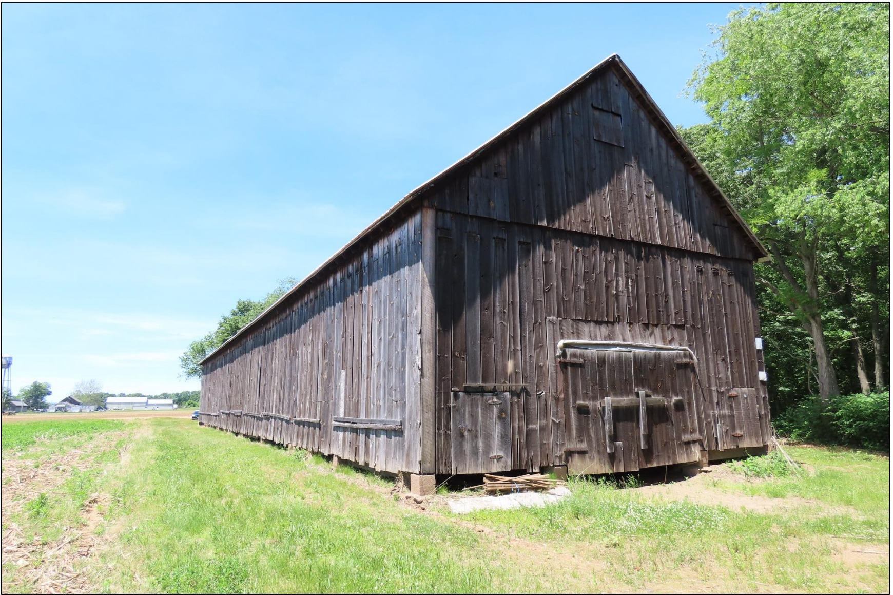
Photo 55: Shed 31, view east.
