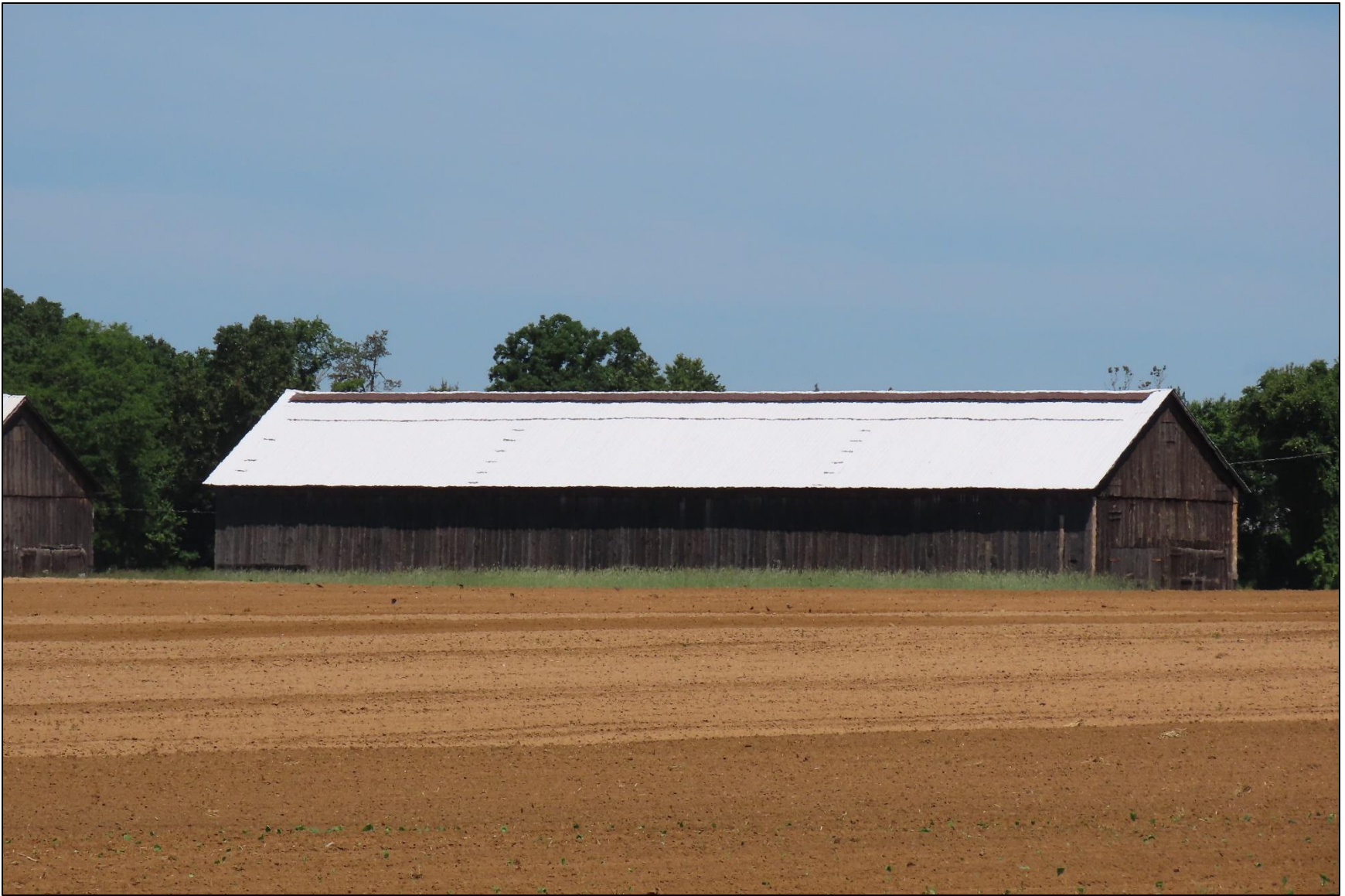
Photo 45: Shed 3, view north.
