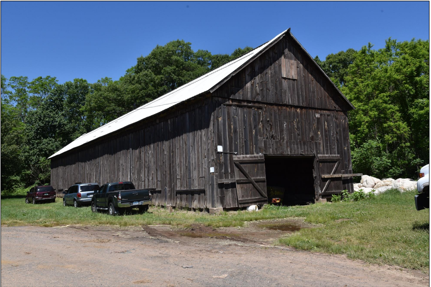
Photo 52: Shed 21, view northwest.
