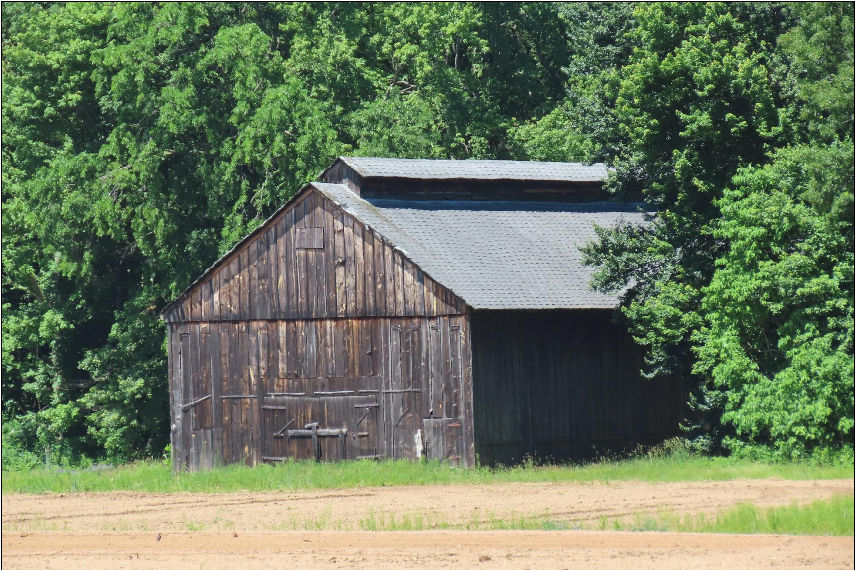
Photo 22: Shed 13, view southwest from Windsorville Road.
