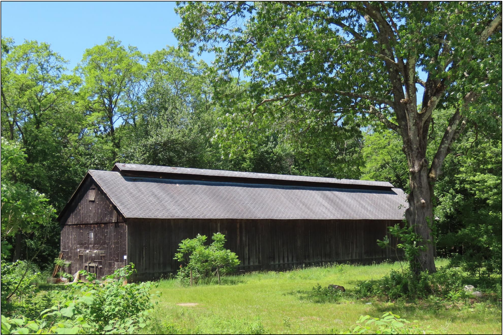
Photo 30: Shed 18, view southwest.
