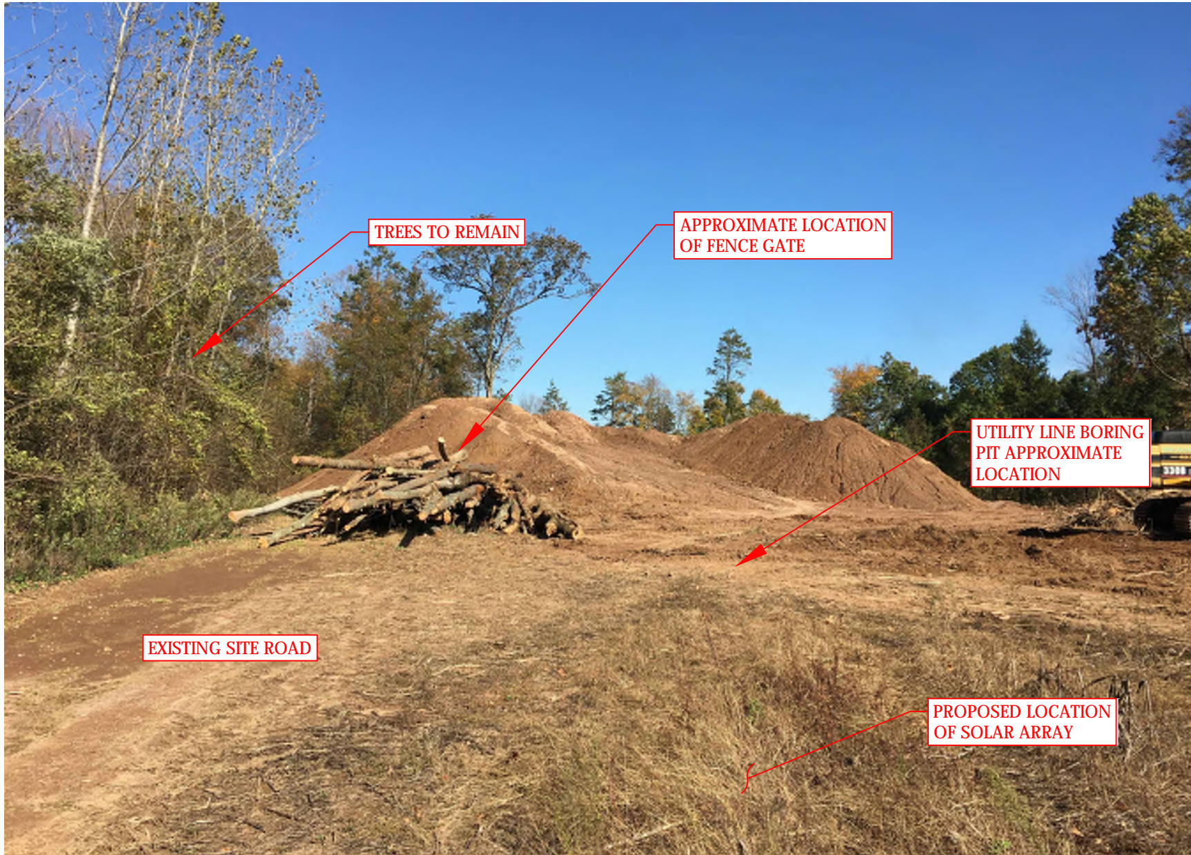
Photo 19 Boring Pit and Utility Line
