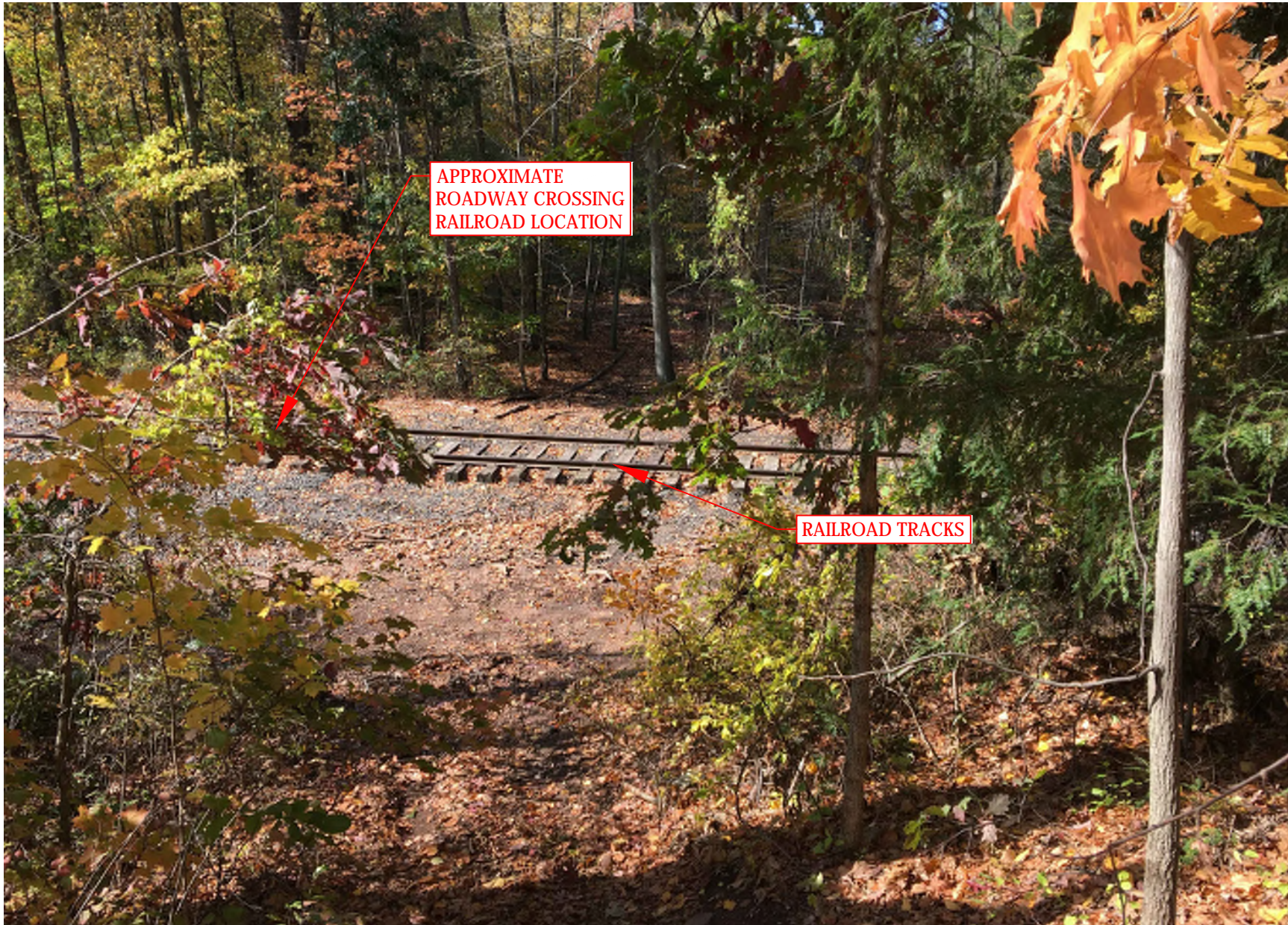
Photo 18 Utility Line Boring Under Railroad Tracks
