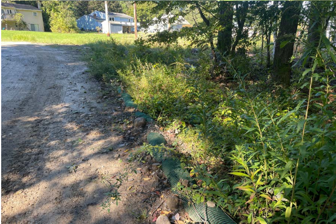
Photo 3: View of perimeter erosion controls along access road.
