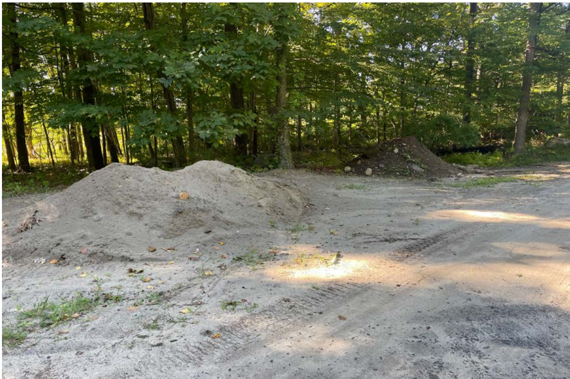
Photo 4: View of material stockpile areas.
