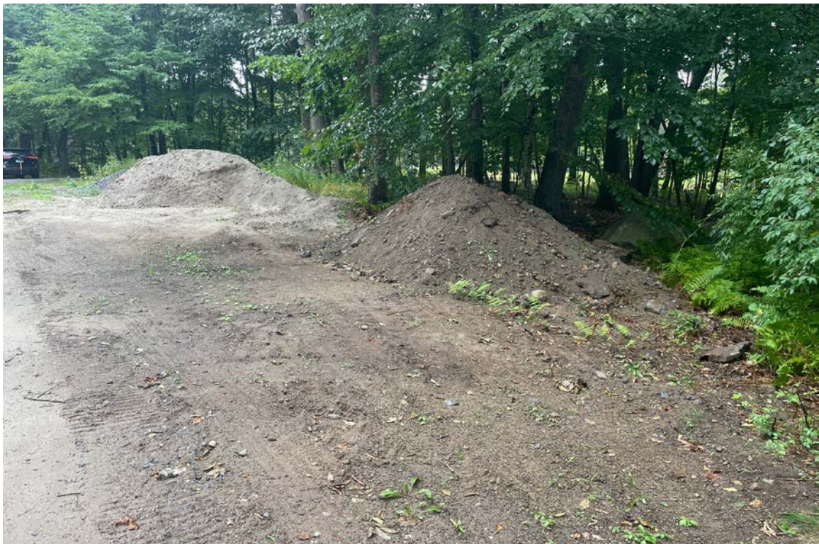
Photo 4: View of material stockpile areas.
