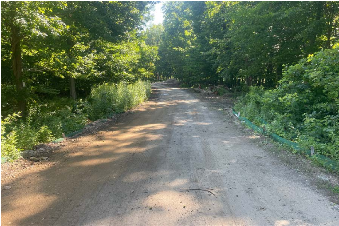
Photo 1: View of access entrance off Phillane Drive, note completed trenchwork.
