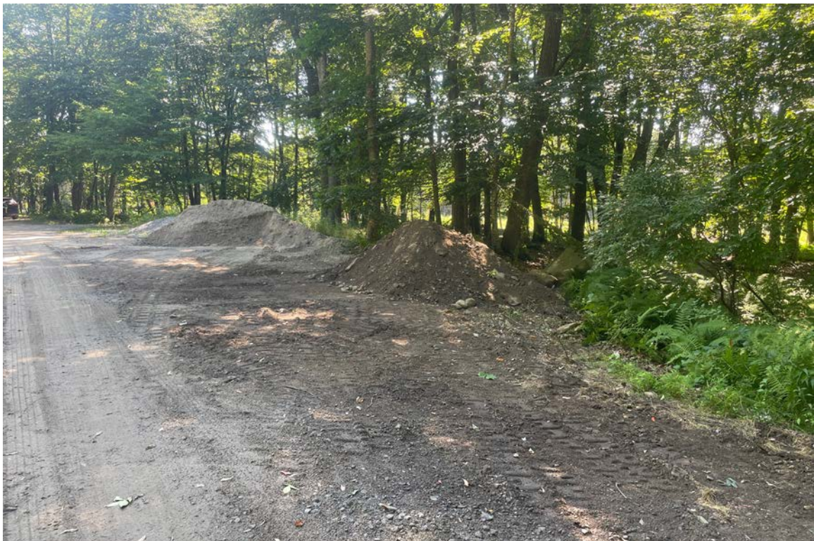
Photo 4: View of material stockpile area.
