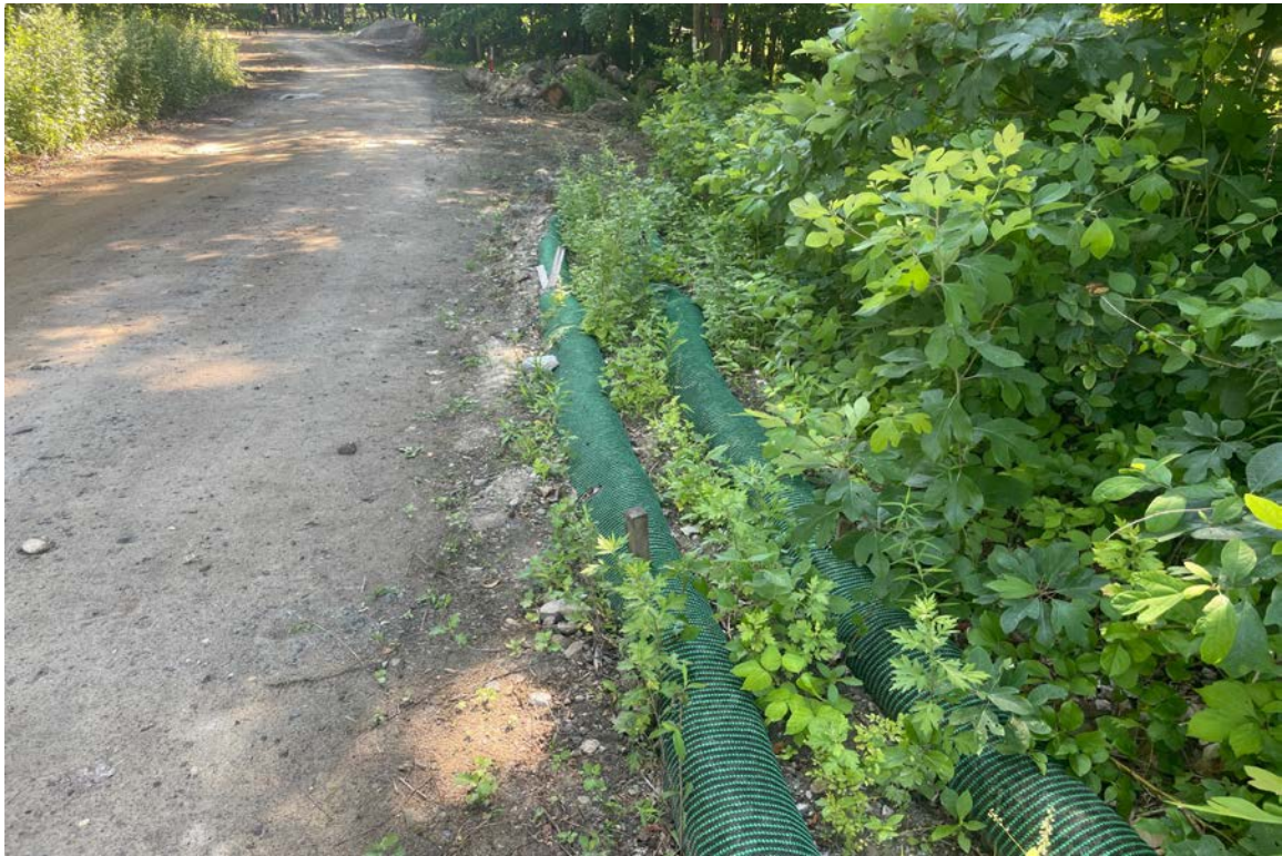
Photo 3: View of perimeter controls along roadway.
