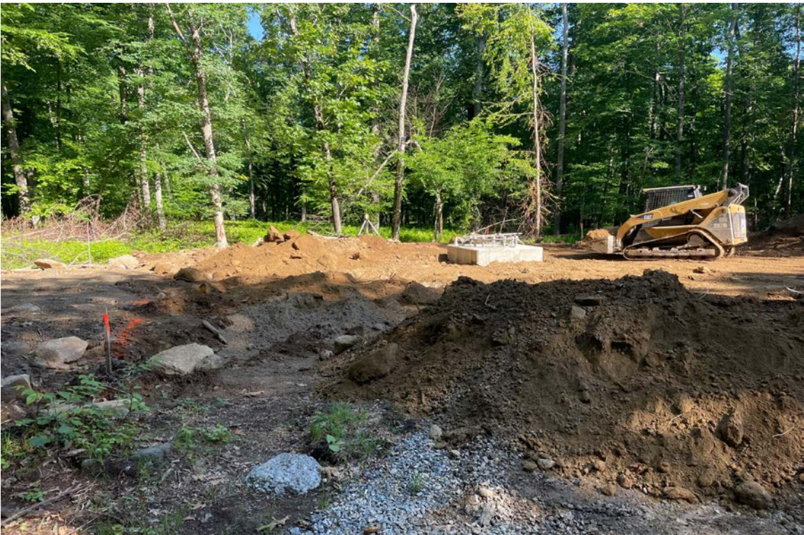
Photo 2: View of compound area grading work.
