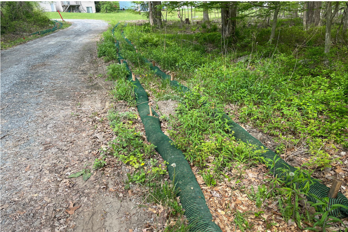
Photo 4: View of perimeter controls installed at wetland crossing.
