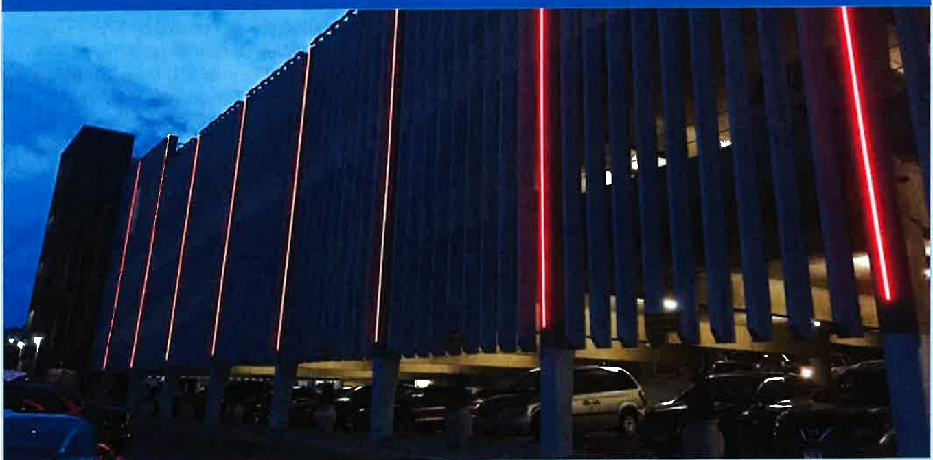
Improvements at the Yankee Doodle garage included exterior and interior LED lighting, and improved security features.
