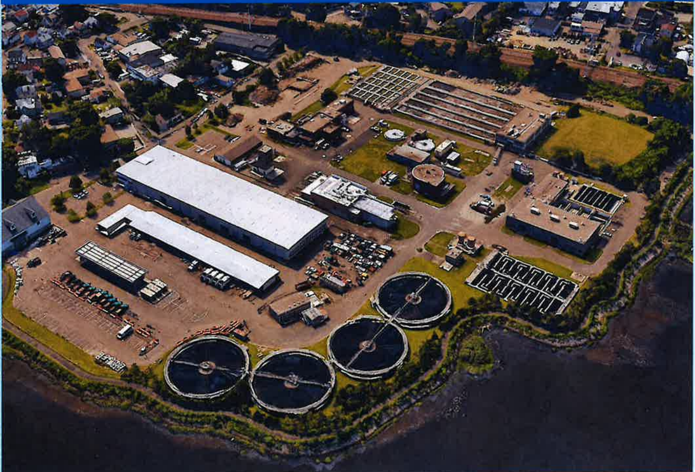
The Wastewater Treatment Plant at Liberty Point
