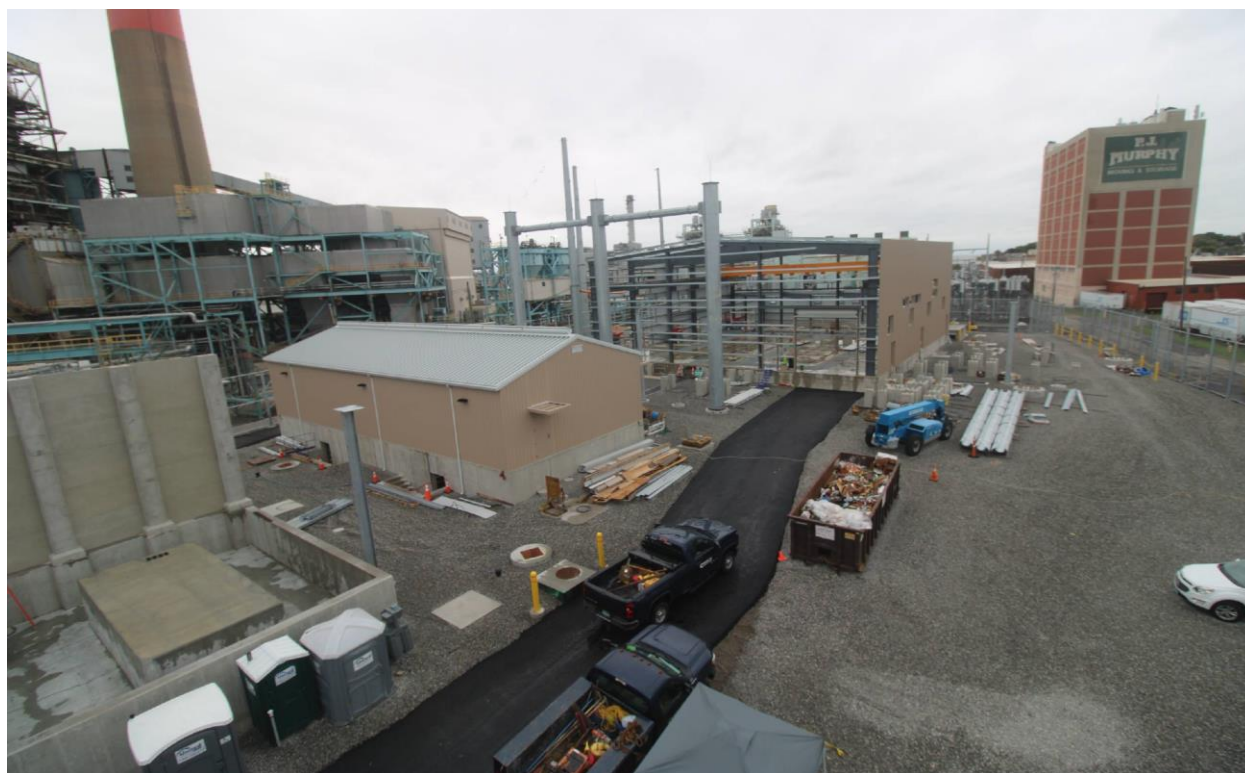
Photo 1: Broadview of project site with GIS/Control Building being erected.
