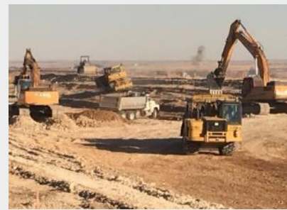
White Alpha II: reservoir construction
