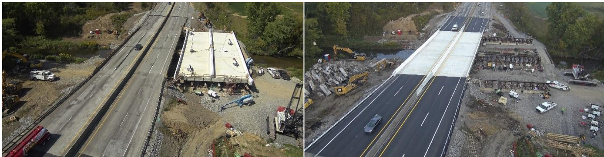
Figure 3 - Accelerated Bridge Construction Technology
