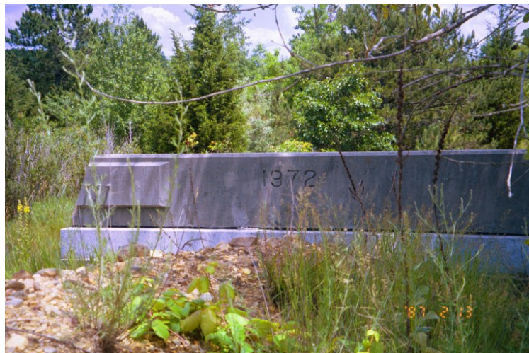
ROUTE 11 TERMINATED AT THE ROUTE 82 OVERPASS IN 1972
