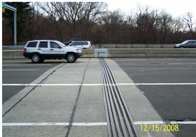
Expansion Joint at Baldwin Bridge, Old Saybrook / Old Lyme
