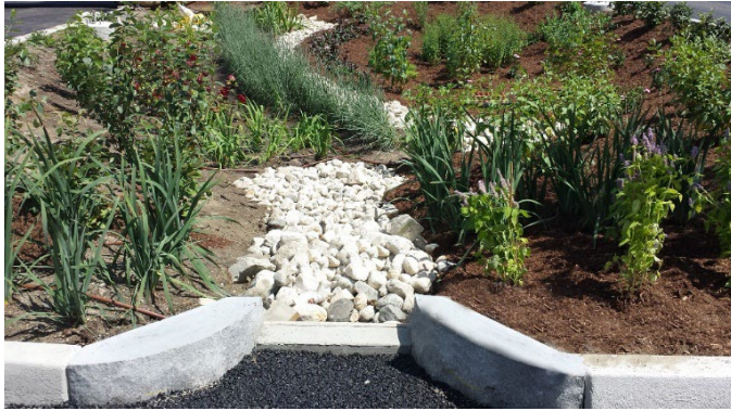
Figure 13-39. Typical Inlet Curb Cut Openings
