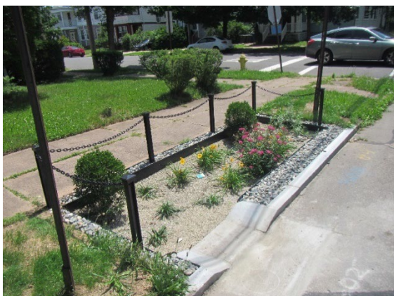
Roadside bioswale in urban residential setting.
