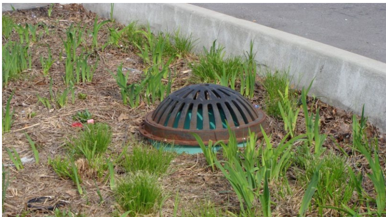
Figure 13-45. Typical Dome Grate Overflow/Outlet Structure
