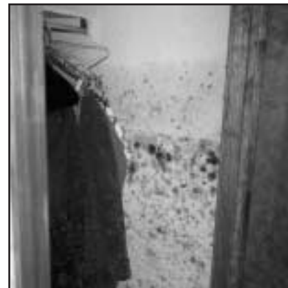
Above, Penicillium , Aspergillus and Stachybotrys on closet wall.
