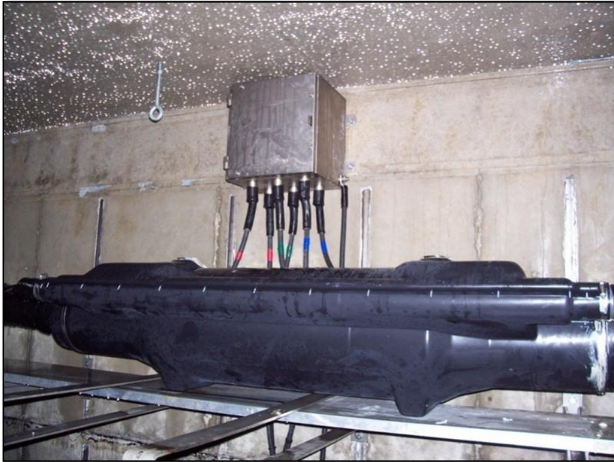
Figure D-6. Typical 115-kV Splice Assembly
