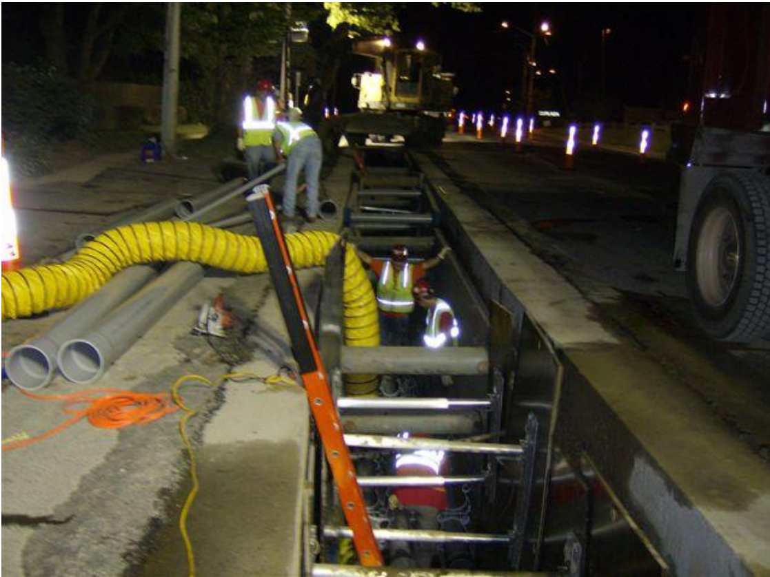
Figure D-4. Typical Duct Bank Trench
