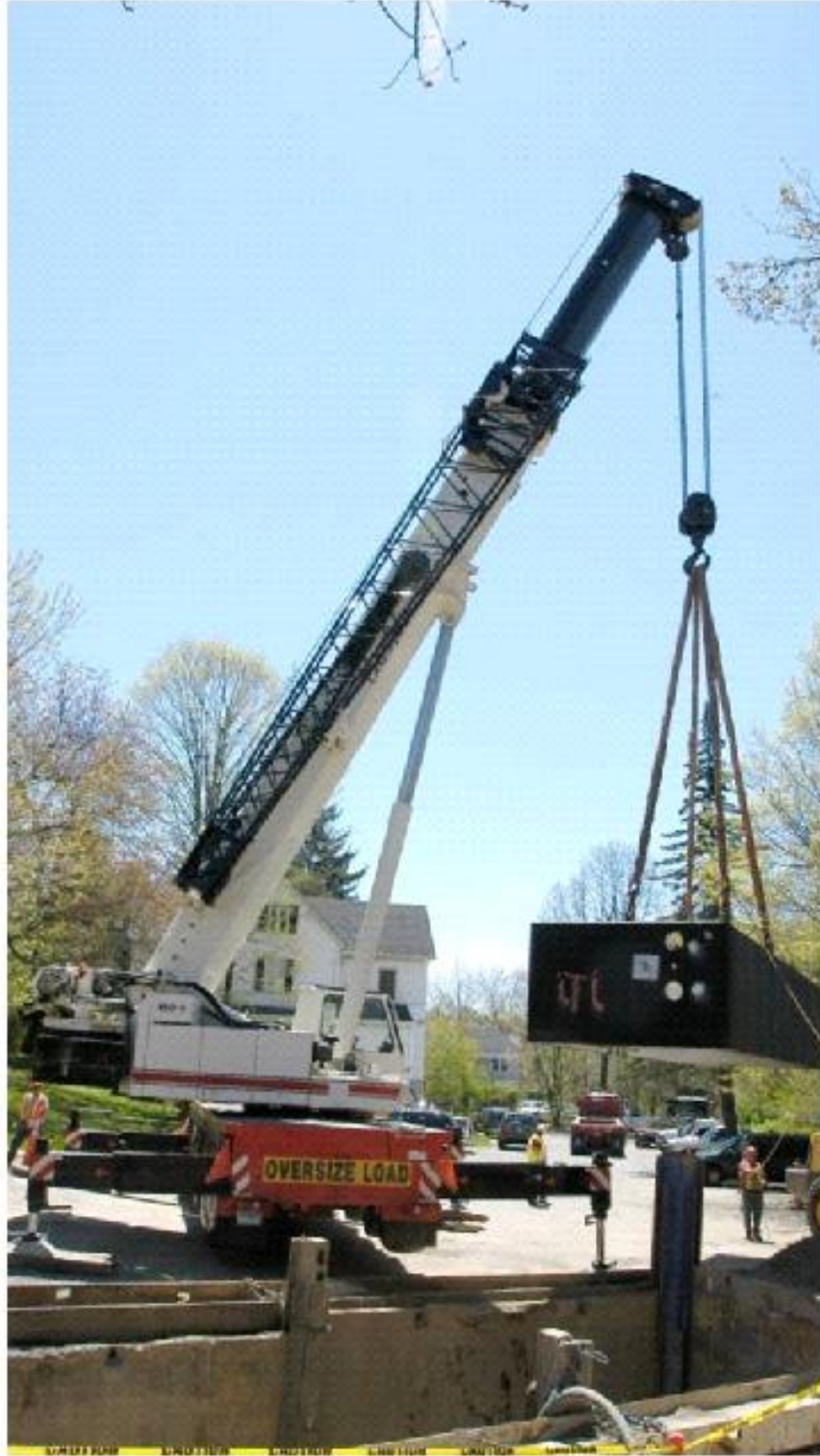
Figure D-3. Typical Splice Vault Installation
