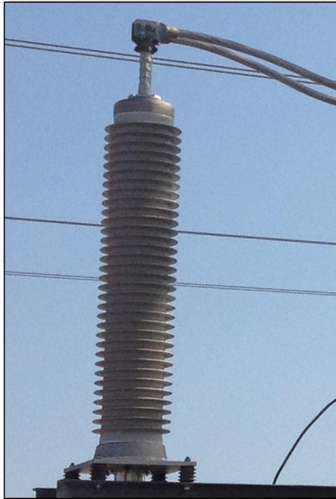
Figure D-7. Typical Cable Termination
