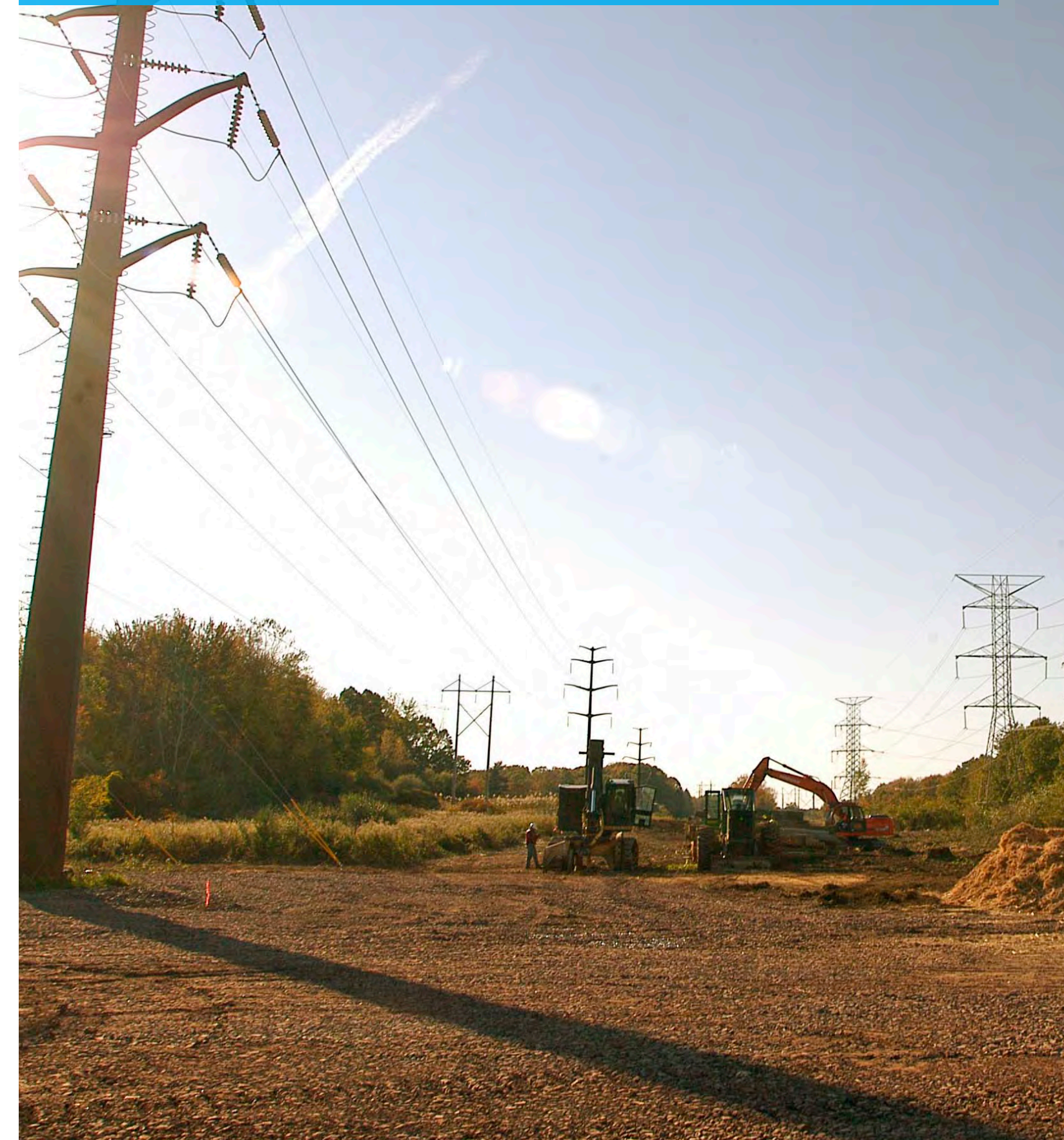
2. Work Area Prep
