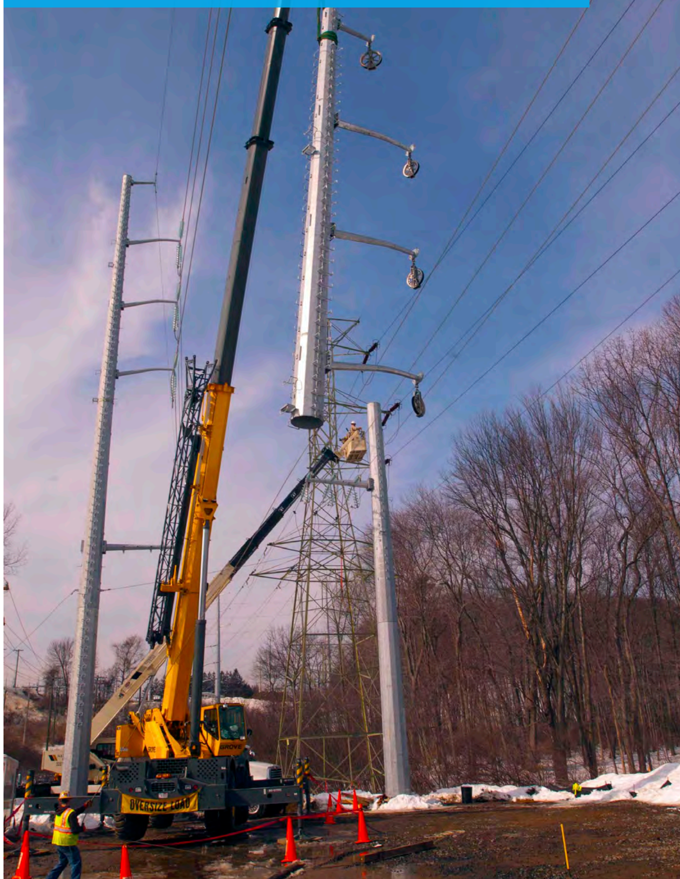
4. New Structure Installation
