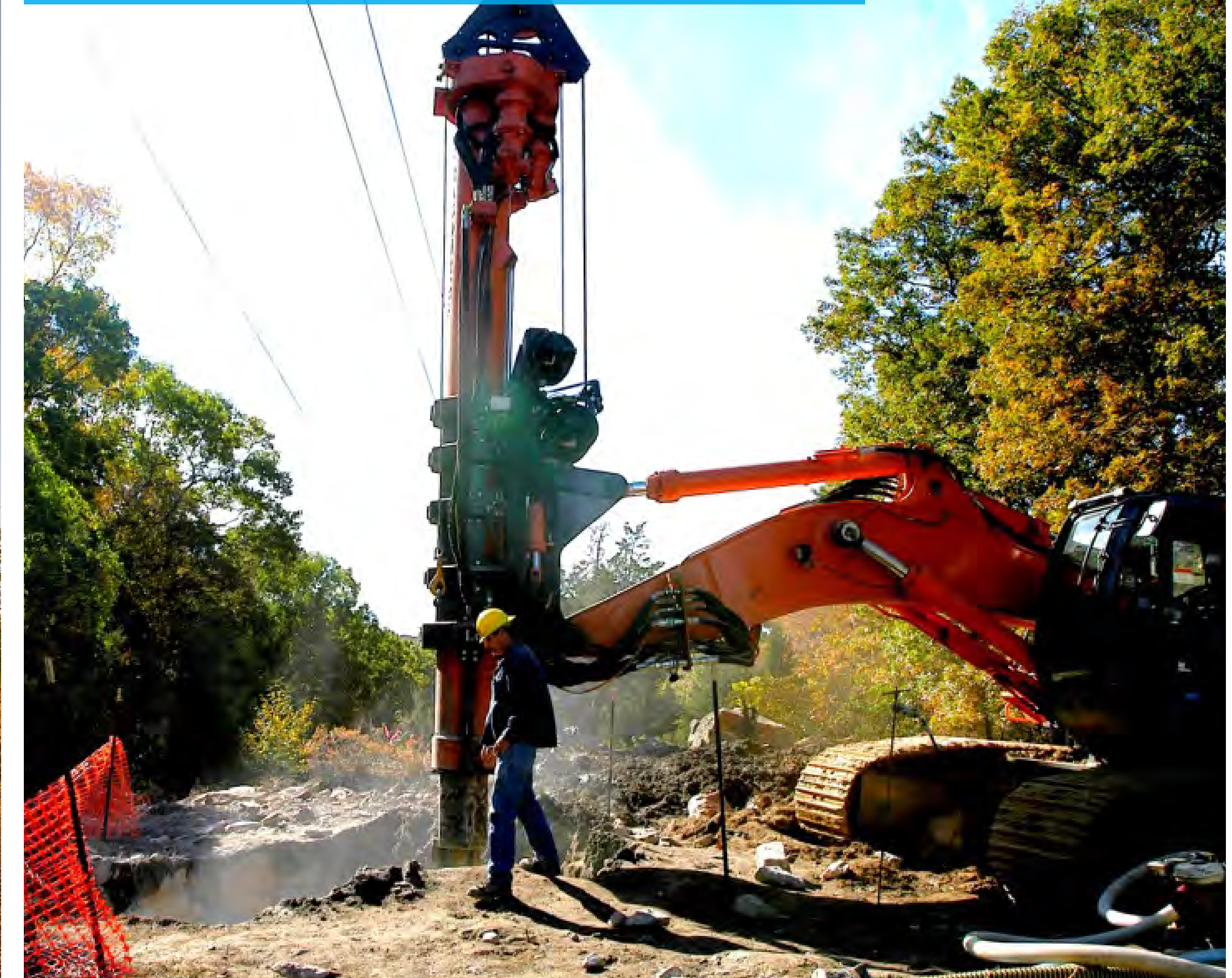
3. Structure Foundation Installation
