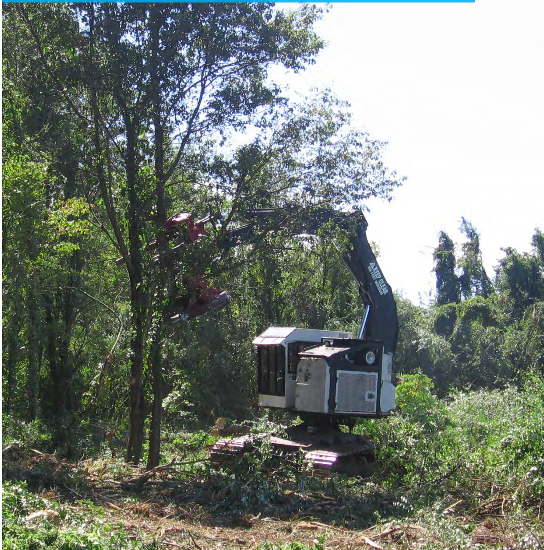
1. Right Of Way Clearing
