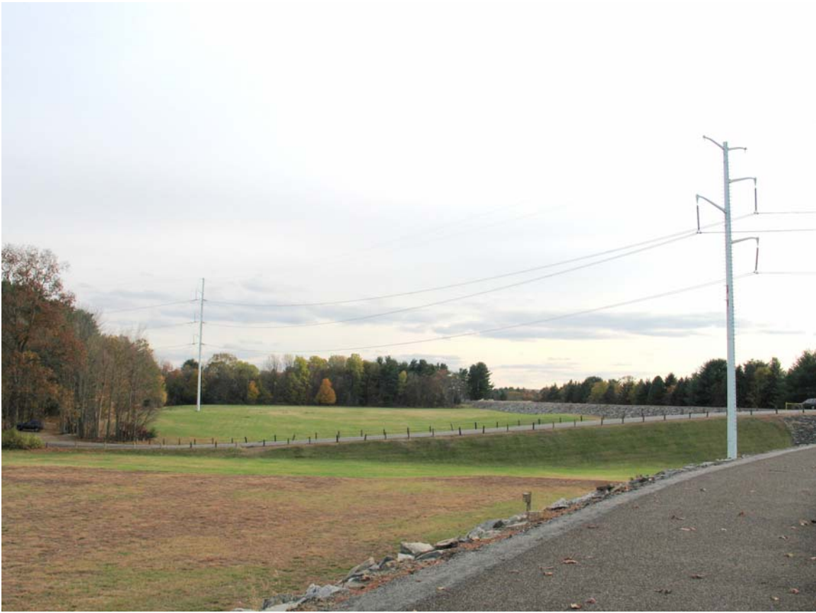
Photograph 6. VIEW SOUTHEAST FROM MANSFIELD HOLLOW DAM 430 FEET TO EXISTING STRUCTURE 9081 (RIGHT) AND 1000 FEET TO EXISTING STRUCTURE 9082 (LEFT)
