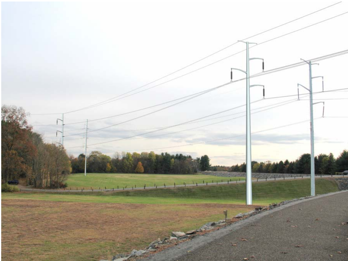
Photograph 7. VIEW SOUTHEAST FROM MANSFIELD HOLLOW DAM WITH EXISTING AND SIMULATED STRUCTURES
