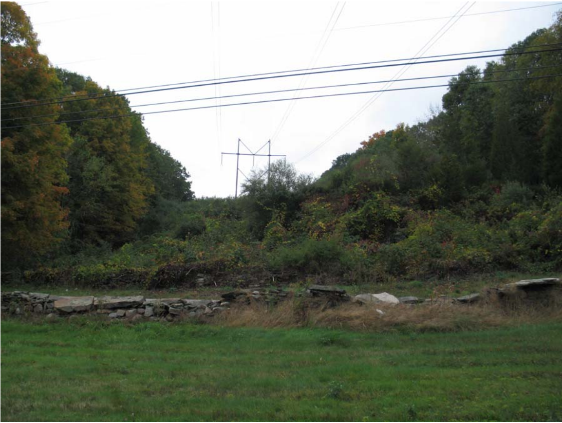
Photograph 8. VIEW SOUTHWEST FROM STATE ROUTE 169 400 FEET TO EXISTING STRUCTURE 9198
