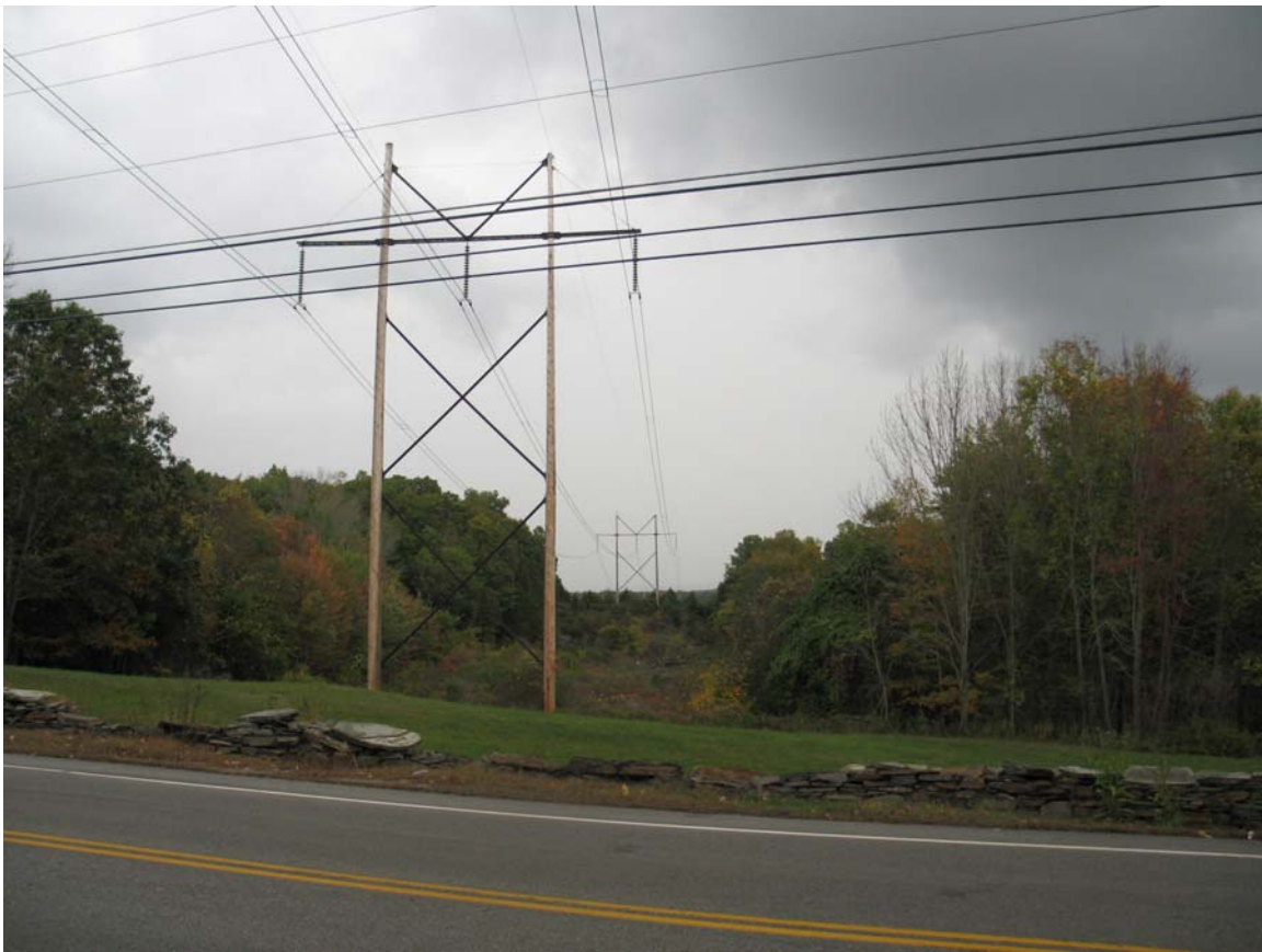
Photograph 10. VIEW NORTHEAST FROM STATE ROUTE 169 130 FEET TO EXISTING STRUCTURE 9199
