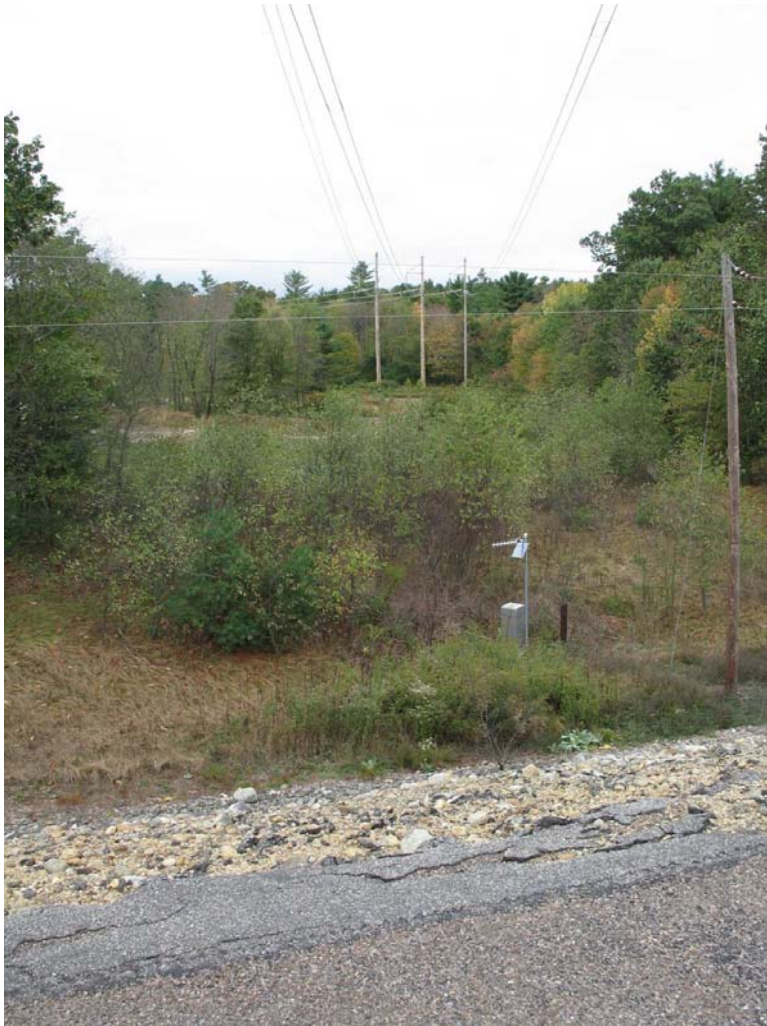
Photograph 4. VIEW NORTHWEST FROM MANSFIELD HOLLOW DAM DAM 630 FEET TO EXISTING STRUCTURE 9080
