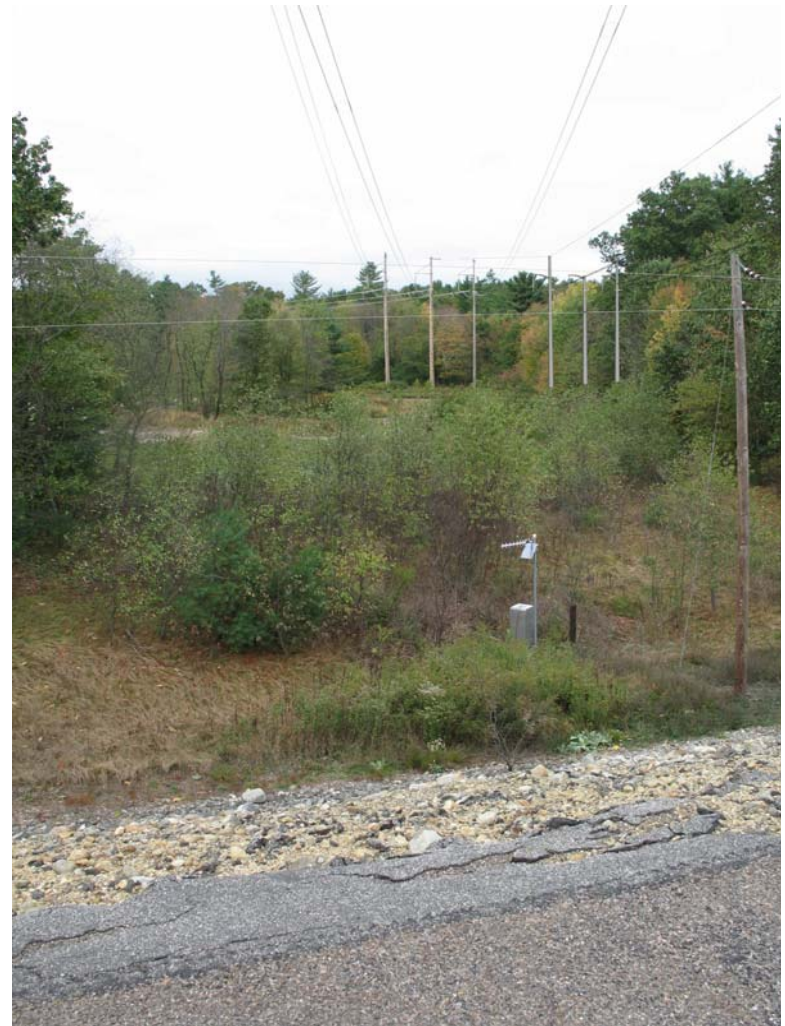
Photograph 5. VIEW NORTHWEST FROM MANSFIELD HOLLOW DAM WITH EXISTING AND SIMULATED STRUCTURES
