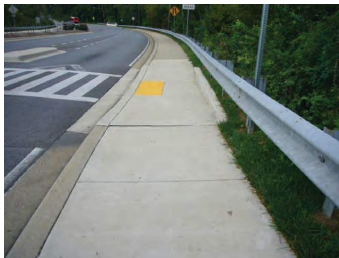
Figure 4-16. Parallel curb ramp.
