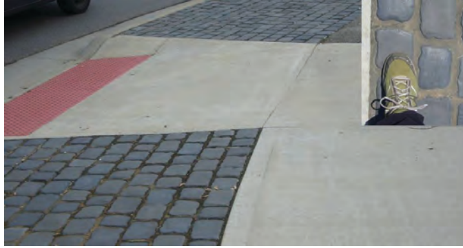
Figure 4-10. Example of surface material that was not recognized as a non-walking surface by blind participants.
