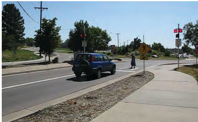
Figure 4-22. Pedestrian hybrid beacon at roundabout in Golden, Colorado.
