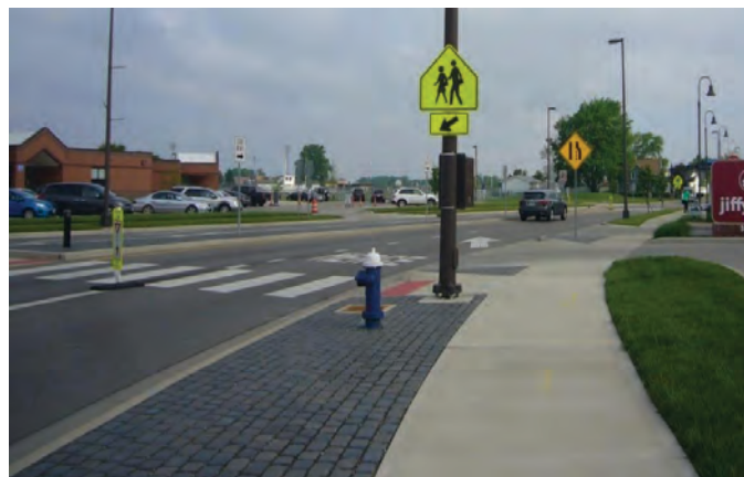
Figure 3-7. Sidewalk separation at a roundabout not detectable under foot or by the use of a long cane.
