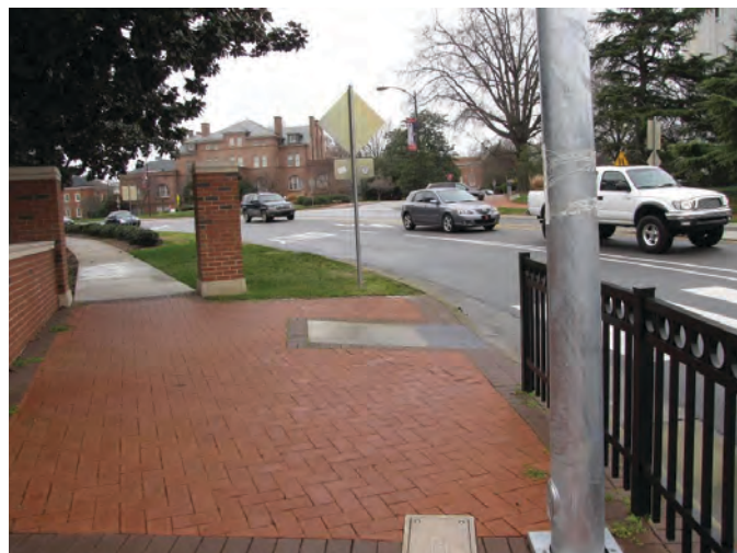
Figure 4-11. Fencing and grass strip at a roundabout corner.
