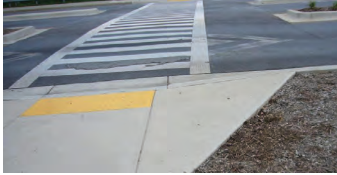
Figure 4-17. Ladder crosswalk marking.
