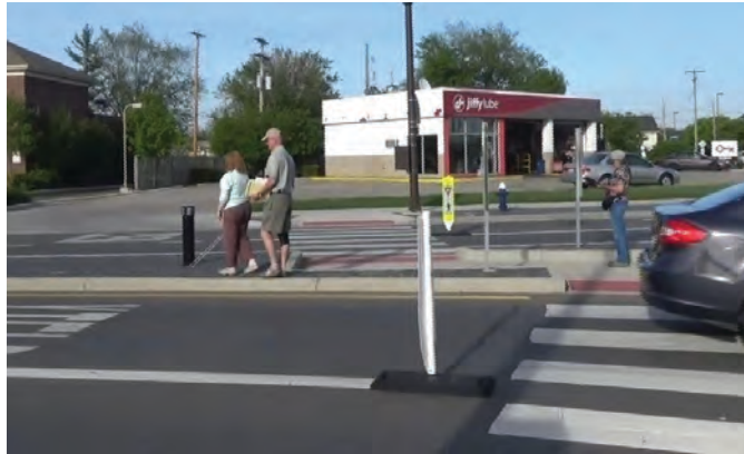
Figure 3-3. Pedestrian walking on a splitter island rather than in a cut-through crosswalk.
