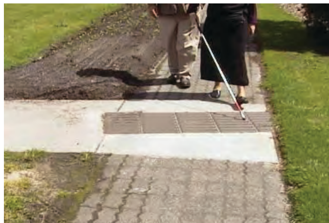
Figure 4-13. Australian bar tile surface.
