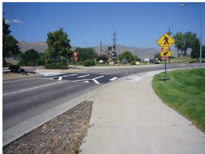
Figure 4-29. Raised crosswalk at a two-lane roundabout.
