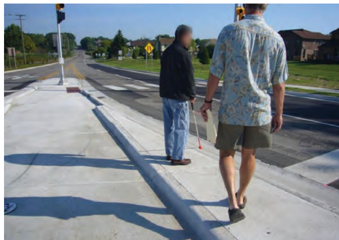
Figure 4-18. All-paved roundabout splitter island.
