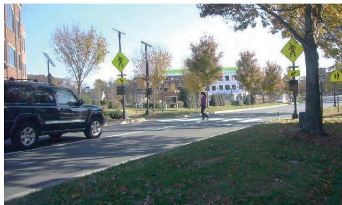
Figure 5-13. RRFB at a two-lane roundabout.
