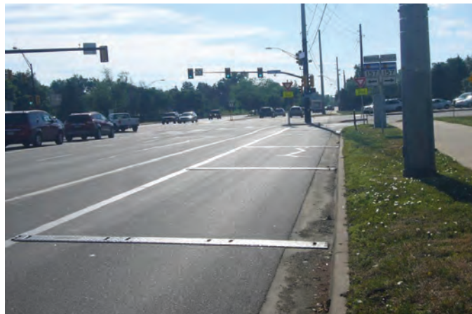
Figure 5-17. Sound strips installed at a CTL.
