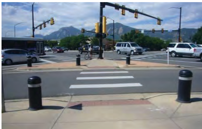
Figure 5-14. Detectable warning surface installed at a CTL crossing.
