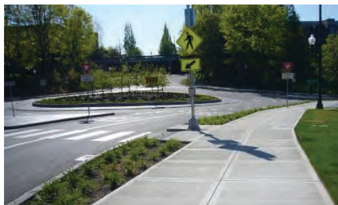
Figure 4-9. Landscaping that discourages crossing to the central island and provides an edge that blind pedestrians can follow (i.e., trail) with the long cane to locate a curb ramp.
