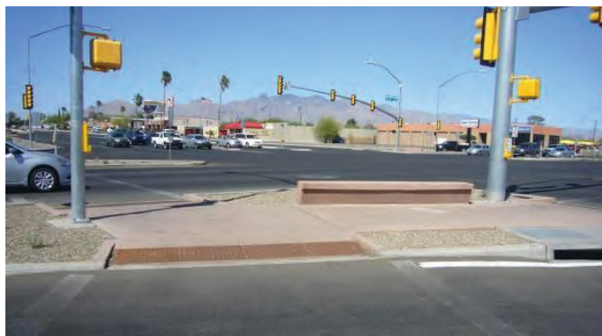
Figure 5-5. Island with ramps to paved walkways and gravel outside the pedestrian path area.
