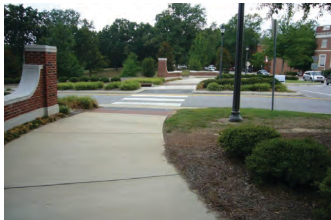
Figure 4-8. Sidewalk curving away from the corner to guide pedestrians directly to the crosswalks.
