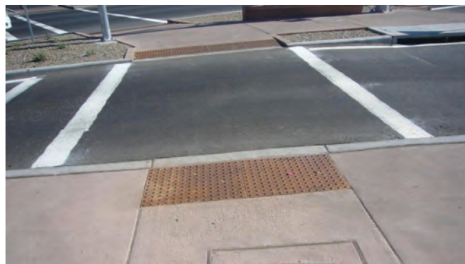
Figure 5-8. Example of a properly placed and aligned crosswalk at a CTL.
