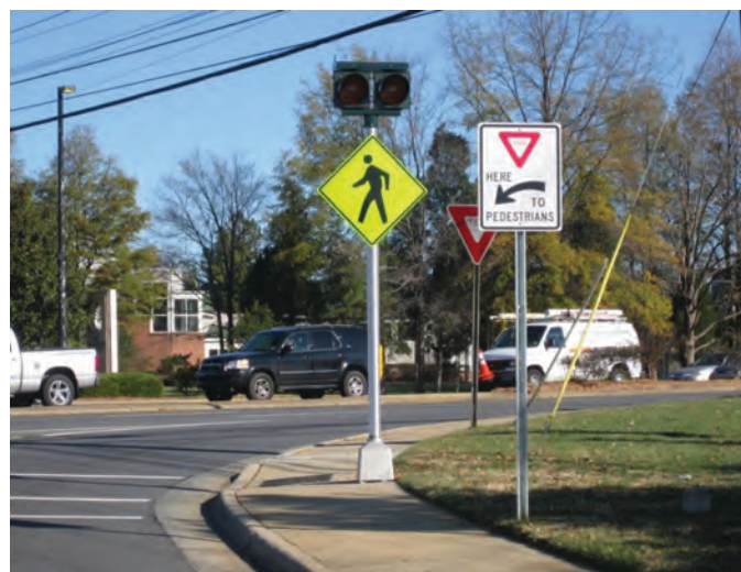
Figure B-6. Flashing beacon at CTL.
