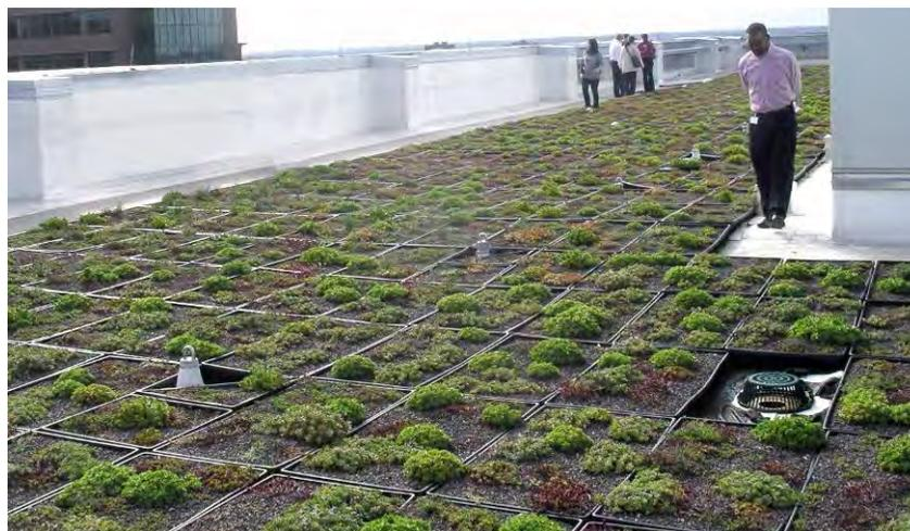
Figure 2.2.3. Modular Green Roof System Installation
