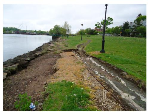
Figure 2.1.1. Shoreline Erosions and Erosion on Walkways at Quinnipiac River Park
