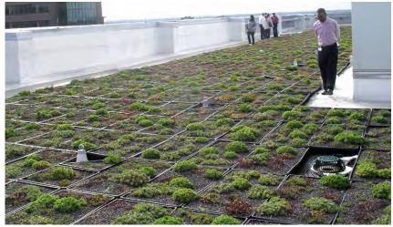
Figure 2.2.3. Modular Green Roof System Installation
