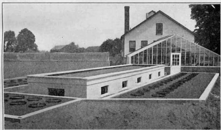
FIGURE 9. Exterior view of the lysimeters.
