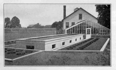
FIGURE 9. Exterior view of the lysimeters.
