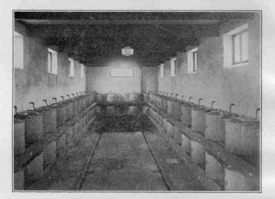
FIGURE 10. Interior of lysimeter pit.
